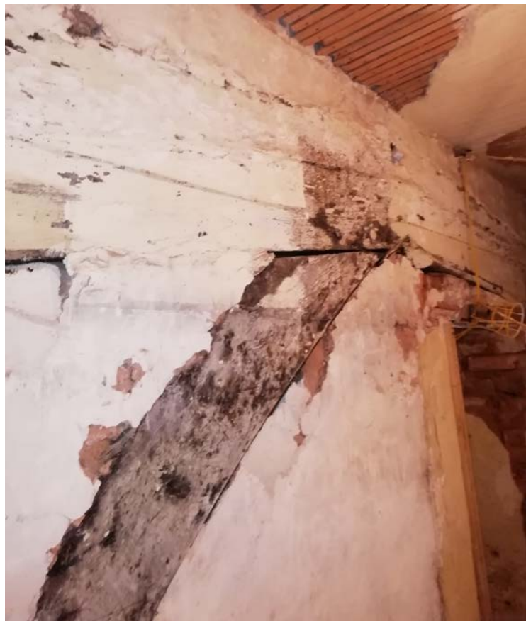
Figure 3: The west arch-brace and tiebeam to the north remnant medieval truss, looking north (photograph Martin Bridge)
