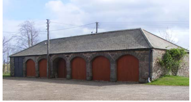
Here, this single-storey, seven-bay cart shed stands alone on the yard perimeter. The hipped roof is a design common to yard buildings of the 18th and 19th centuries. Photo © Jen Deadman]
