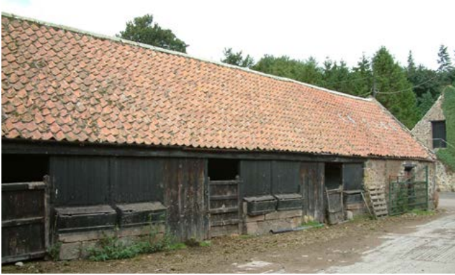
Late 19th-century cattle units often consist of hemmels and yards with shelter sheds and root houses. The root houses here have outward-facing double doors, through which fodder could be loaded into them, and the rear walls contain a doorway to each yard; each pair of yards, now covered, was served by one root house. Photo © Jen Deadman
