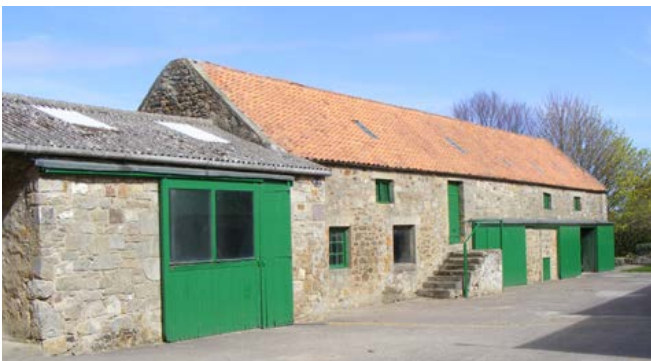
This late 18th- or early 19th-century combination barn combines various functions in one build, some of which are difficult to determine from the exterior alone. It comprises stables to the left, with external steps to the right of its blocked door to the window. At the far end are cart sheds (20th-century doors) with a granary above. Photo © Jen Deadman
