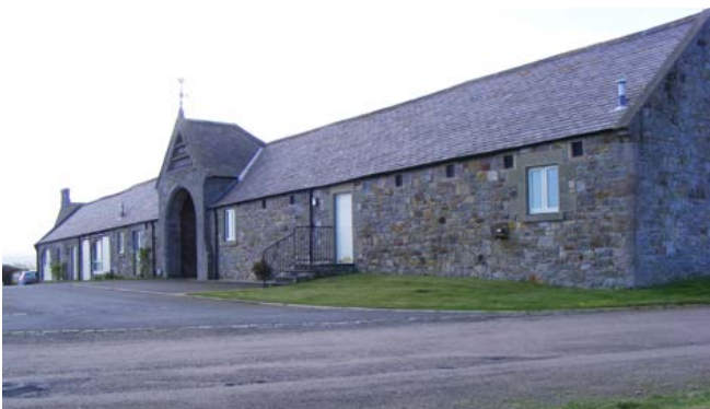
This early to mid-19th-century courtyard farmstead exemplifies many key features of this area. The house faces away from the regular courtyard arrangement of farm buildings, and to the left is the distinctive conical roof of a horse engine house (locally termed a horse gin or gin gang) attached to a threshing barn and straw barn. Photo © Jen Deadman
