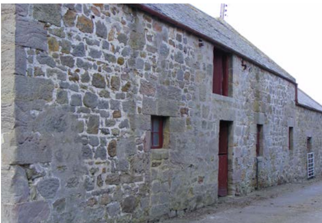
Stables are frequently incorporated in a yard range and are generally lofted over. The rubble walling here suggests a date of around 1800 or earlier. Photo © Jen Deadman
