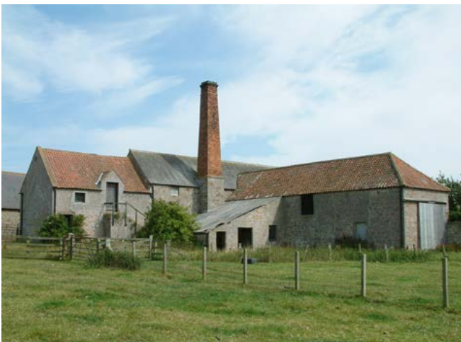
Engine houses. This group at Ford has the chimney stack which served the steam engine and its boiler, housed in the lean-to at the angle between the threshing barn and the straw barn. The steps to the left provide access to a granary. Photo © Jen Deadman
