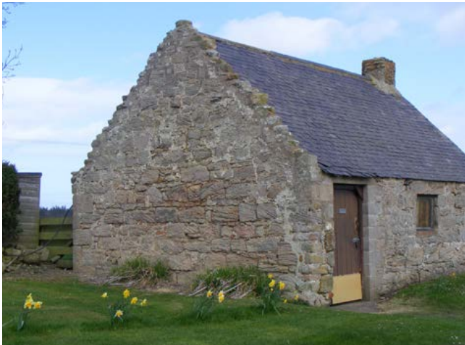
Smithies. This smithy stands by the roadside, adjacent to estate cottages at Felkington, which by around 1800 had shrunk from a village into a farm hamlet comprising one large farmstead. It is characteristically single-storey and has one entrance flanked by a small window. It has a stack set against the gable wall. The crow-stepped finish to the near gable is in the Scottish tradition. Photo © Jen Deadman
