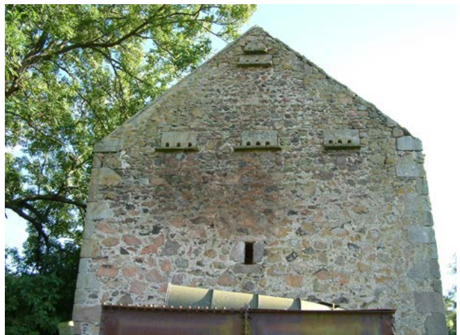
Pigeon lofts are frequently seen in the gable ends of houses and barns. At Akeld bastle, the pigeon loft, sited on the south elevation, comprises five separate stone ledges and stone backing pieces, four pierced with three pigeon holes and the fifth, at the apex, by two holes. Photo © Jen Deadman
