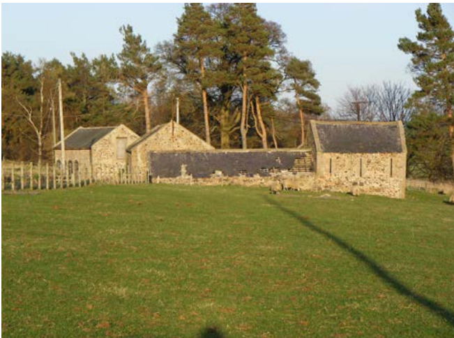
Cattle housing. On this smaller, late 18th- or early 19th-century steading, the single-storey byre range adjoins a hay barn on one side of a yard. Photo © Jen Deadman
