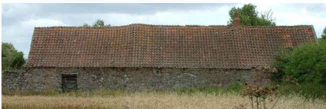
This rare, surviving 18th-century or earlier linear farmstead, built of random rubble and river boulders, is set in fields of piecemeal enclosure to the north-west of Wooler. To the north are larger, more regular fields indicative of late 18th- and 19th-century enclosure. The house body is one cell and single storey with external access directly into the room. There is no evidence for a loft. The byre has stalls for four beasts, with opposed doors east and west towards the northern end of the byre. The east door opens onto the front yard; the west door (blocked), opens directly onto the fields. The lintel over this door appears to be a re-used cruck blade. The room at the far end has opposed doors at its northern end, and a forking hole in the cross wall linking it to the byre would suggest a loft over a byre or a part-lofted threshing barn. Photos © Jen Deadman
