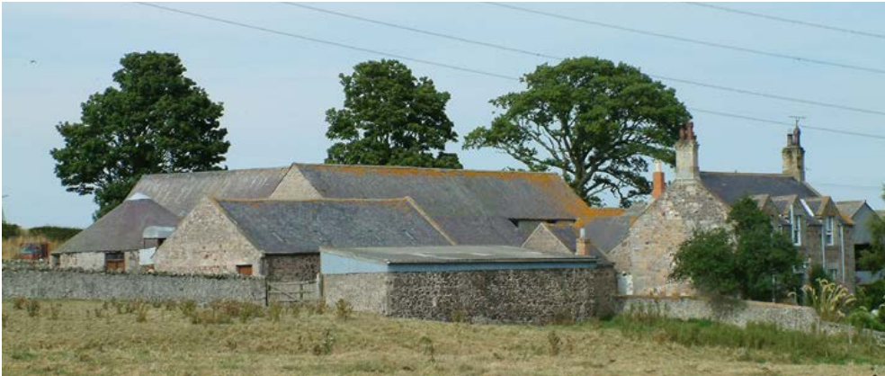
At West Flodden, the horse gin is adjacent to the threshing barn which adjoins the large combination barn. The intricate roof structure is still intact. Photos © Jen Deadman
