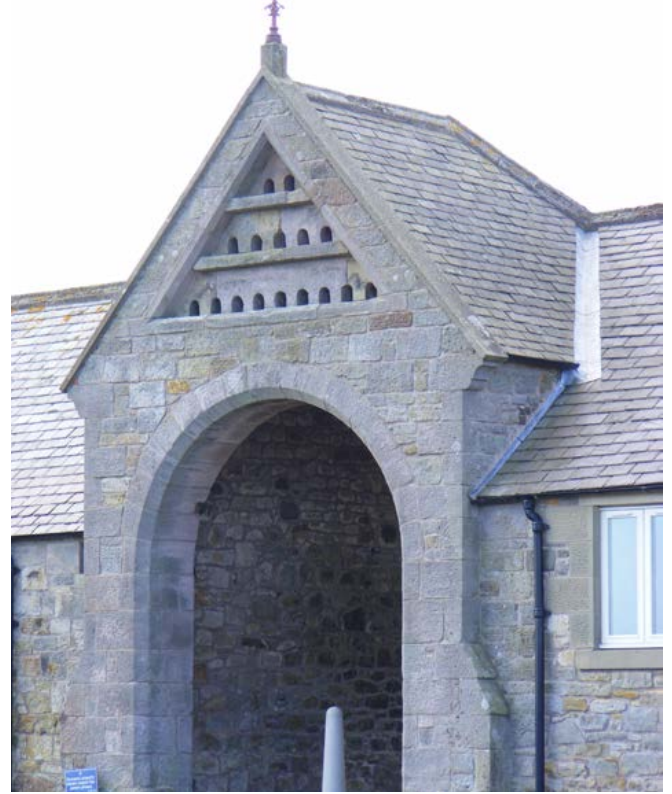
On the large estates, the pigeon loft is frequently sited at the top of a tower which commands a central position above the main entry to the farmstead. At New Bewick, the tower rises above the adjacent ranges, the ground and first floor acting as reception and offices for the farm. Photo © Jen Deadman
