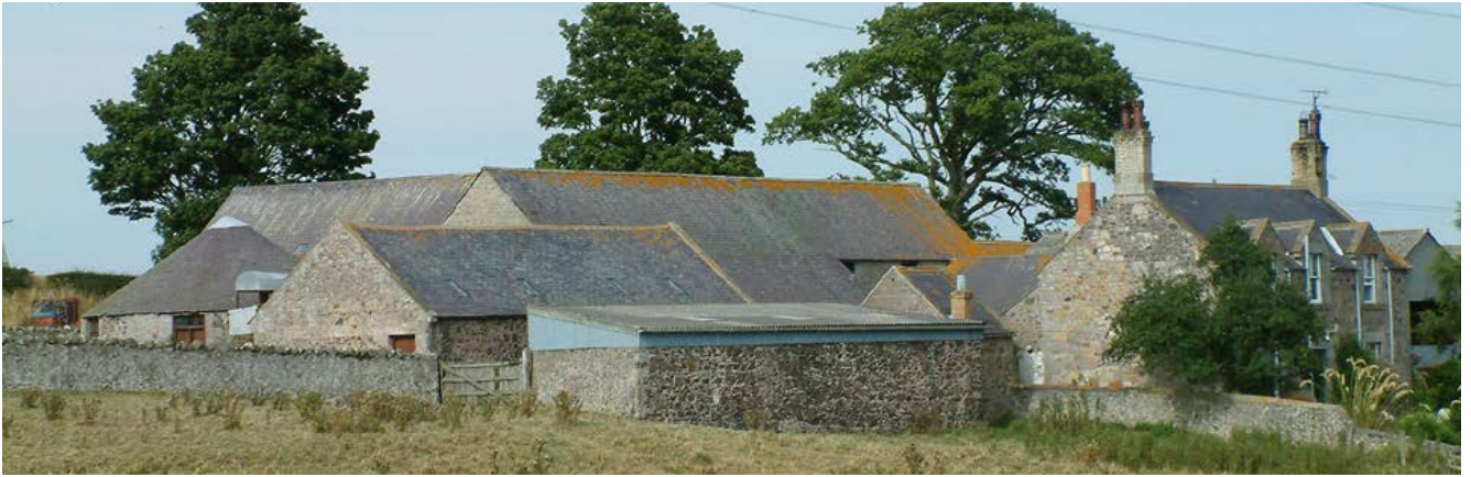
This early to mid-19th-century courtyard farmstead exemplifies many key features of this area. The house faces away from the regular courtyard arrangement of farm buildings, and to the left is the distinctive conical roof of a horse engine house (locally termed a horse gin or gin gang) attached to a threshing barn and straw barn. Photo © Jen Deadman
