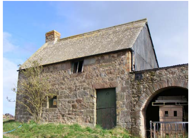
This mid-19th-century smithy adjoins an eight-bay cart shed on the hillside above the yard. It is two-storeyed with a lofted area, probably for a farm worker, above the working smithy. The forge and bellows are still in situ as is a quantity of working tools. Photo © Jen Deadman
