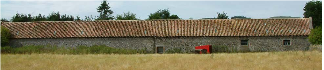
Here, the full length of a rear shelter shed from which all the yards branch off is viewed from across the fields, the long, low range a characteristic feature of this particular farming landscape. Note the pantile roof. By the end of the 19th century, slates were usually adopted. Photo © Jen Deadman
