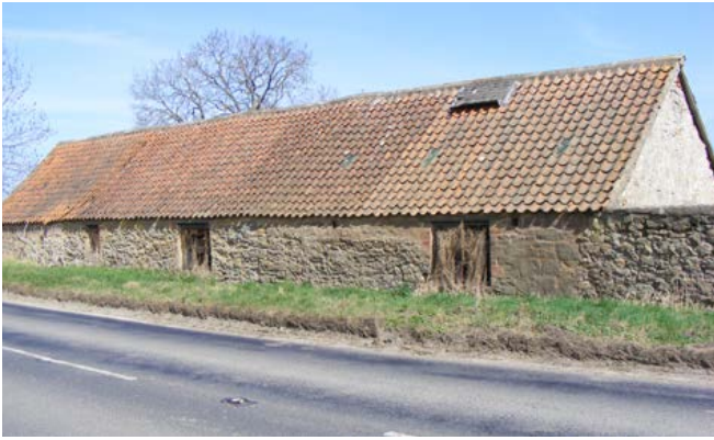
Combination barns. This linear range, possibly of 18th-century date, is a rare, surviving example of a pre-improvement era farm building. It comprises a small combination barn with threshing floor and animal housing adjoining at the far end. The barn has a small entry opening onto a yard area, raised into the roof for extra height. An opposed door opens onto the roadside. Hay was stored to the left of the threshing floor, with a byre to the right. Photo © Jen Deadman
