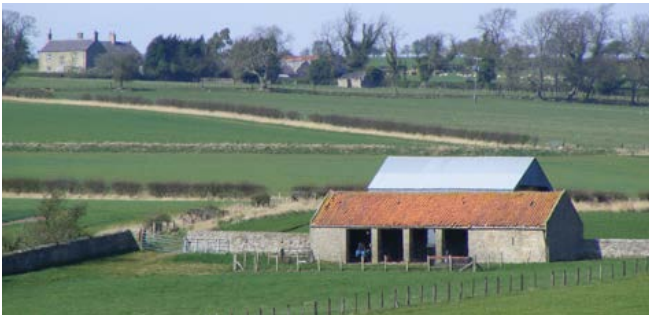
Cart sheds. At New Bewick, this mid-19th-century, open-fronted, four-bay cart shed, with a roof supported by cast iron columns, lies in a stepped range of single storey ancillary buildings. To the right are cottages and a trap house with a further cart shed to the left. Photo © Jen Deadman
