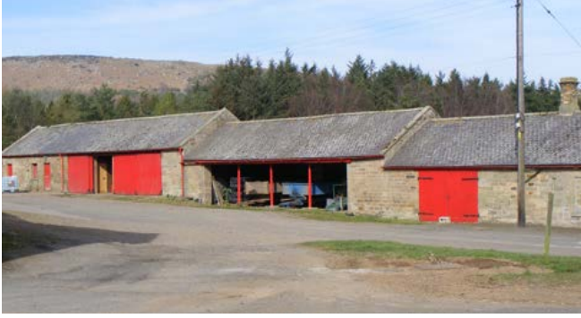
Cart sheds. At New Bewick, this mid-19th-century, open-fronted, four-bay cart shed, with a roof supported by cast iron columns, lies in a stepped range of single storey ancillary buildings. To the right are cottages and a trap house with a further cart shed to the left. Photo © Jen Deadman
