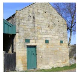
Mid- to late 19th-century combination barn, built of well coursed and squared masonry, as is the pigsty. Note the fine coping stones on the sty wall and the quality of the dressings around openings and feeding chute. Photo © Jen Deadman
