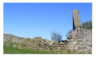
Adjoining to the left is an older structure, now ruinous but with the gable end still intact. Walls of field stone stand to approximately one metre high. The newer build abuts the older and incorporates the old gable in its fabric. The older building measures approximately 6 by 4.5 metres. Photo © Jen Deadman
