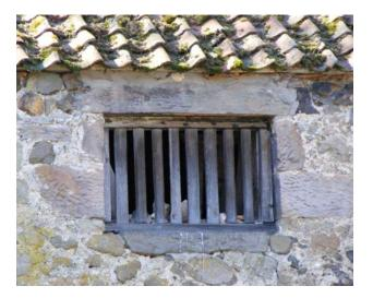
Quoins to corners and openings are generally of long and short sandstone blocks. Here they are left unfinished at the outward edge and marked with a scribed line up to which the render would have abutted. Photo © Jen Deadman
