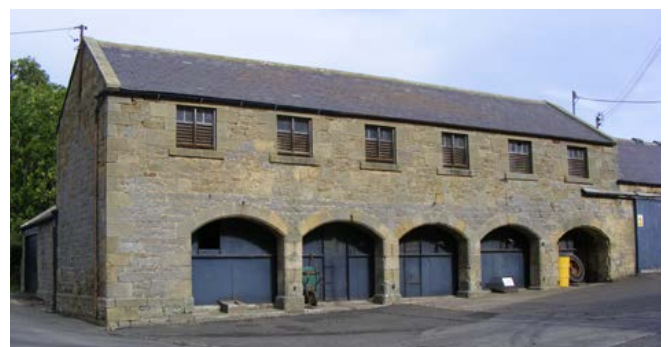
The combination of a large cart shed over granary is a characteristic building type of the Northumberland Coastal Plain, extending north into the Lothians and south into Lincolnshire. Below is a late 19th-century remodelling of an early 19th-century, single-storey range. Photo © Jen Deadman
