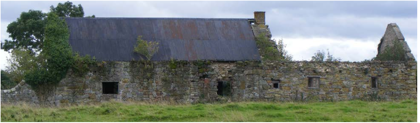
A rare survival of a 17th-century linear farmstead – with a former dwelling and integral cow house/barn built to a longhouse design – can be found in the hamlet of Cheswick, south of Berwick on Tweed (as illustrated on front cover and map on p.10). The single-storey structure stands alone amongst former open fields evidencing strip cultivation and rig cultivation. On the front elevation, adjacent to the stack, is a doorway with a striking four-pointed arched lintel which provided access via a cross passage behind the stack to both the low (animal) end to right and upper (domestic) end to left. Corrugated iron replaces former thatch. A former stone walled enclosure is evident to the side and rear of the animal end. Photo © Jen Deadman
