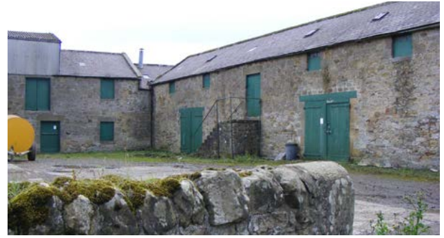
Here, on the outskirts of Rock village, this large arable farm has a granary set over cart sheds linked to a large, multifunctional building housing a corn drier. Photo © Jen Deadman
