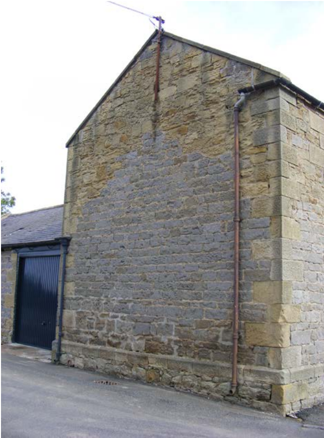
The evidence for raising to two storeys is seen in the contrasting colours of the stonework in the gable end and front elevation. At the gable end the line of the earlier lower roof is visible. Photo © Jen Deadman
