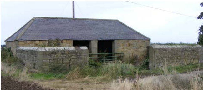
This shelter shed for cattle is located on the roadside outside the estate village of Rock. Also termed 'hemmel', it provides cattle with open access to the small yard set in front. Troughs and mangers are ranged along the roadside elevation. There is pedestrian access to the shelter in the west gable. Photo © Jen Deadman
