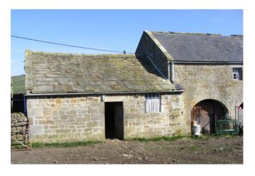
A stable showing a stone slate roof in diminishing courses, with a straight joint to the right, showing that it is an earlier phase of construction than the hemmel, with granary to the right. Photos © Jen Deadman
