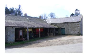
Here, once again, the cart or implement is set outside the yard by the roadside. This roof is supported by simple, cast iron columns. Photo © Jen Deadman
