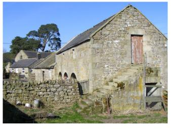
19th-century steading set in the hamlet of East Woodburn in the south-west of the area, showing in the foreground steps to a granary above an open-fronted hemmel for cattle. It has small, part-glazed windows, the lower section being of wooden slats for ventilation. The ridge has raised pieces to aid ventilation. To the left, is a single-storey stable. There is a dog shelter in the recess under the stone steps. Photo © Jen Deadman
