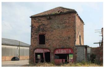
An early 19th-century dovecote on a large farmstead with two-bay cart shed below. The nesting boxes are of brick. A drive shaft and belt in the cart shed would suggest a secondary function for the latter such as a turnip house with motive power sourced from the now derelict adjoining building. Photo © Jen Deadman
