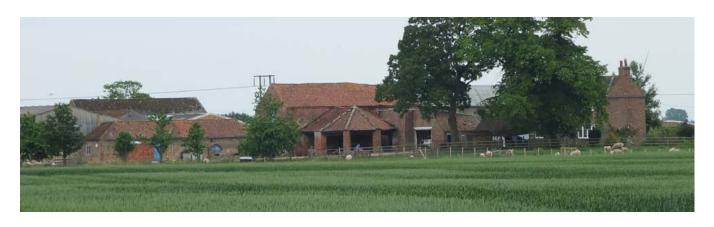
Once a common component of the yard, few horse engine sheds (this having a polygonal roof) now remain. Evidence for them can be found occasionally in roof lines discernible on the rear walls of some barns, while some, as here, still survive. Photo © Jen Deadman
