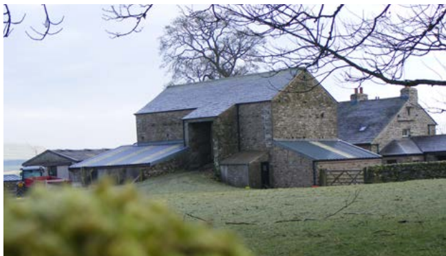
Outskirts of Raisbeck, below Asby Fell, South Orton Fells. A Farmstead with bank barn parallel to the rear of the house, which faces away from the yard. Cattle entries are sited on the yard elevation of the barn. Latterly, a further working building was added to close off the yard area to the north, to form a U-shaped plan. Photo © Jen Deadman
