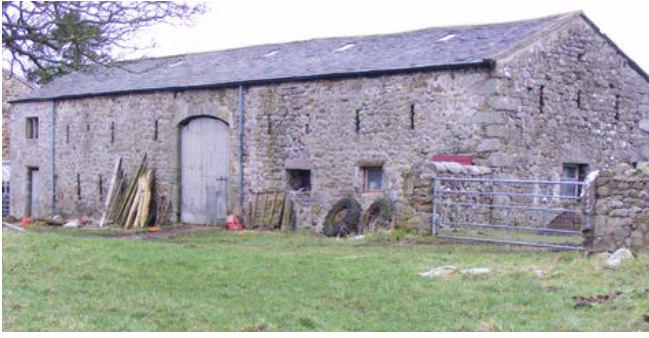
This large, late 18th-century combination barn fronts a yard area. A full-height hay mow flanks the high cart entry to the left, beyond which there is a possible former domestic unit. To the right is a byre with a loft over. There are blocked entries (reduced to windows) on the front elevation. A walled enclosure fronts the building. Photo © Jen Deadman
