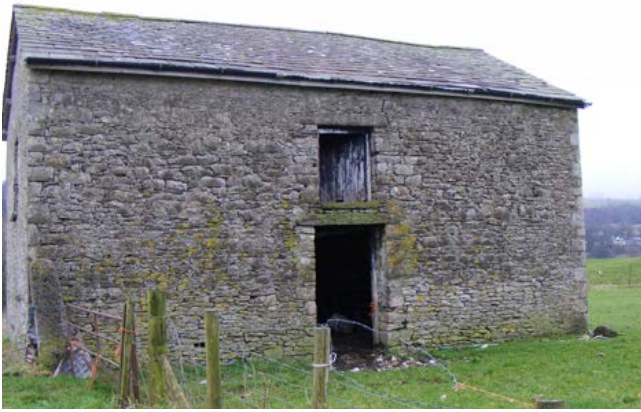
This larger, lofted field barn has an entry in the long elevation. Here, the cattle were possibly tethered either side of the entry. Photo © Jen Deadman
