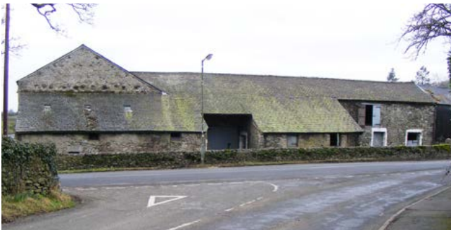
Here, there is a clever amalgamation of the standard combination barn and the part lofted barn, the latter made evident by the large cat slide roofs over the numerous outshots. Photo © Jen Deadman
