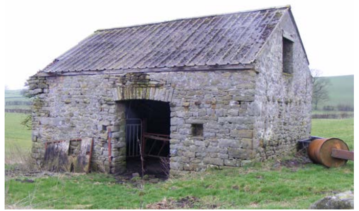
Field barn with cart entry and loft over with a plan form in the style of the part-lofted combination barn. Here the byre was to the right of the entrance and was lofted over. The loft would be served by the forking hole in the gable end. To the left was the open hay mow. Photo © Jen Deadman
