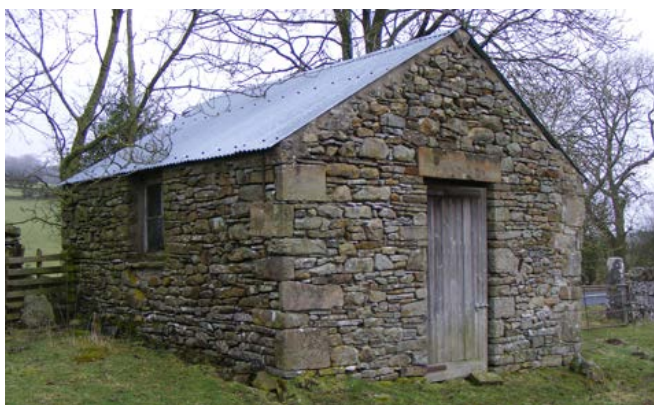
Field barns Field barns take various forms. They can be located against field boundaries or are visible as free-standing structures isolated in the fields. The majority are found on the wide valley floors. They provided shelter for five or six cows and had a hayloft at the upper level. Occasionally, they are single storey, but many are lofted. This example is single storey with an entry in the gable end. Photo © Jen Deadman
