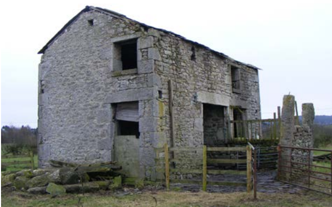
Lofted field barn divided into two unconnected areas, that to the left with an unusual walled enclosure to the front. Field barns, once redundant and with little prospect of alternative use, rapidly deteriorate in condition. Photo © Jen Deadman
