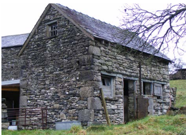
Stables Stables are frequently found as component parts of a combination barn. This mid-19th-century example is a small, free-standing building with a loft over. It is part of the farm complex, but faces out into the field. It has a loft over. Note the slates laid flat over the lintels and the massive sandstone quoins. Photo © Jen Deadman
