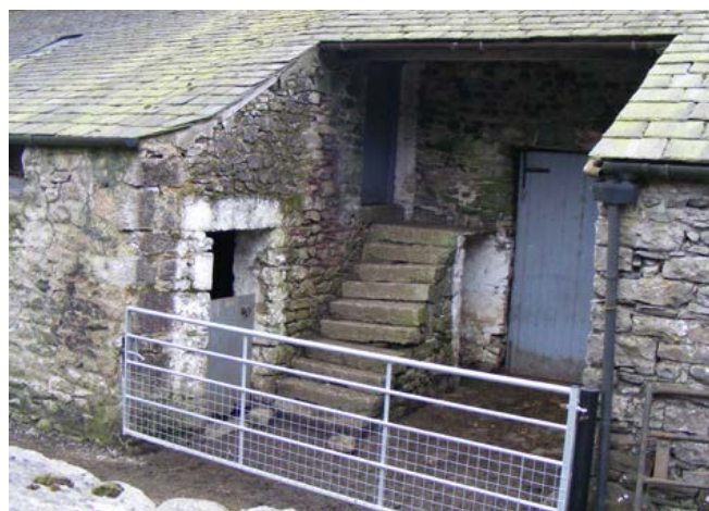
Calf housing Calf housing is often located in the outshots of combination barns. This outshot houses a small calf house with a loft over – the loft accessed by external steps set under the shelter of the pentice roof. A small entry in the loft wall under the eaves was probably designed to allow hens access, via wooden ramp, to the loft. This arrangement is often found above pigsties. A dog hull lies below the steps, again sheltered by the pentice roof of over the cart entry. Photo © Jen Deadman
