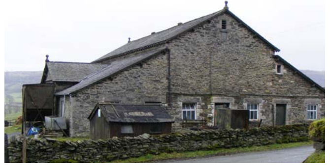
This large combination barn, a late example dated 1904, is a component part of a large, dispersed farmstead of manorial status which lies north of Witherslack. The farmhouse has 16th- to 17th-century origins. The barn has the appearance of the part-lofted plan form with outshots flanking the long elevation. The projecting porch with pitched roof is not found in the 18th-century form of this building. Photo © Jen Deadman
