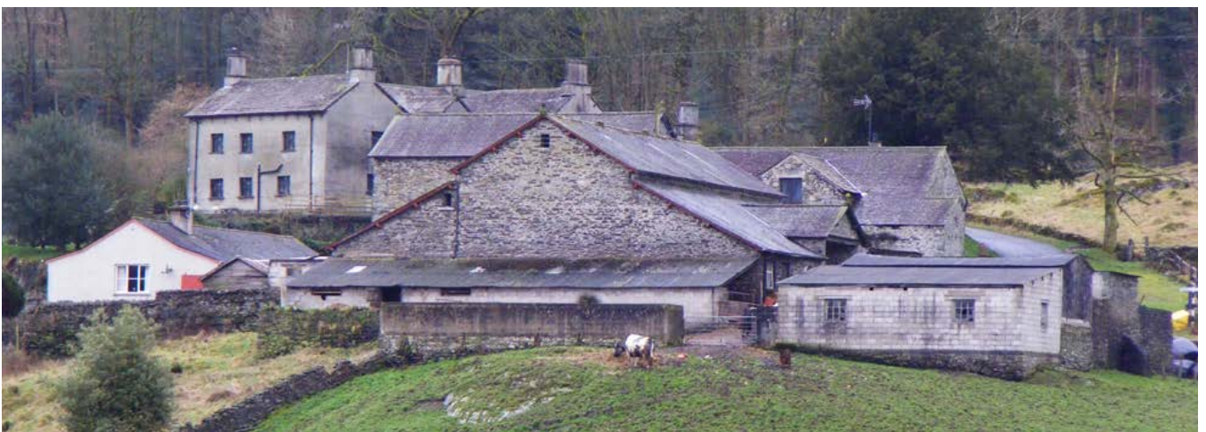
Large, dispersed farmstead sited on both sides of the road in fields of piecemeal enclosure on Cartmel Fell. The sloping site comprises a series of working buildings set one below the other. The farmhouse sits at the highest point and is a large complex with 16th-century origins. Photo © Jen Deadman
