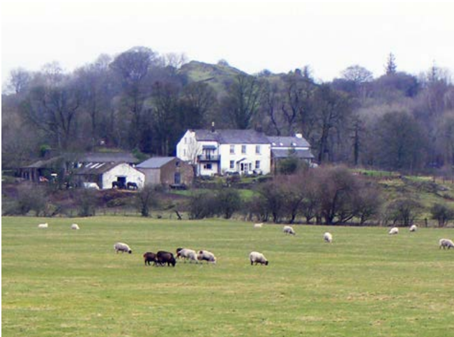
Farmstead on the edge of reclaimed mossland on the Cartmel peninsula, where drained marshland is criss-crossed by large drainage dykes and large rectilinear fields of late enclosure. The mid-19th-century farmhouse faces towards the drained mosslands. Farmsteads sited on the mosslands are frequently 20th century in date. Photo © Jen Deadman
