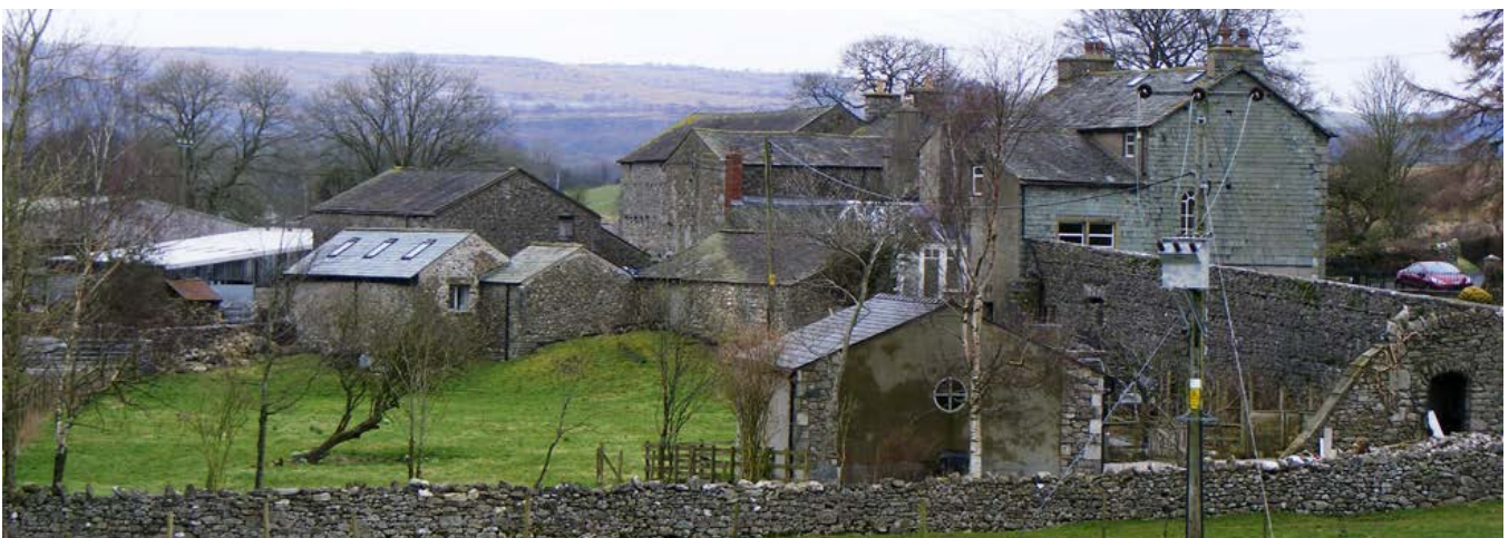
Courtyard plans. Large complex set on the edge of Hilderstone Moss, west of Burton-in-Kendal and the M6 motorway. Individual early to mid-19th-century buildings are set around three sides of a yard with smaller buildings detached from the yard. The house looks away from the group, this being found on larger and high-status farmsteads. The surrounding land mossland has been drained and divided up into neat, rectilinear parcels. Photo © Jen Deadman
