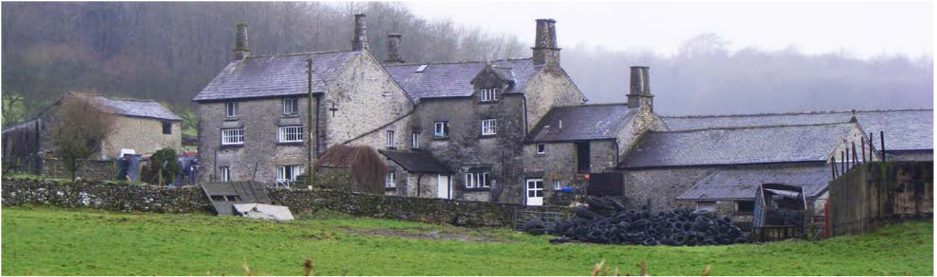
Flodder Hall. Large, gentry farm of 16th-century origins with later additions. This is one of a string of farmsteads, some of which are very large, which lies below Whitbarrow Fell on the west side of the Lyth valley, above the River Gilpin. The land immediately below, on which the majority of the farmsteads sit, is comprised of small, irregular fields of earlier enclosure. The land below (Lyth Moss), has been drained and presents a landscape of rectilinear fields of late enclosure. The high-status house looks away from the loose courtyard group of buildings and towards the mosslands. Photo © Jen Deadman
