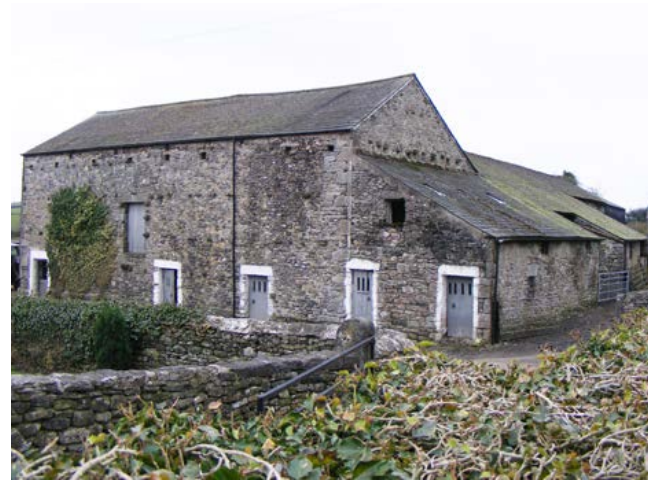
Farmstead occupying corner plot in the village of Ackenthwaite. Large, early to mid-19th-century combination barns are conjoined to accommodate cattle housing and hay storage, both in the main body of the buildings and in outshots. Photo © Jen Deadman
