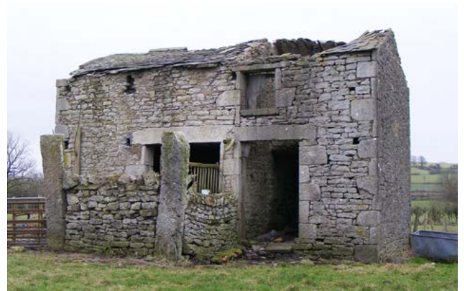
Lofted field barn divided into two unconnected areas, that to the left with an unusual walled enclosure to the front. Field barns, once redundant and with little prospect of alternative use, rapidly deteriorate in condition. Photo © Jen Deadman
