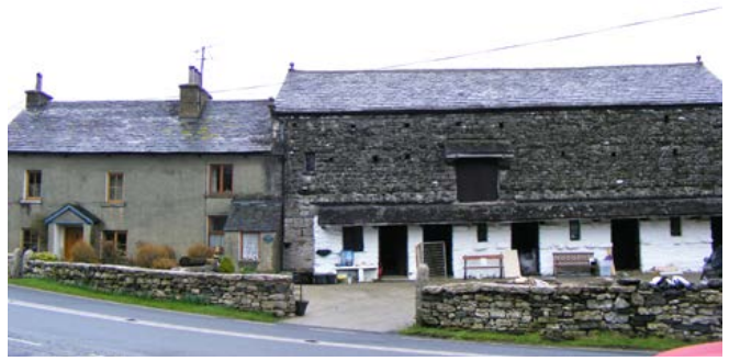
South Low Farm, north of Flodder Hall. The late 17th-century house with large combination barn attached lies close to the roadside with a walled holding enclosure to the front. A second barn is set parallel behind, with a free-standing stable forming the third side of the yard. Note the continuous canopy, a typical feature. Photo © Jen Deadman
