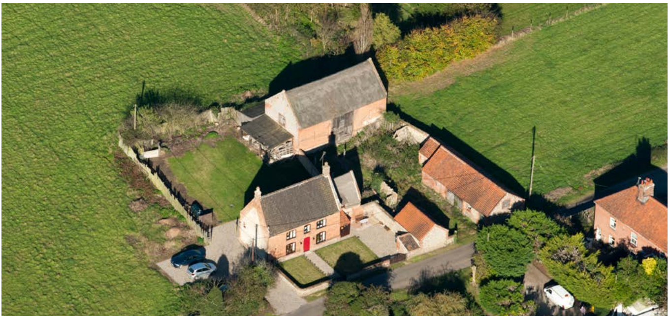
A small-scale early to mid- 19th century farmstead at Ridlington Witton, showing a three-bay reed-thatch barn. Photo © Historic England 29192/038
