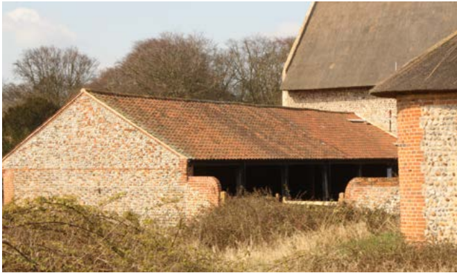
Shelter sheds From the 18th century, but more commonly in the 19th century, single-storey, open-fronted buildings were constructed for cattle. These shelter sheds usually faced into cattle yards and were often attached to an earlier barn, resulting in regular courtyard plan types. Photo © Bob Edwards
