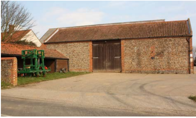
This 19th-century, five-bay barn lies near the coast and is largely constructed from cobbles with brick dressings. Although it has coped gables, it is probable that it has always been roofed with pantiles. As is commonly seen in the area, an attached shelter shed creates an L-plan range. Photo © Bob Edwards
