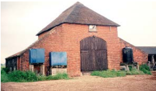
The hipped roof and aisles to this building at Freethorpe (see p. 10), give it a very distinctive form. The double doors provide access to a root store for feeding turnips to cattle which are housed in loose boxes in the aisles. This building type, recorded in the late 18th century but mostly 19th century in date, is confined to The Broads (NCA 80) and the area around it. Photo © Susanna Wade Martins
