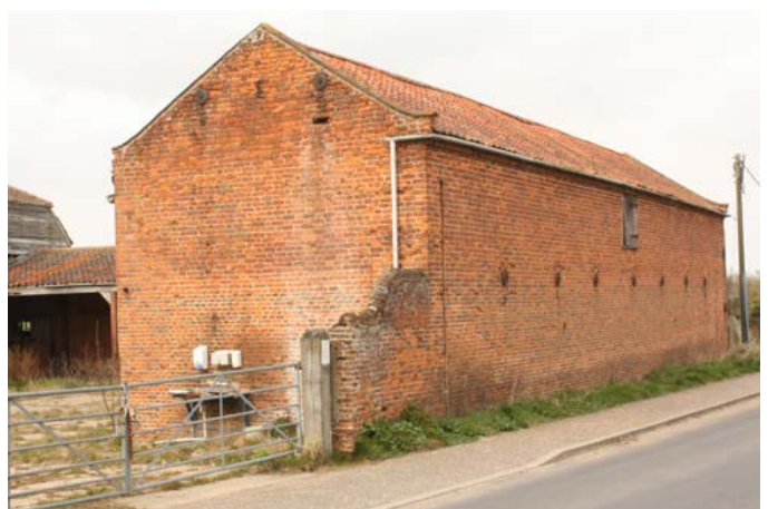
A large, two-storey stable on a Manor Farm. The size of the building indicates that this farm had a large team of horses to work the arable lands. Closer inspection of the building, which initially appears to be 18th or early 19th century in date, shows that it is a building of at least two phases with thinner, early bricks to the lower part of the rear wall and later brickwork above, showing that the stable was raised to two storeys. Photo © Bob Edwards
