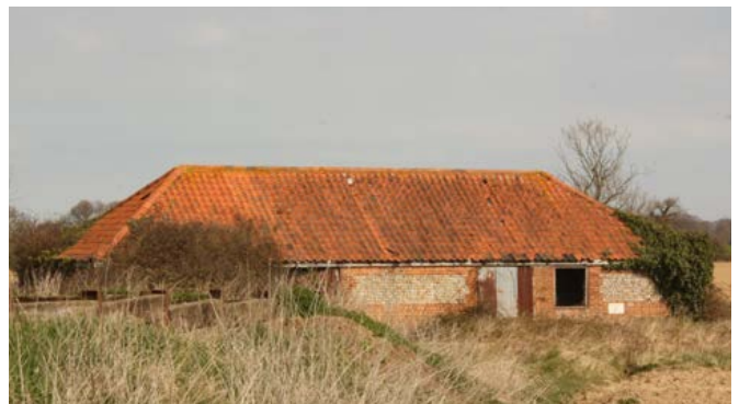
Outfarms or field barns do not appear to have been numerous in the landscape, but there are surviving examples. This building provided housing for cattle near the fields where their manure would be used as fertiliser. Photo © Bob Edwards
