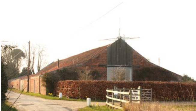
This large, barn-like building provided storage in the main body of the building, probably for root crops, particularly turnips, and cattle housing in loose boxes in the aisles. This is a building type that is characteristic of this area. Photo © Bob Edwards
