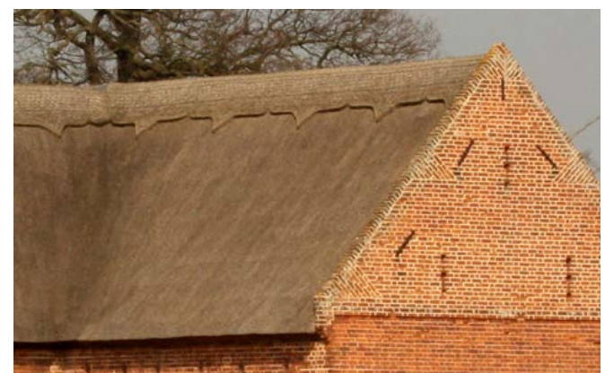
Reed thatch on a brick barn with coped gables incorporating tumbled brickwork, these being highly characteristic materials and features found across the area. Photo © Bob Edwards
