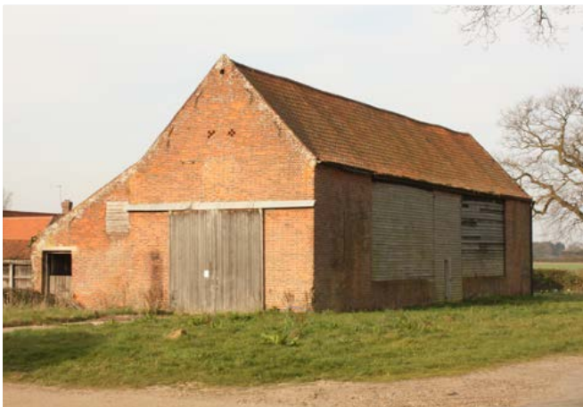
This five-bay barn also has a contemporary aisle to the rear although the end door suggests that the aisle provided cattle housing. As in most cases where the aisle provided animal housing, there is a change in the pitch of the roof over the aisle in order to ensure sufficient headroom for cattle. The barn is one of a relatively small number in the area that incorporate timber-framing in the front wall. The large door in the gable is a later insertion. Photo © Bob Edwards.
