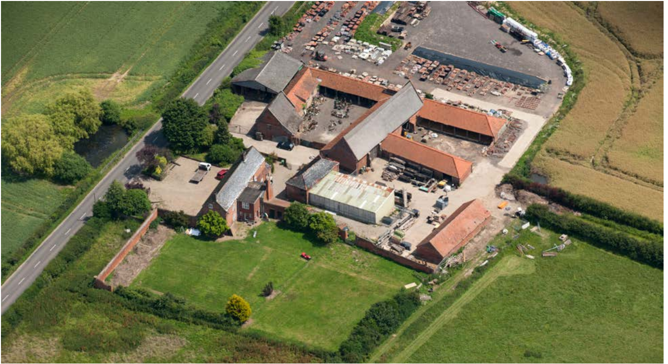
At the core of this large-scale farmstead is a threshing barn with two threshing bays, flanked by two cattle yards. The barn, like the granary/stable to the left, dates from the mid- to late 18th century. Photo © Historic England 29125/050
