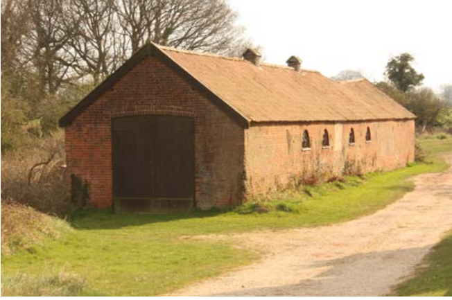
This single-storey stable with a single-bay trap house at the end is typical of stables of the mid to late 19th century when the importance of good ventilation for the horses was better understood. This led to the construction of single-storey buildings without a hay loft and often the use of ridge vents. The use of lunette windows is a feature often found on stables in this area. Photo © Bob Edwards
