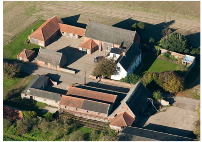
A characteristic regular multi-yard plan at Lessingham, showing the late 17th- and 18th- century house and two threshing barns. Also belonging to this earlier phase is the stable block and cartshed facing the road. The cattle yards include a covered yard attached to the nearside barn. Photo © Historic England 29191/046
