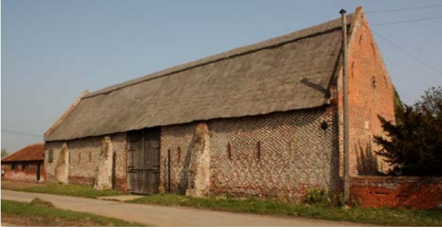
Barns This seven-bay, 17th-century barn is part of a manor farm located on the drier ground on the edge of the marsh. The lower part of the wall displays diaper patterning in brickwork but has chequer pattern above possibly indicating rebuilding. The upper parts of the gable have also been rebuilt in red brick. Photo © Bob Edwards.
