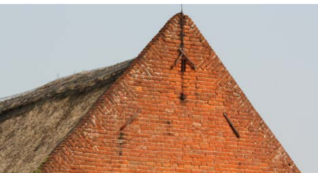
Tumbled brickwork, the setting of bricks at an angle to form the coping of the gable, is a characteristic of Norfolk architecture. Photo © Bob Edwards.
