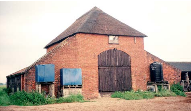
The hipped roof and aisles to this building, at Freethorpe in NCA 79 (North East Norfolk and the Flegg), give it a very distinctive form. The double doors provide access to a root store for feeding turnips to cattle which are housed in loose boxes in the aisles. This building type, recorded in the late 18th century but mostly 19th century in date, is confined to The Broads and the area around it. Photo © Susanna Wade Martins
