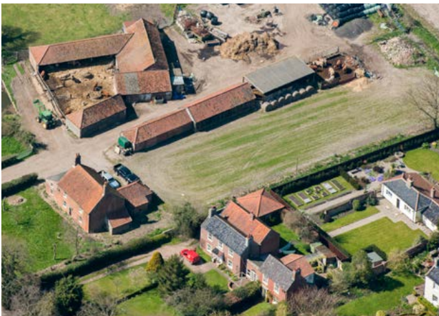
At the core of this farmstead at Somerleyton, as rebuilt in the mid 19th century around an earlier barn, is a cattle yard with a lean-to for cattle – another typical feature – also added to the barn. Photo © Historic England 29350/020
