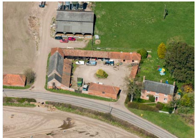
A regular courtyard arrangement with buildings built around all sides of the yard at Somerleyton. Note the farmhouse, characteristically detached and facing into its own garden, and the earlier reed-thatched threshing barn with its 19th-century lean-tos. Photo © Historic England 29350/ 039
