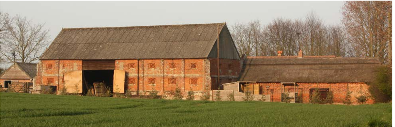
A large 19th-century brick barn with distinctive ventilation holes in the brickwork. Photo © Bob Edwards.
