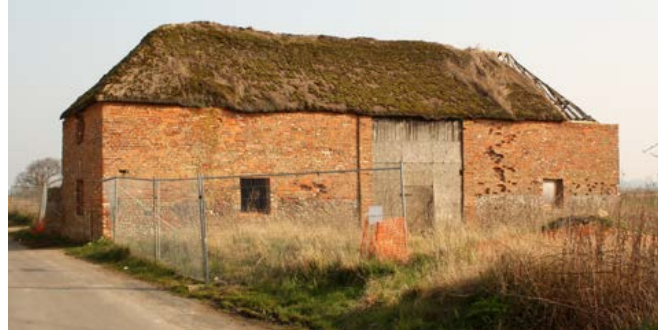
A mid-18th-century brick-built barn, having a hipped roof rather than the gables typical of earlier barns. To the rear was a single-storey lean-to, possibly for cattle. This barn was one of two barns on this farm, the second barn being a slightly smaller, late 17th-century or early 18th-century, three-bay, brick building. Photo © Bob Edwards.
