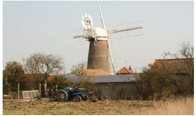
Windmills The drainage of the marshland depended on the use of windmills to drive the pumps. Most of these windmills stood alone in the marshland but occasionally they are associated with small farmsteads. Photo © Bob Edwards.
