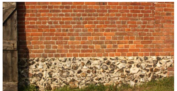
Whilst flint cobbles were commonly used in farm buildings, broken or knapped flint is less frequently seen. Photo © Bob Edwards.
