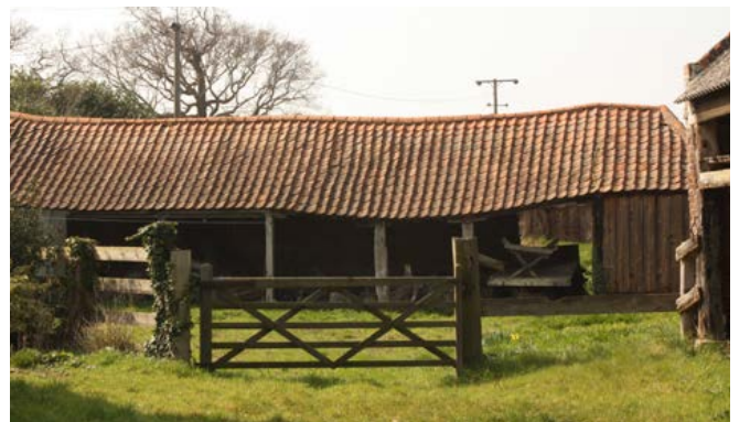
Cattle housing The most common form of cattle housing is the open-fronted shelter shed, a single-storey building that faces into a yard. Most are of 19th-century date. Examples from the 18th century are very rare and significant. Photo © Bob Edwards
