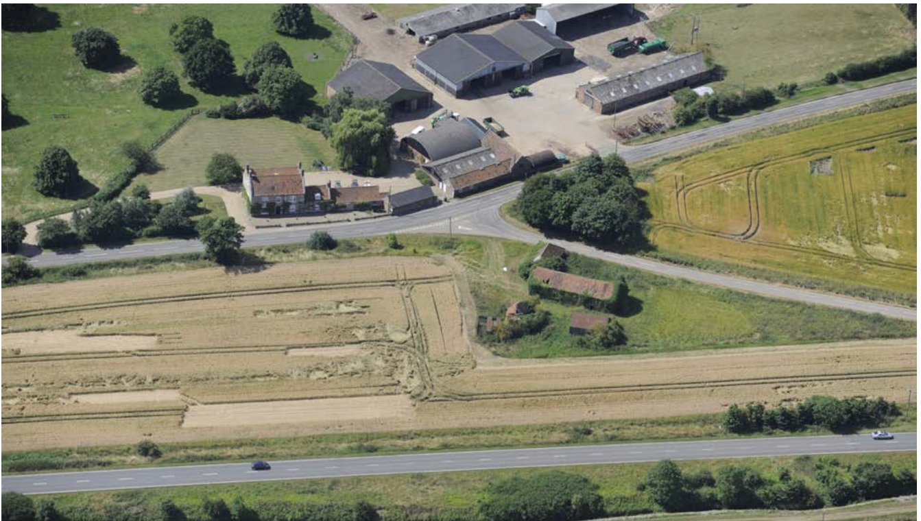
Priory Farm, Bridge End. A dispersed multi-yard complex with 18th-century buildings set at one end of an ancient causeway across the western fens. The farmhouse appears to be an older, linear farmstead with working buildings attached in line. Large, modern buildings have been added to the complex while historic buildings typically used for housing livestock are disused. Photo © Historic England 28555/018
