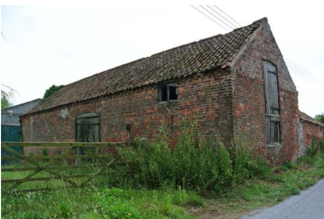
Disused combination barn with a gable-end loading door to a first-floor granary over stables, Donington Fen. The barn comprises one side of a regular L-plan courtyard with cattle sheds in the adjacent range, indicating a typical mixed or arable farming operation. The farmhouse itself is set behind the complex facing into the wider landscape and away from the working buildings. Photo © Locus Consultants
