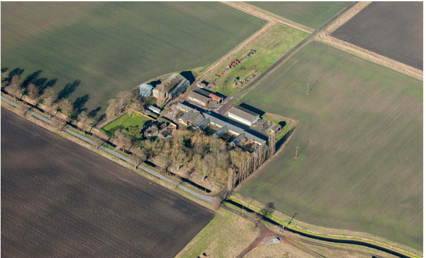
The High Farming years of the mid-19th century saw investment by estates in many farmsteads with barns for processing corn and feed for livestock, with two or more yards for cattle in E-shaped or even double-E plans as here at Knarr Cross, within an area drained and enclosed in the early 17th century. Pre-19th-century buildings are very rare in these landscapes. Photo © Historic England 29327/016
