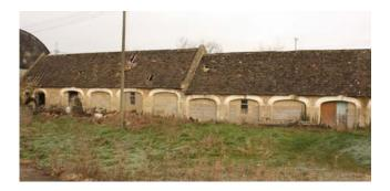
Open-fronted shelter sheds are the most common building type on farmsteads in this area. They are typically stone built with timber posts to the open front but here, in the west of the area, they have stone piers. Photo © Bob Edwards
