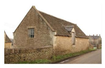
Large stables are not common in this area due to the limited extent of arable; only the larger farms having substantial stables. This example is of two storeys with the hay loft accessed from the road, which is higher than the yard, and a cart shed accessed from the far gable end. Photo © Bob Edwards
