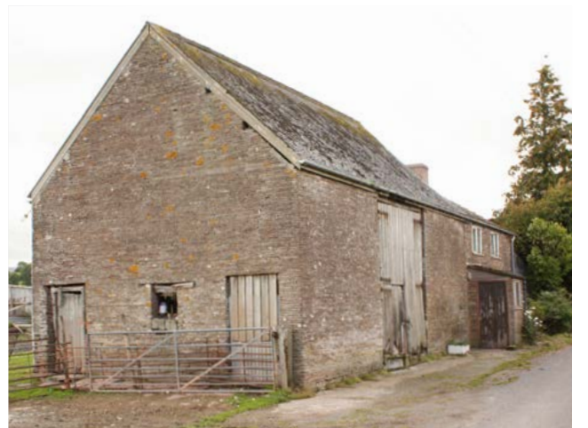
A combination barn in the Black Mountains, of a type commonly found in Wales. The doors in the gable end provide access to a cow house. Photo © Bob Edwards
