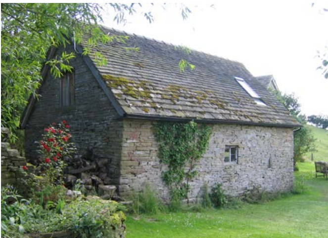
The rear of a small threshing barn in the Black Mountains. Note the small winnowing hole which is sited opposite the entry to the threshing floor. Photo © Jeremy Lake
