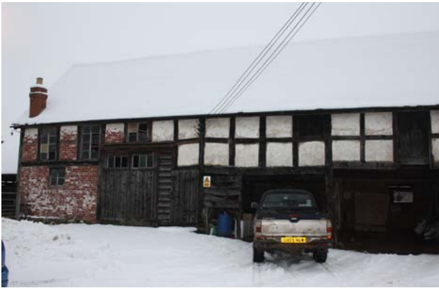
A timber-frame combination range, with a first-floor door on the right to the granary and a threshing bay to the left. Photo © Bob Edwards
