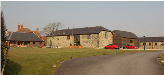
A large, loose courtyard group with working buildings to four sides of the yard on a mixed farm that clearly had considerable arable, as it has two threshing barns, one a staddle barn, with ranges of cattle housing to two-and-a-half sides of the yard with the stable (behind the staddle barn) set at right angles to the main yard area. The farmhouse, standing off to one side of the yard, looks out across the landscape. The cart shed to the left faces onto the track leading into the farmstead. Photo © Bob Edwards
