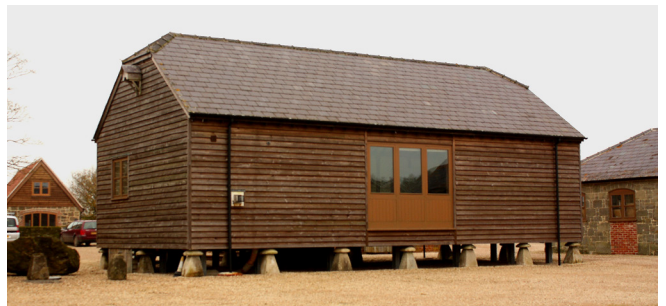
A staddle barn built on one of the larger farms in the area which also had a conventional threshing barn. This barn is an outlier from the main concentration of this type of barn in the chalk downland of Wiltshire, west Hampshire and Berkshire. Photo © Bob Edwards
