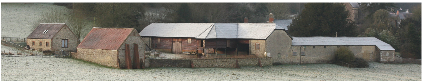
This regular courtyard plan farmstead was built in the mid-19th century on the Longleat Estate and represents one of the larger farmsteads in the Character Area. The large barn has a projecting horse engine house attached on the side of the stack yard and has single-storey ranges for cattle facing into the main yard area beyond the barn. Photo © Bob Edwards
