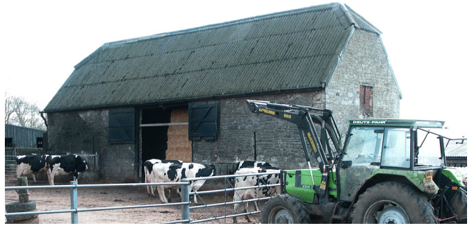
A five-bay threshing barn with half-hipped roof, probably formerly tiled or thatched. Photo © Bob Edwards
