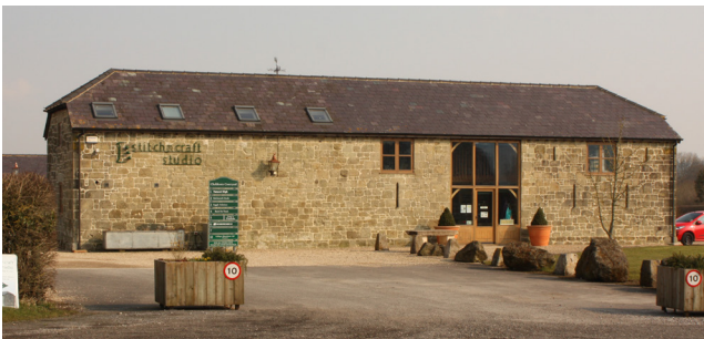
A large, combination barn range that consists of a threshing barn of four or five bays with animal housing to the left part. Photo © Bob Edwards
