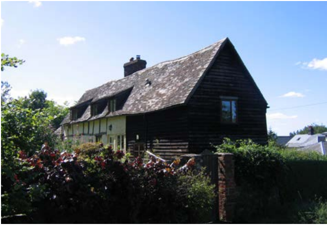
A rare surviving example, to the west of the area, of a timber-framed linear farmstead of the 17th century or earlier, where the house and working buildings are attached and in-line. Photo © Bob Edwards
