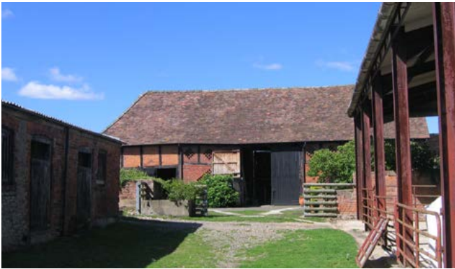
Some substantial timber-framed barns of the late 16th and 17th centuries have survived, with the distinctive square panel timber framing typical of the western English carpentry tradition. Photos © Bob Edwards
