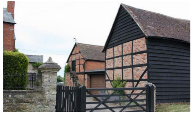
Some substantial timber-framed barns of the late 16th and 17th centuries have survived, with the distinctive square panel timber framing typical of the western English carpentry tradition. Photos © Bob Edwards
