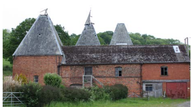
In the mid- to late 19th century, when much of the Malverns was developed with suburban-style villas and houses, the large farms of this area were provided with industrial-scale buildings such as this combination barn (left) and hop kilns and stowage. Photo © Bob Edwards
