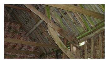
A barn with a 'sling brace truss': a 19th-century truss type that is rarely seen outside of Dorset. The diagonal timber is a later addition. Photo © Bob Edwards
