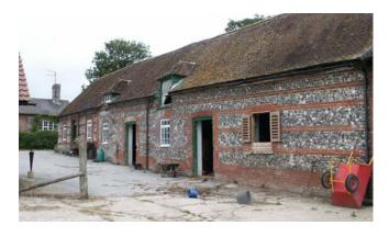
A large, brick and flint stable range reflecting the number of horses required to work the large arable farms in the downs. The hayloft over indicates that this is an 18th or early 19th-century example, later examples usually being single-storey to provide better ventilation for the horses. Photo © Bob Edwards
