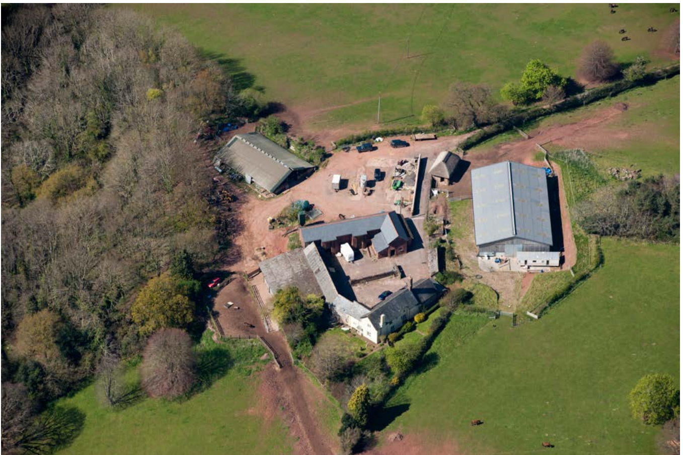
Holt Ball Farm on the Selworthy estate, where farms were amalgamated and restructured from the 1820s. The farmhouse is the earliest building, attached to a dairy and linhay for cattle, cattle and horses also being housed in the ground floor of the threshing barn, which was built with two threshing bays. Note the cart shed facing the entrance routeway. Photo © Historic England 27981/016
