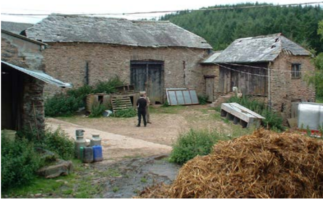
The traditional threshing barn is widely found on Exmoor. This example from the southern fringe is a good size for its small farmstead, and indicates the expansion in corn farming during the boom times of the late 18th and the 19th centuries. Attached at the corner is the granary. Photo © Philip White
