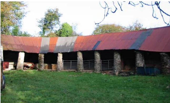
Cattle housing These otherwise typical Exmoor shelter sheds with round piers have an unusual, curved layout only known at one other location. Photo © Philip White
