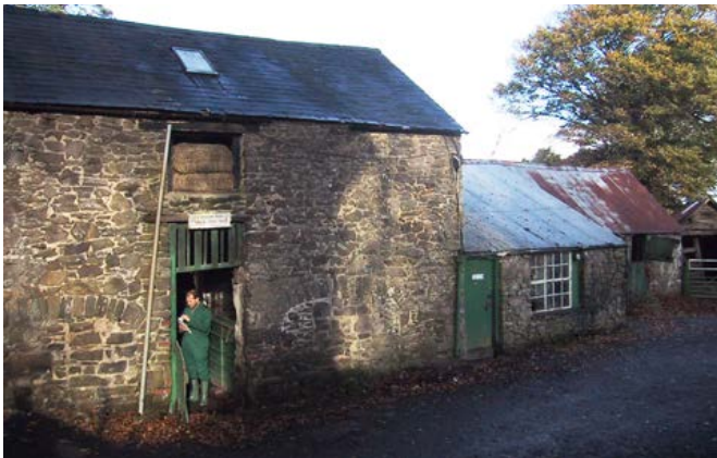
This form of lofted cattle house with full-height narrow entrance is found only occasionally in the West Country. The arched cattle entrances to the cow house were infilled when its use changed. Photo © Philip White
