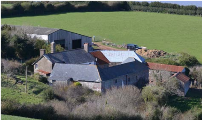
This regular, multi-yard plan developed with two yards. The stabling and main barn with cattle housing is housed in the tall buildings which, together with the house, enclose the main yard. Downslope is an additional cattle yard. This multi-yard arrangement is repeated across Exmoor, with many variations. Photo © Philip White
