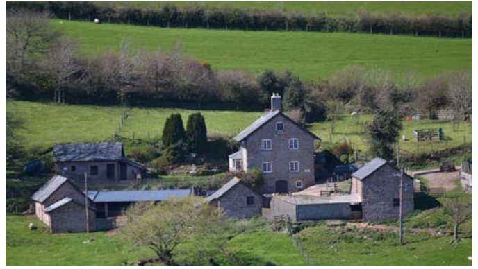
This late 19th-century, smaller-scale group has also developed around two yards. Many farmsteads were rebuilt in the late 19th century, after the 1870s, which often marks the last phase of farm building in England. Photo © Philip White
