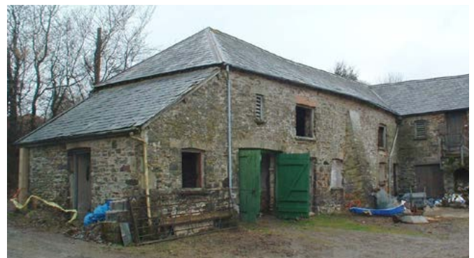
Cart sheds will generally house one or two carts and are often attached to, or as here, are part of another building. They are also found as lean-tos. Photo © Philip White
