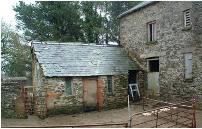
Other building types Pigsties usually take a similar form to the typical Devon or Cornwall style. This pigsty has a separate access on the right to provide feed without entering the sty itself. Photo © Philip White
