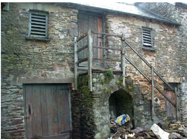
Granaries Granaries at first-floor level are the most typical type on Exmoor. They always feature steps and are most often found over animal houses, from dog kennels to stables. The steps shown have a recess for a dog or goose, intended to ward off rats. Photo © Philip White
