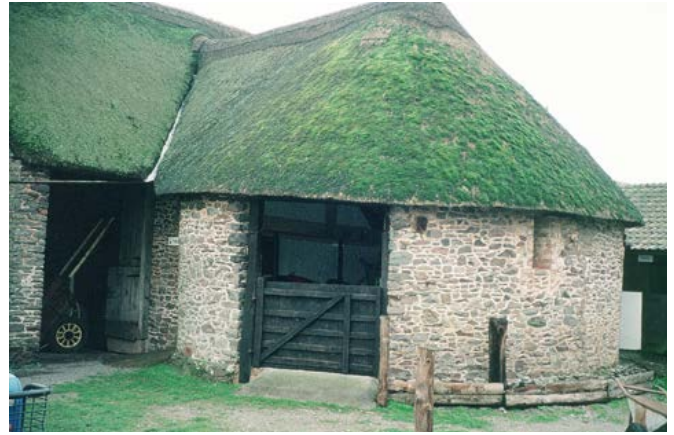
An engine house for horse-powered threshing machinery. Historic maps show that many barns had attached engine houses, but surviving examples are now rare. Photo © Jeremy Lake
