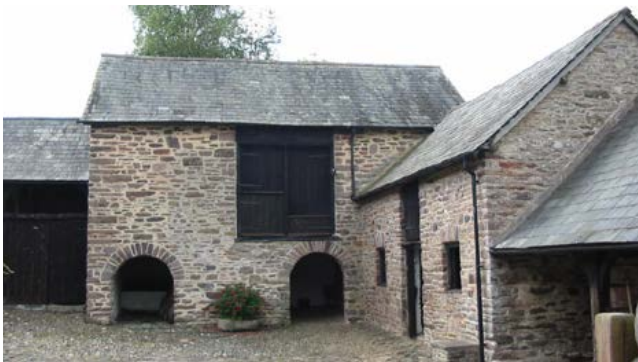
Barns This small bank barn is typical of the many small, courtyard farmsteads on Exmoor. It provides evidence of the regional character seen in Exmoor buildings. The low cattle arches may indicate use by calves. Attached to the right is a stable with a hay loft. Photo © Philip White
