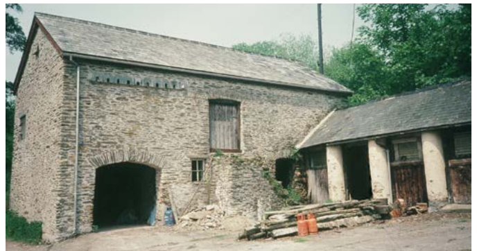
This is another typical arrangement – a barn with attached linhay. The barn is a bank barn. The upper threshing and crop storage area is accessed from the bank to the rear: next to the threshing floor is a platform for a horse walk, for powering a threshing machine inside the barn. A cart shed and a stable face the farmyard, and pigeon holes are also built into the front elevation. Photo © Jeremy Lake
