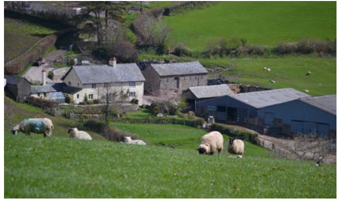
Courtyard plans A loose courtyard plan. To the right of the house is a yard now flanked by two opposing buildings, and prominent to the right is a bank barn. There are small buildings, possibly for calves, to the left of the house. Photo © Philip White
