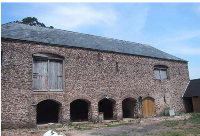
This large bank barn, dating from c.1800 served an estate farm. It had two threshing floors and one winnowing door, later reduced in size. To the rear is a rare, two-storey round house. The cow house below opened on to one large yard. Photo © Philip White
