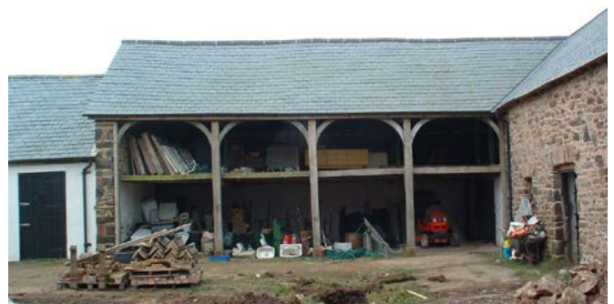
Linways with timber posts occur more often around the high moor than on it and this shows a typical three- to five-bay arrangement with curved braces. Oak was the obvious choice originally but softwood posts are found, usually as replacements. Photo © Philip White
