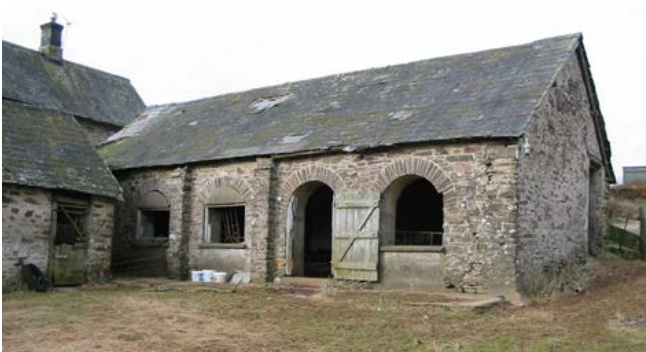
Some shelter sheds are designed both to provide greater protection and for feeding, whilst still allowing free access to animals. They are generally found in more exposed yards. Most openings in this building have been partly blocked up. Note the feed passage door in the gable. Photo © Philip White
