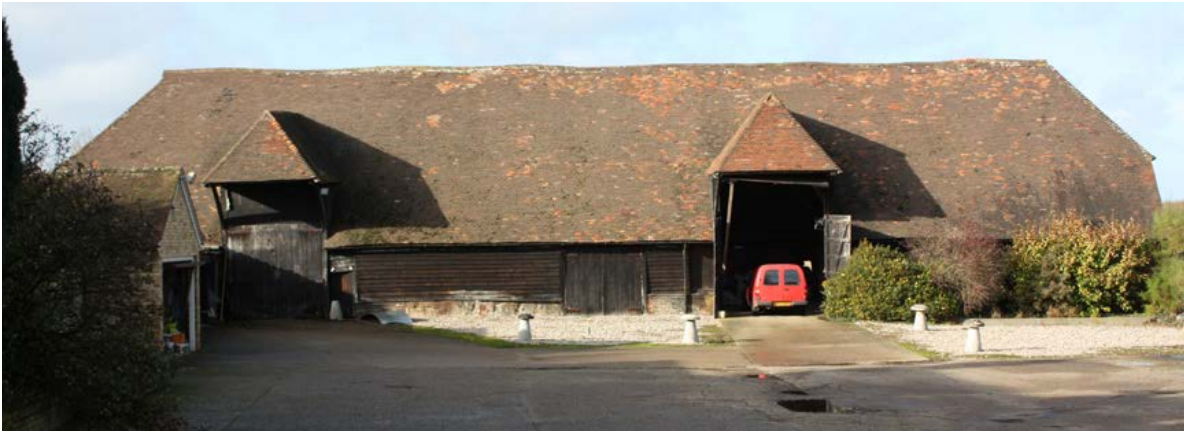
Large, timber-framed, aisled threshing barns dating from the 14th to 17th centuries are one of the defining building types within this area. Photo © Bob Edwards
