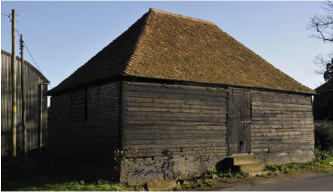
A large granary raised on a plinth wall rather than staddle stones. © Historic England
