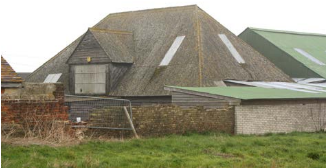
A three-bay, aisled barn of 17th-century date on a small farmstead, Hoo. Photo © Bob Edwards
