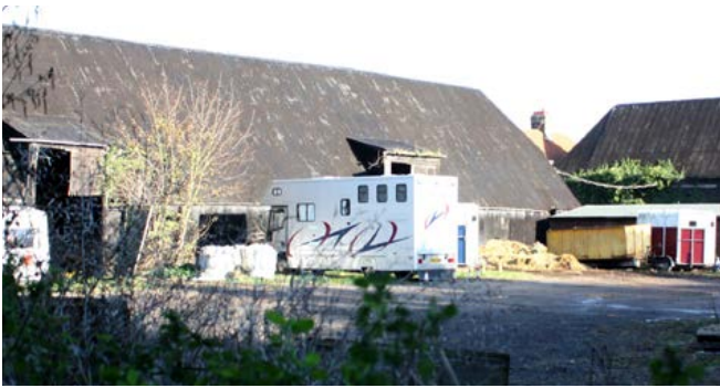
Medium to large-scale, loose courtyard plans were predominant in this area, particularly in the north-east where two or more large threshing barns, stables and granaries would be set around a yard. Photo © Bob Edwards
