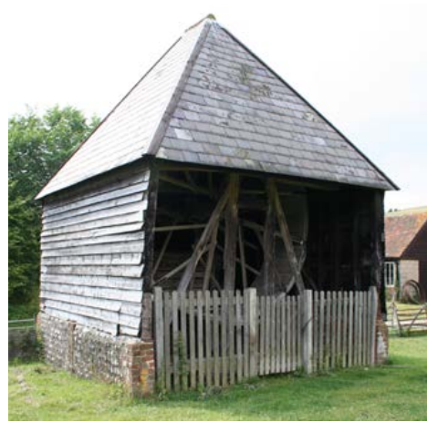
A surviving example of a donkey wheel for drawing water from a well. Photo © Bob Edwards
