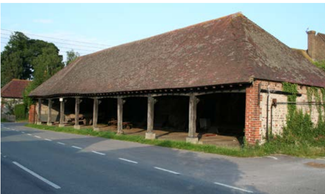
A very large cart shed of nine bays. Examples such as this served large arable-based farms. The cart shed typically faces away from the farmyard and onto the street. Photo © Bob Edwards
