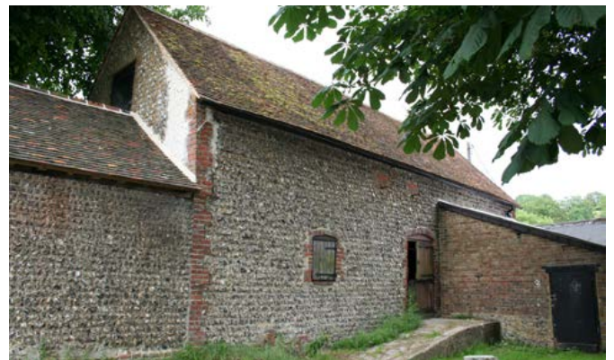
A large stable reflecting the need for large teams of horses on the arable farms of the area. The small window and loft above for storage of fodder indicates that it was built in the 18th or early 19th century. Photo © Bob Edwards
