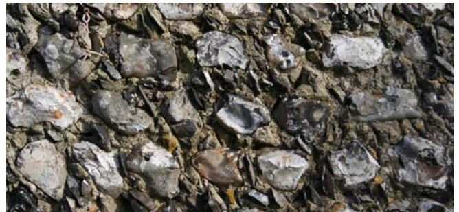
Flint walling, with flint galleting infilling the mortar joints, is rarely seen in other downland areas of southern England. © Photo © Bob Edwards
