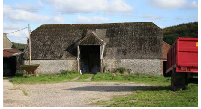
A typical five-bay barn, aisled to the rear and built in flint cobble. Photo © Bob Edwards
