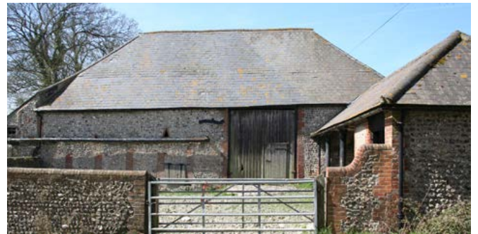
A barn with a later shelter shed attached to form an L-plan is a common arrangement. Photo © Bob Edwards
