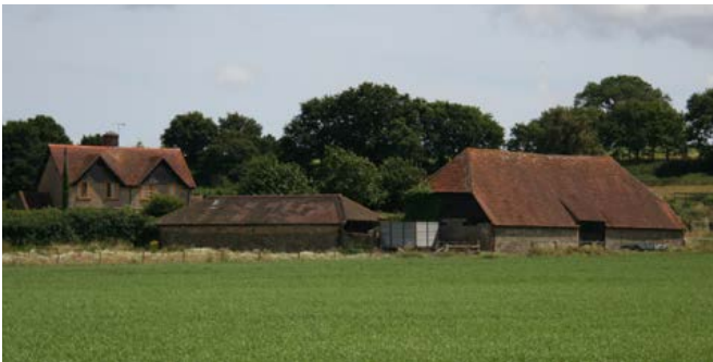
Loose courtyard plans with detached buildings set around a yard were the predominant farmstead type across the Character Area. Photo © Bob Edwards
