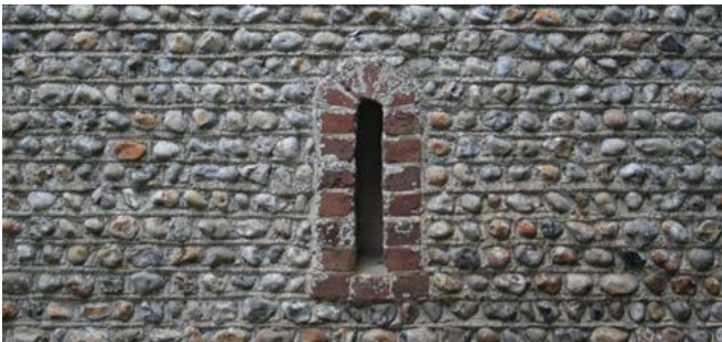
The use of cobbles for walling is characteristic of the area. Photo © Bob Edwards
