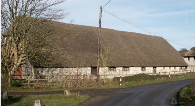
A large aisled threshing barn built in the 15th century on one of the Bishop of Winchester's estates, at Hensting in Hampshire. In the 17th century, a bay was added to provide stabling. Photo © Bob Edwards
