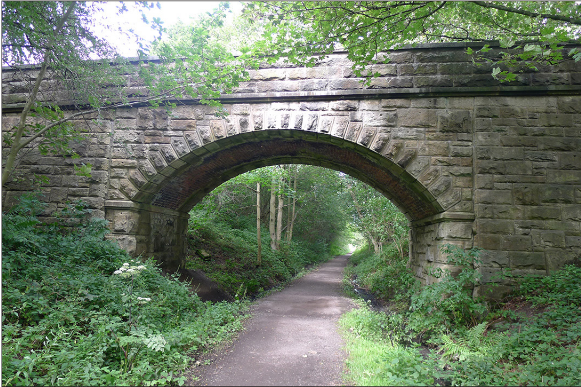
Fig 46. Southern elevation of railway accommodation bridge BIF/12. (© Historic England/Marcus Jecock)
