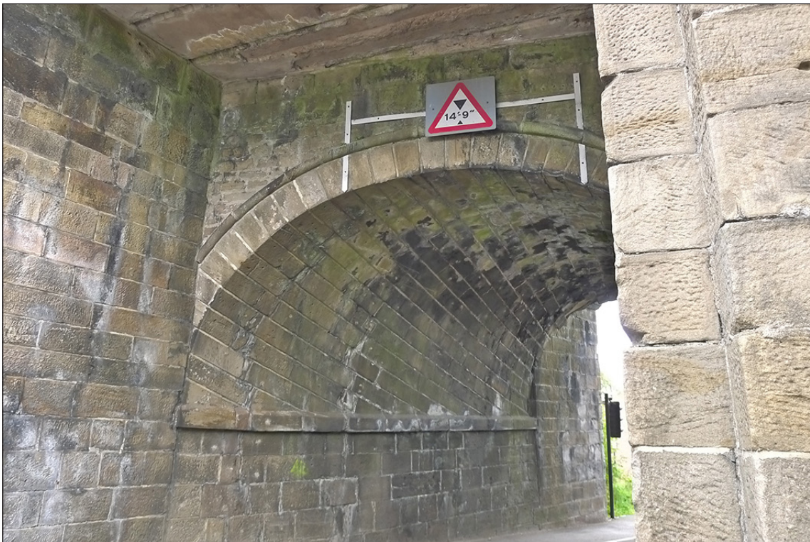
Fig 53. Detail of the original western elevation of railway underbridge DAE2/4 (High St, Coundon Grange), showing arch ring, archivolt and impost banding. (© Historic England/Marcus Jecock)
