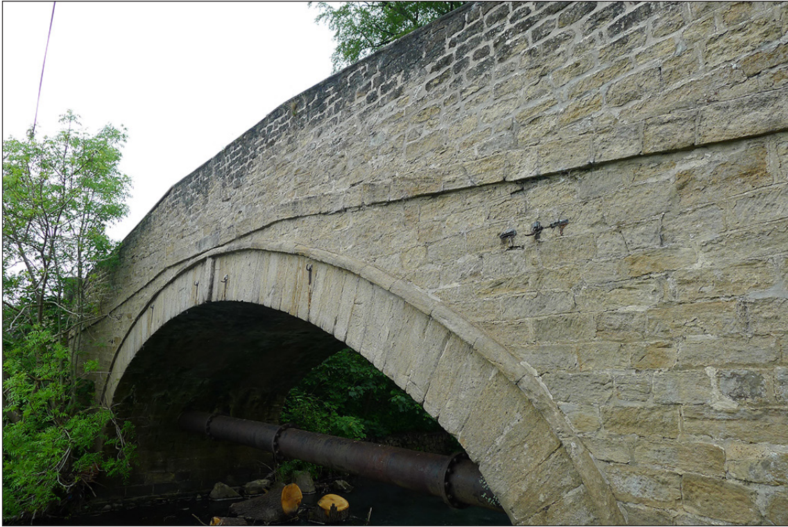
Fig 11. The western (downstream) elevation of Jock's Bridge. Note the humpbacked form of the string course at deck level mirrored by the parapet above. (© Historic England/Marcus Jecock)
