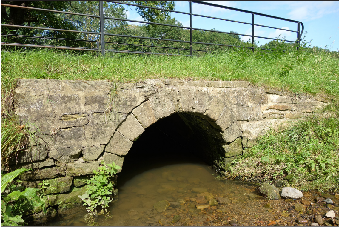
Fig 80. The eastern headwall of 'Bishop Trevor's' culvert for the Coundon Burn in Auckland Park. (© Historic England/Rebecca Pullen)
