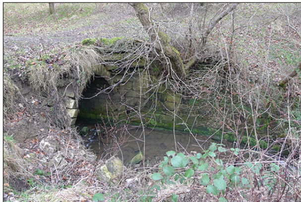
Fig 85. The eastern elevation of ‘footbridge no. 1’ across the Coundon Burn in Auckland Park. Note the corbelling in the north-east spandrel to ease the passage of the footpath on to the bridge, and the short length of training wall. (© Historic England/Marcus Jecock)
