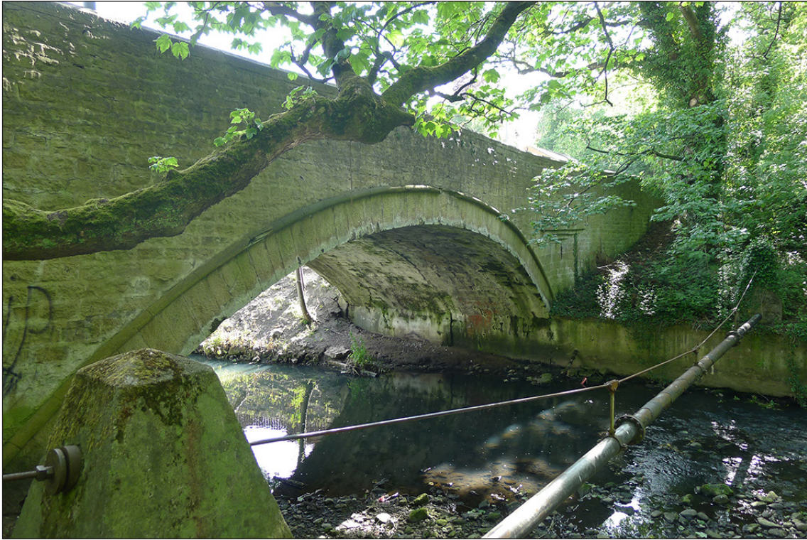
Fig 17. The northern (downstream) elevation of the phase-2 Gaunless Bridge. (© Historic England/Marcus Jecock)
