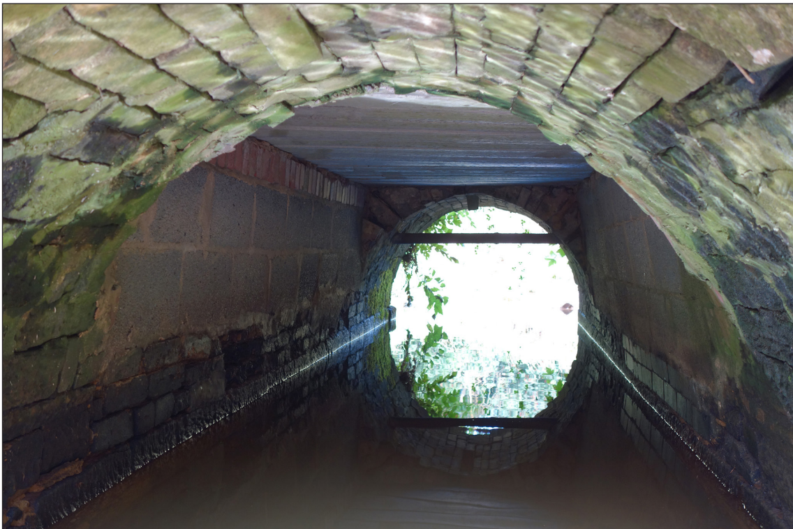
Fig 81. Detail looking through the arch barrel of 'Bishop Trevor's' culvert for the Coundon Burn in Auckland Park, showing the central section rebuilt and re-decked in modern materials. (© Historic England/Rebecca Pullen)
