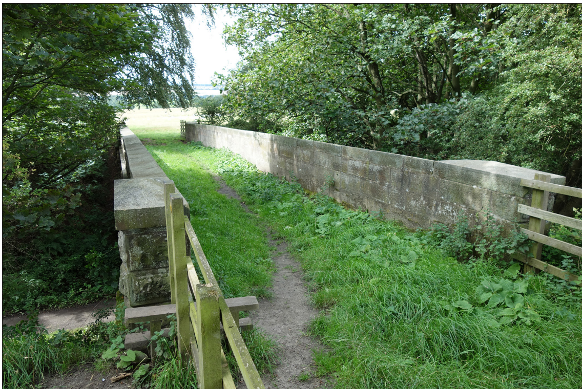
Fig 48. View west along deck of railway accommodation bridge BIF/12, showing parapets and end piers. (© Historic England/Rebecca Pullen)
