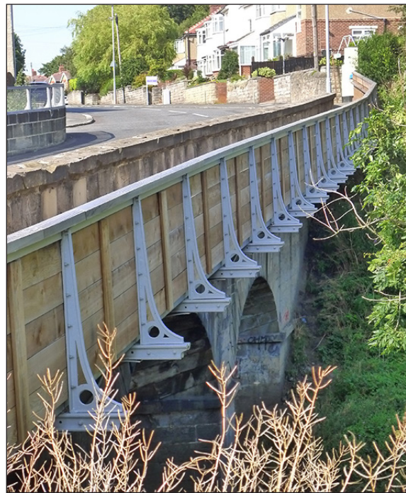
Fig 73. The Victorian pedestrian walkway cantilevered out against the eastern elevation of railway overbridge DAE2/11 ('Latherbrush Bridge'). (© Historic England/Marcus Jecock)
