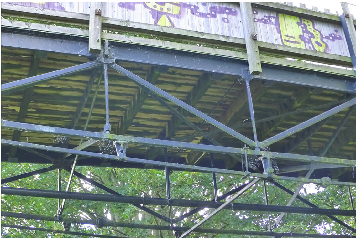
Fig 75. Detail of the chords, truss structure and cross-bracing of railway accommodation overbridge DAE2/12 (lenticular truss). (© Historic England/Marcus Jecock)
