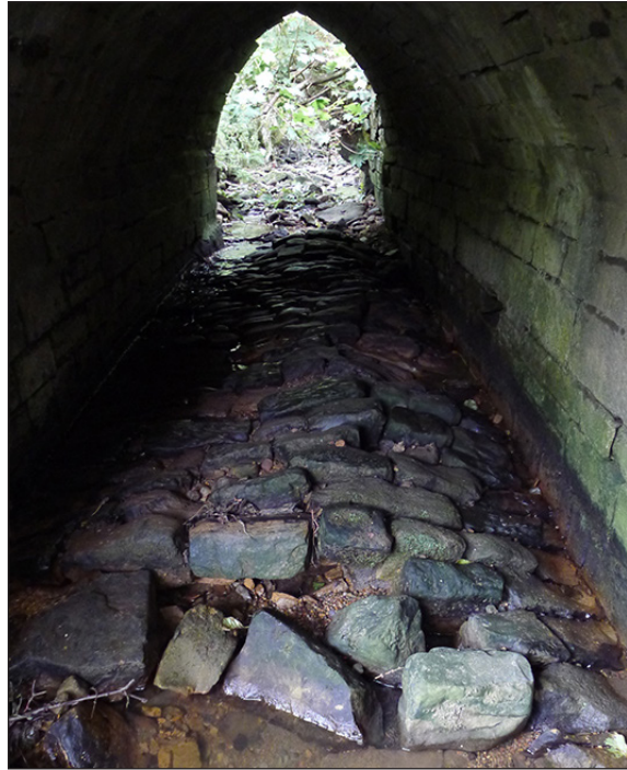
Fig 86. View beneath 'footbridge no. 1' across the Coundon Burn in Auckland Park. Note the deformed and disintegrating paved invert. © Historic England/Marcus Jecock)
