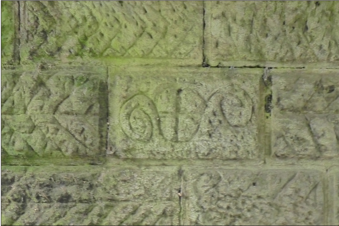
Fig 61. Detail of the cartouche in the centre of each abutment of railway underbridge DAE2/7 (Bone Mill Bank). (© Historic England/Marcus Jecock)
