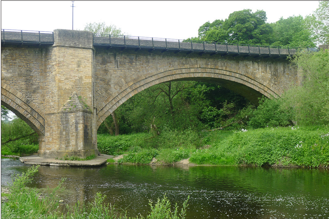
Fig 6. The northern arch of Newton Cap Bridge from the east. Note the fourth arch ring, and the off-centre voussoirs close to the springing from the pier with signs of patching in the spandrel above. (© Historic England/Marcus Jecock)
