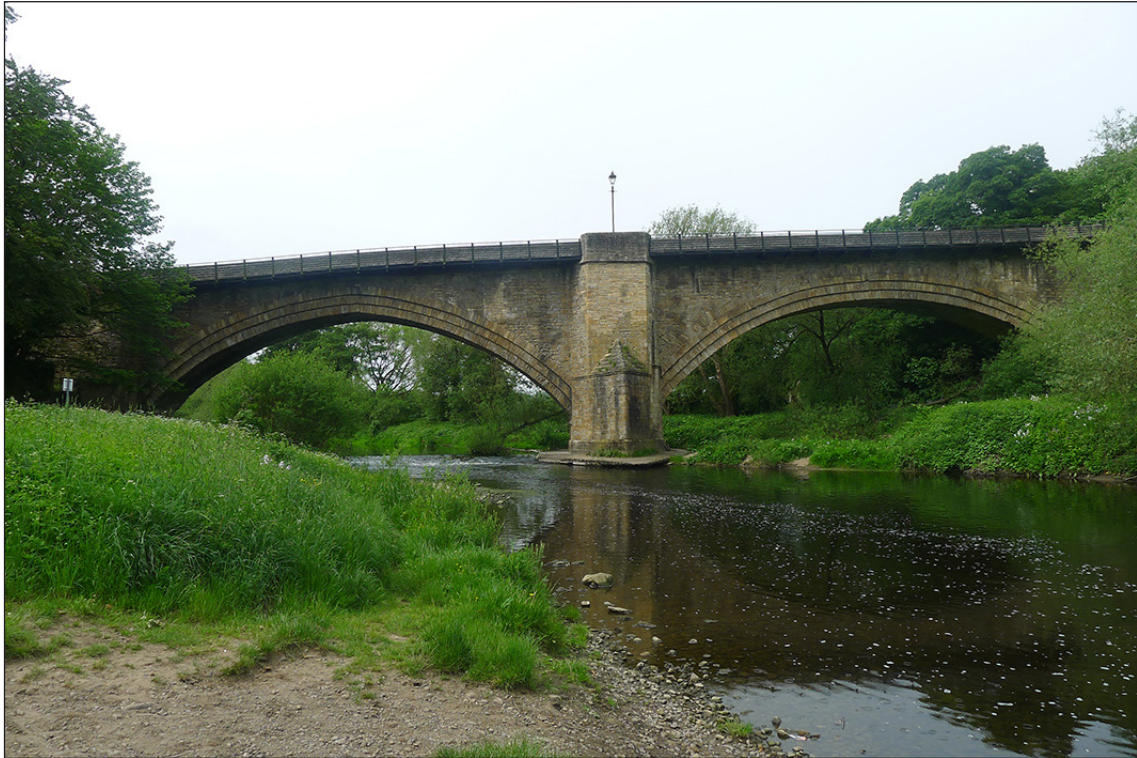
Fig 4. The eastern (downstream) elevation of Newton Cap Bridge. (© Historic England/Marcus Jecock)
