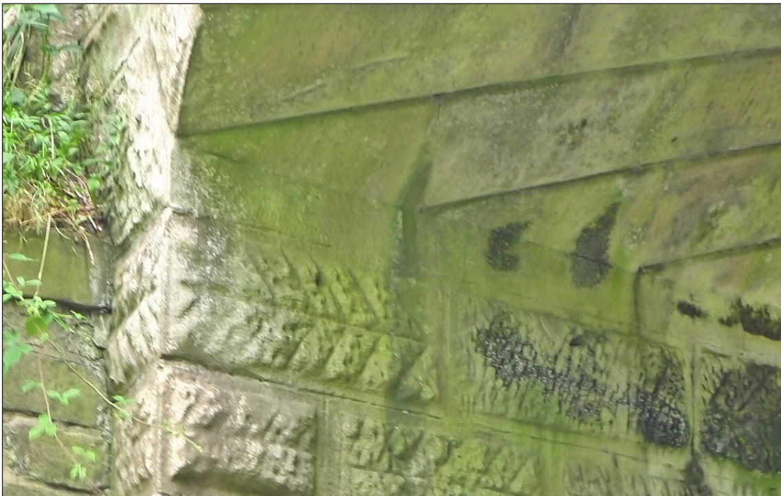
Fig 60. Detail of the arch springing on railway underbridge DAE2/7 (Bone Mill Bank). Note the stones forming the first course of the arch barrel are integral with the abutment coursing, and the distinctive way the stones of the abutment have been dressed using incised chevrons. (© Historic England/Marcus Jecock)
