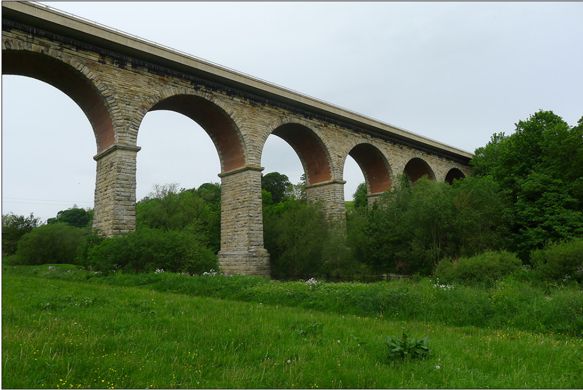
Fig 49. The northern end of Newton Cap Viaduct from the east. Note the modern cantilevered road deck. (© Historic England/Marcus Jecock)
