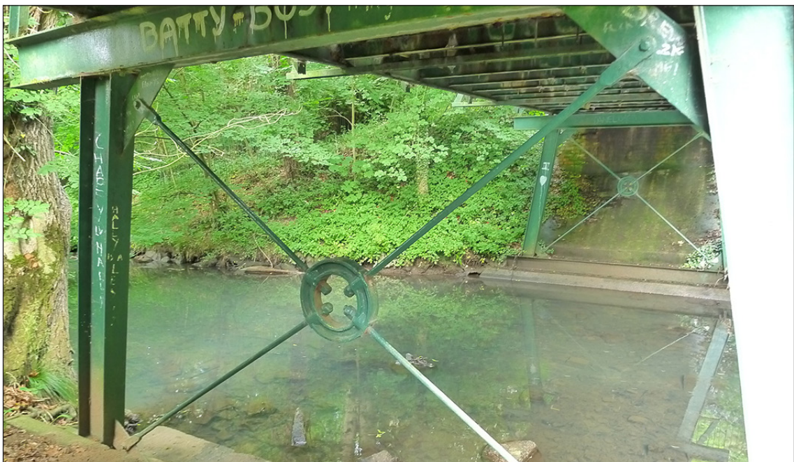
Fig 21. The support trestles to the pony truss in Bishop Auckland Cemetery (© Historic England/Marcus Jecock)
