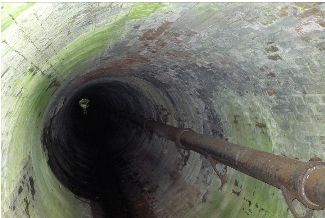
Fig 34. Interior of railway culvert BIF/8. (© Historic England/Marcus Jecock)
