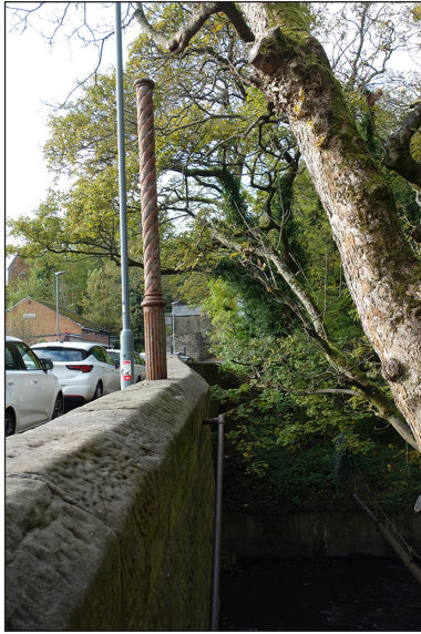
Fig 18. The cast-iron shaft of the old gas lamp on Gaunless Bridge. Note the supply pipe on the outside of the parapet. (© Historic England/Rebecca Pullen)
