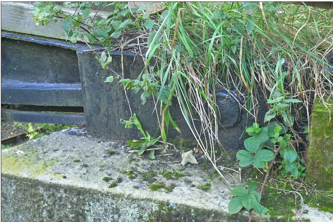
Fig 77. Detail of one of the truss hinges of railway accommodation overbridge DAE2/12 (lenticular truss). (© Historic England/Marcus Jecock)
