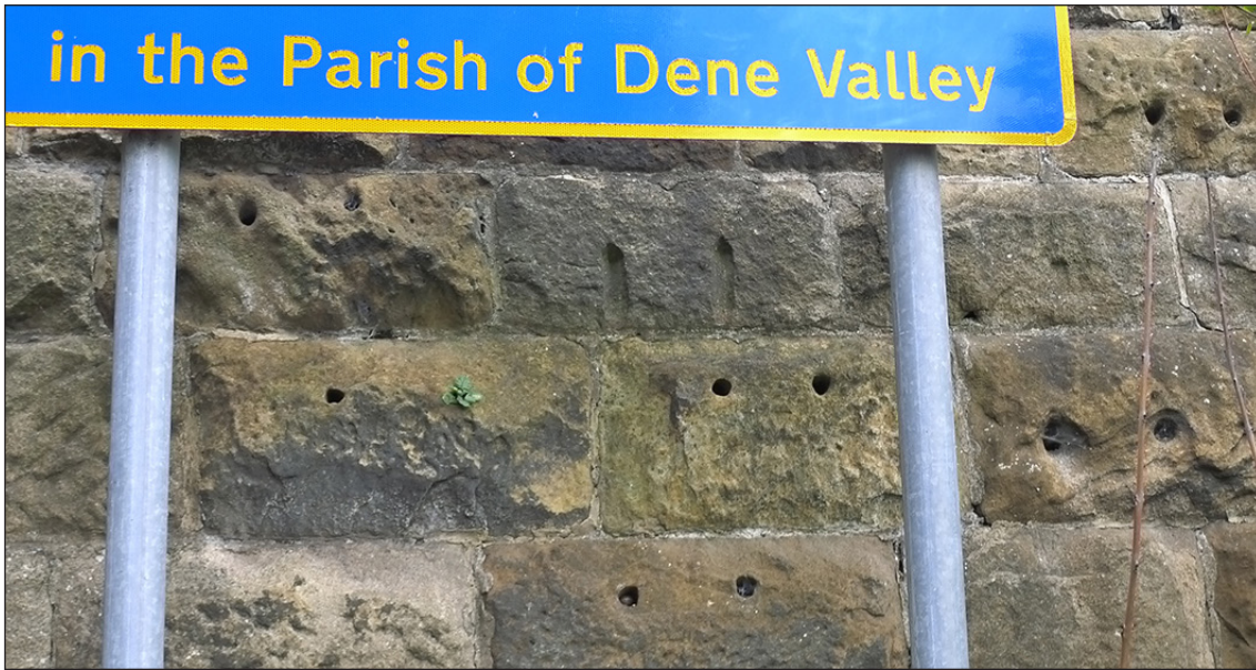
Fig 55. Detail of S&DR stone sleepers re-used in the north-east retaining wall of railway underbridge DAE2/4 (High Street, Coundon Grange). (© Historic England/Marcus Jecock)
