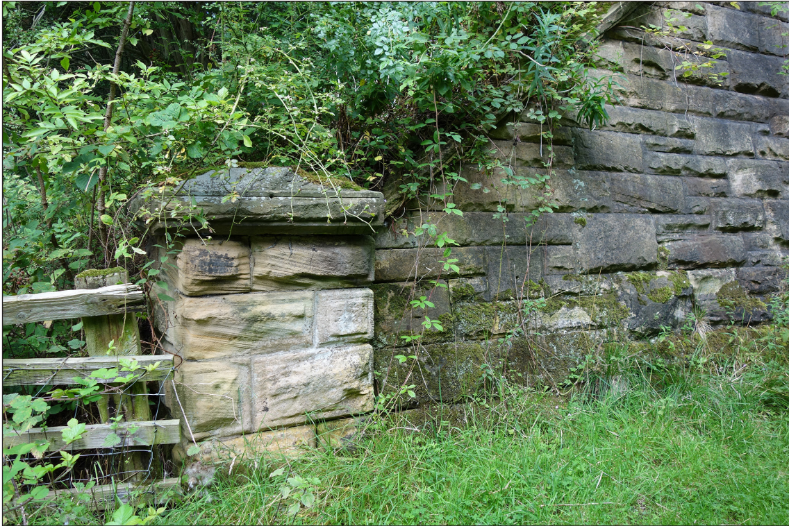
Fig 39. Detail of one of the end piers and part of the embankment retaining walling of railway accommodation bridge BIF/9. (© Historic England/Rebecca Pullen)
