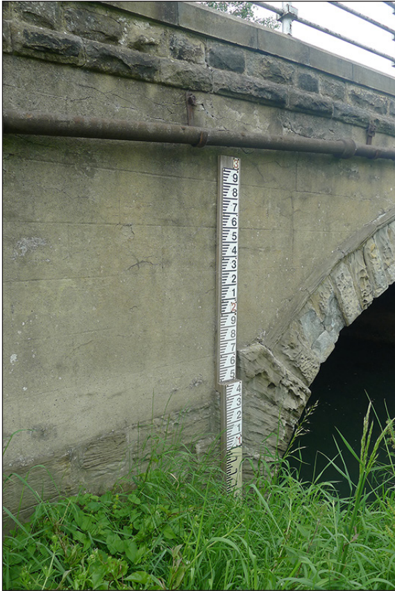
Fig 23. Detail of the western abutment of the phase-1 B6282 bridge over the River Gaunless at South Church, showing the difference in the form of the voussoirs and the exposed masonry in the causeway. (© Historic England/Marcus Jecock)
