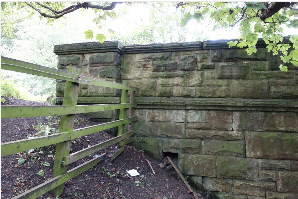
Fig 31. Detail of railway accommodation bridge BIF/7, showing string course, end pier and coping. (© Historic England/Rebecca Pullen)
