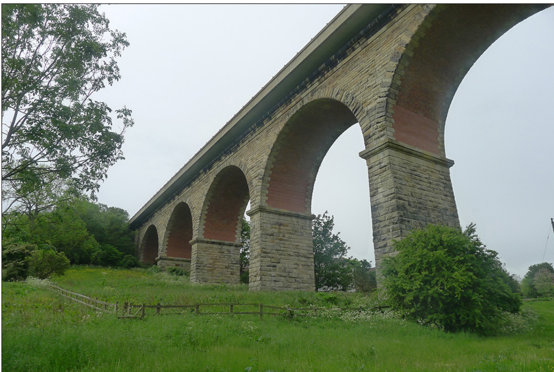
Fig 50. The southern end of Newton Cap Viaduct from the east. Note the modern cantilevered road deck. (© Historic England/Marcus Jecock)
