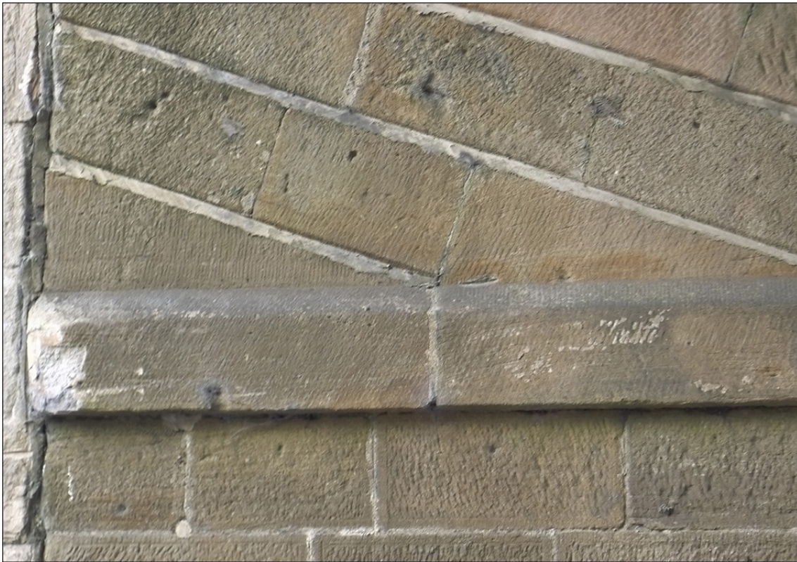
Fig 54. Detail of the impost banding and helicoidal coursing of the phase-1 arch barrel of railway underbridge DAE2/4 (High St, Coundon Grange). Note that the stones forming the first course of the barrel are integral with those in the impost banding beneath. Note also the butt joint with the masonry of the phase-2 widening just visible at left of frame. (© Historic England/Marcus Jecock)
