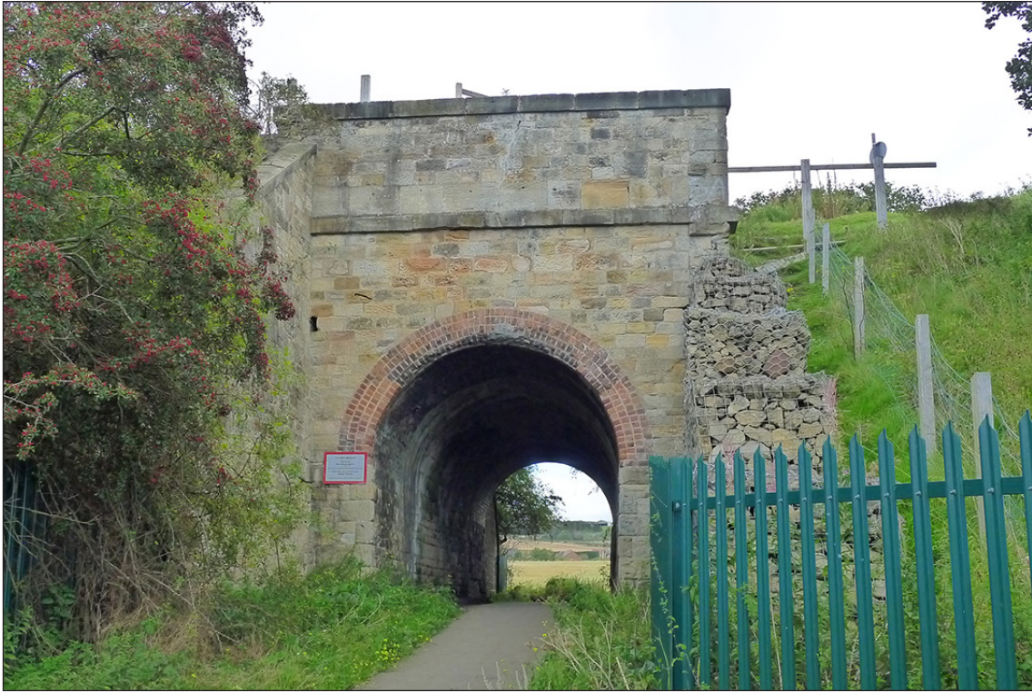
Fig 58. The western, phase-2, elevation of railway accommodation underbridge DAE2/6 ('Shepherds'). (© Historic England/Marcus Jecock)
