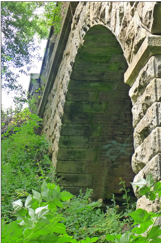
Fig 29. Detail of the western arch and parapet of railway accommodation bridge BIF/5, showing end pier, string course and impost banding. (© Historic England/Marcus Jecock)
