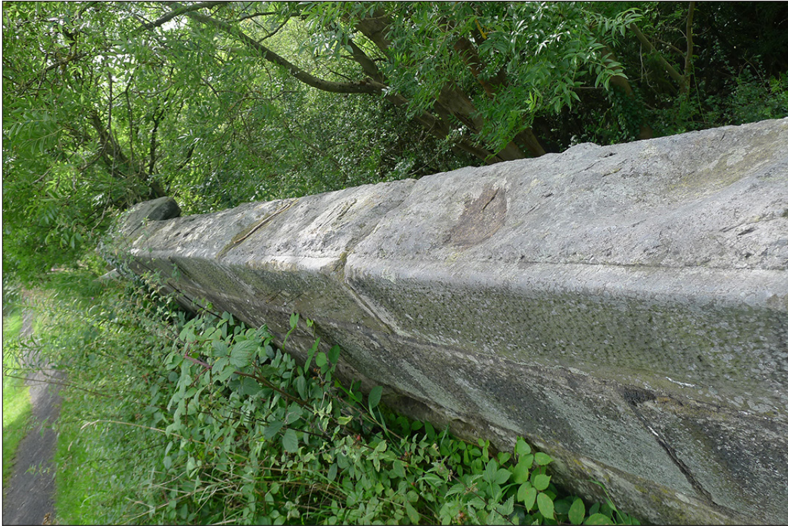
Fig 37. The (?original) eastern parapet of railway accommodation bridge BIF/9. (© Historic England/Marcus Jecock)
