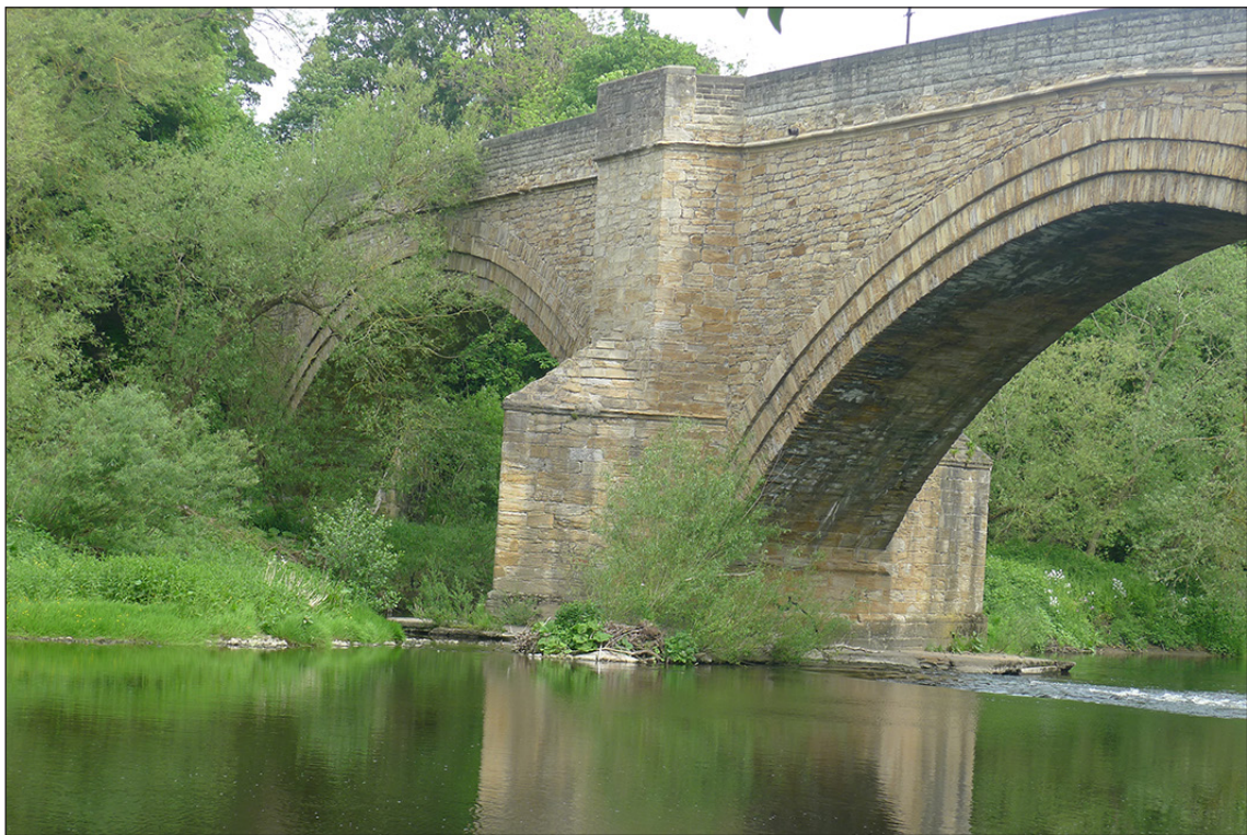
Fig 7. The western (upstream) elevation of Newton Cap Bridge. (© Historic England/Marcus Jecock)
