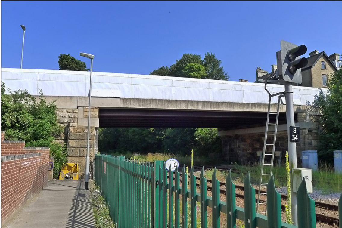
Fig 68. The west elevation of railway overbridge DAE2/10 (Cockton Hill Road). (© Historic England/Marcus Jecock)
