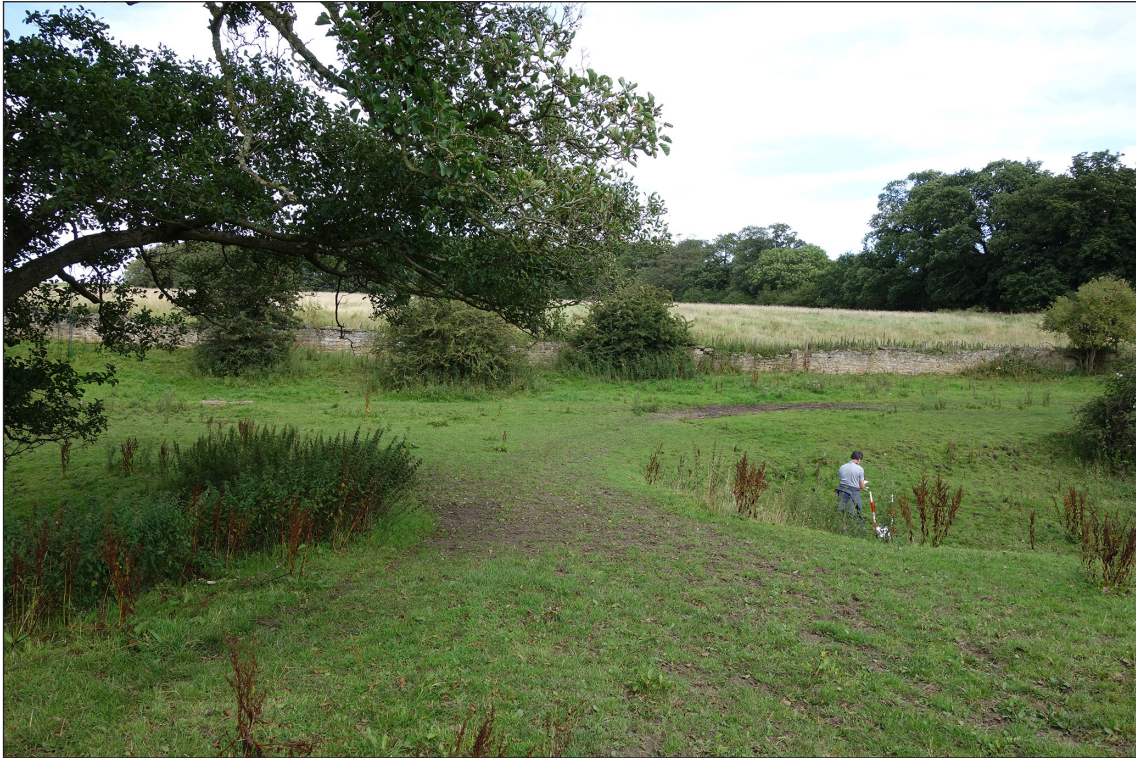
Fig 92. View south across Bishop Van Mildert's drive bridge over the Coundon Burn in Auckland Park, showing the width of the carriage drive. (© Historic England/ Rebecca Pullen)
