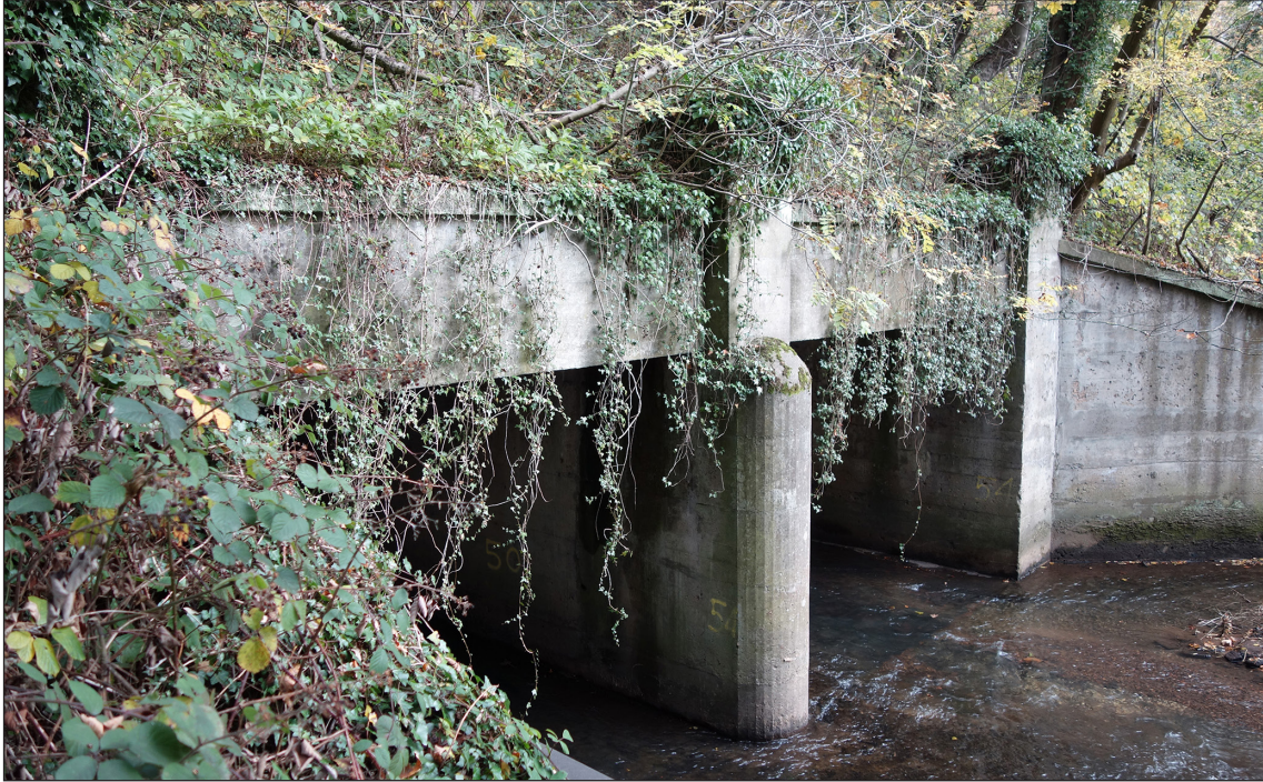
Fig 13. The southern (upstream) elevation of the bridge carrying Durham Road across the River Gaunless. Note the domed top to the bull-nose cutwater and the piers with pyramidal caps that rise through the soffit, which give the bridge a very Art Deco appearance. (© Historic England/Rebecca Pullen)
