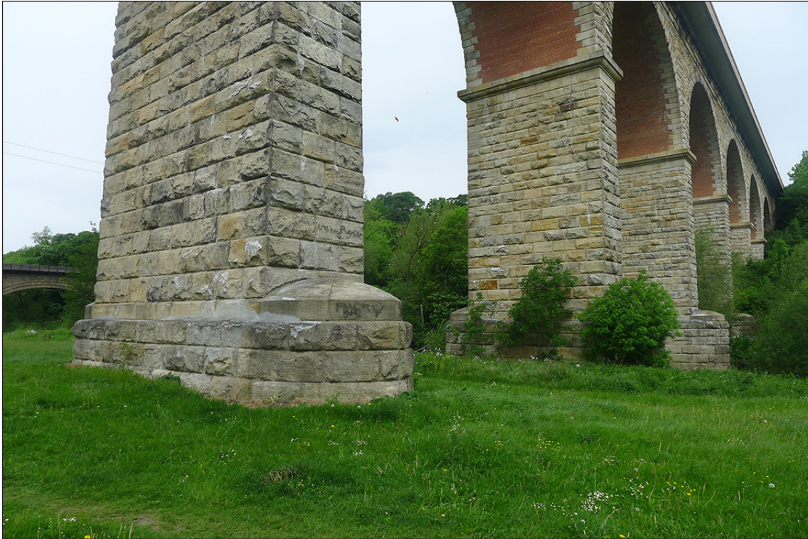
Fig 51. Detail of the cutwaters against the central piers of Newton Cap Viaduct. (© Historic England/Marcus Jecock)
