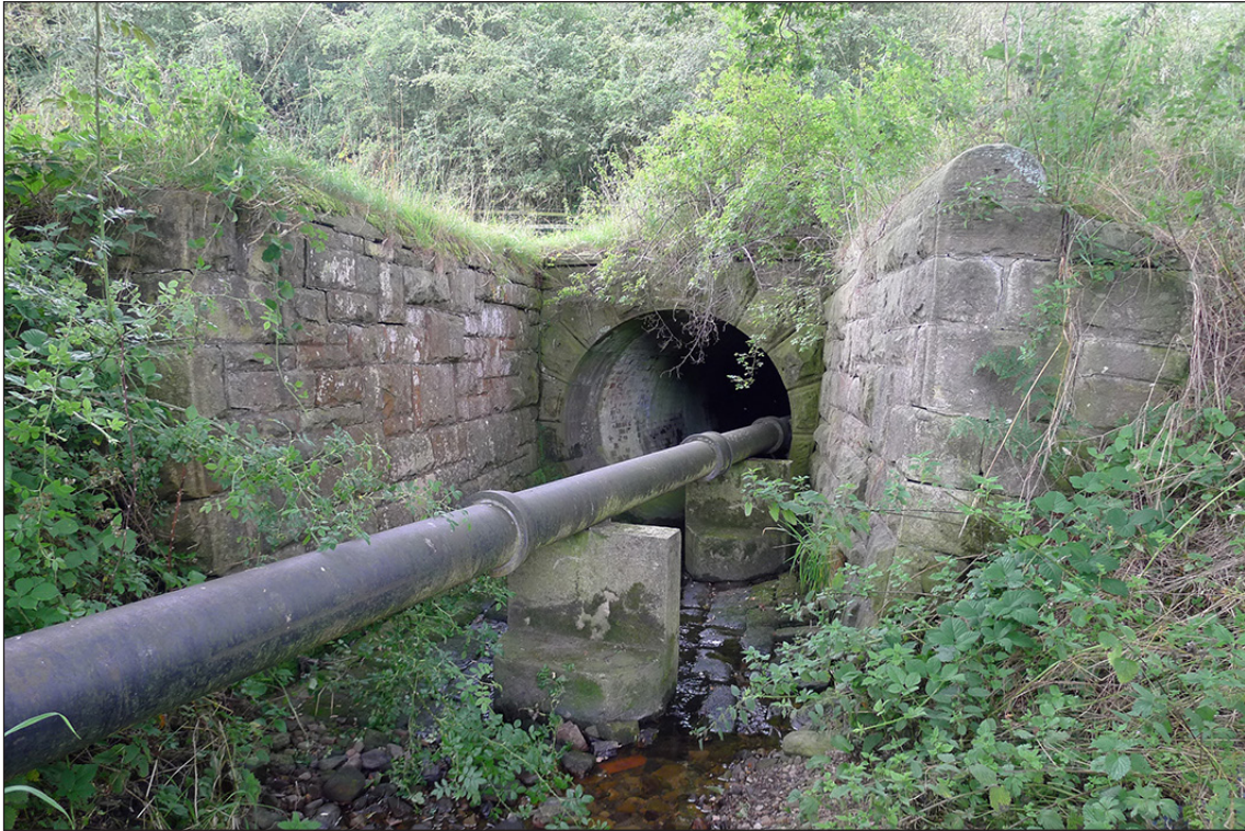
Fig 33. The eastern portal of railway culvert BIF/8. (© Historic England/Marcus Jecock)
