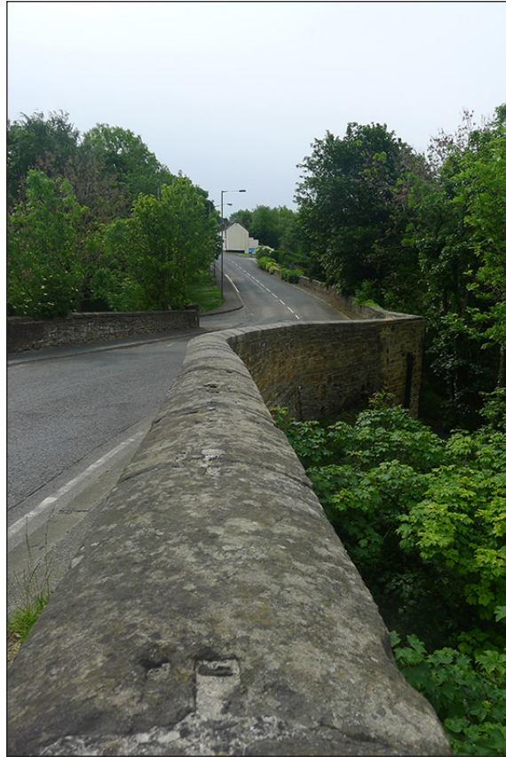
Fig 10. The northern approach to Newton Cap Bridge. (© Historic England/ Marcus Jecock)
