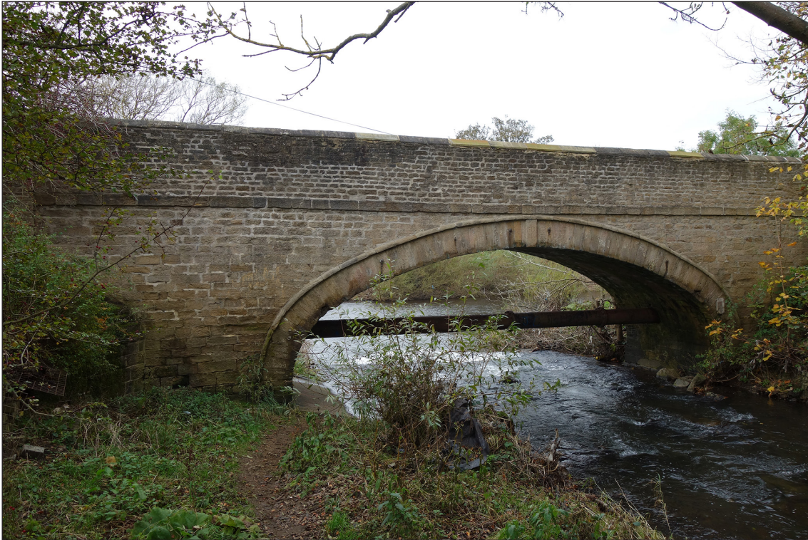
Fig 12. The eastern (upstream) elevation of Jock's Bridge. Note the horizontal string course and parapet, suggesting the elevation has been rebuilt. The date 1819 is inscribed on the keystone of this elevation . (© Historic England/Rebecca Pullen)
