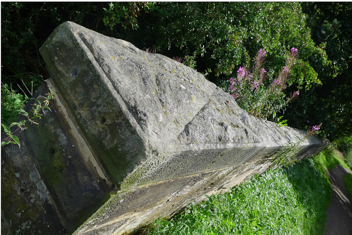
Fig 32. Detail of end pier on accommodation bridge BIF/7, showing the saltire design on the pyramidal cap and the varied treatment of 'public' and 'non-public' surfaces. (© Historic England/Marcus Jecock)
