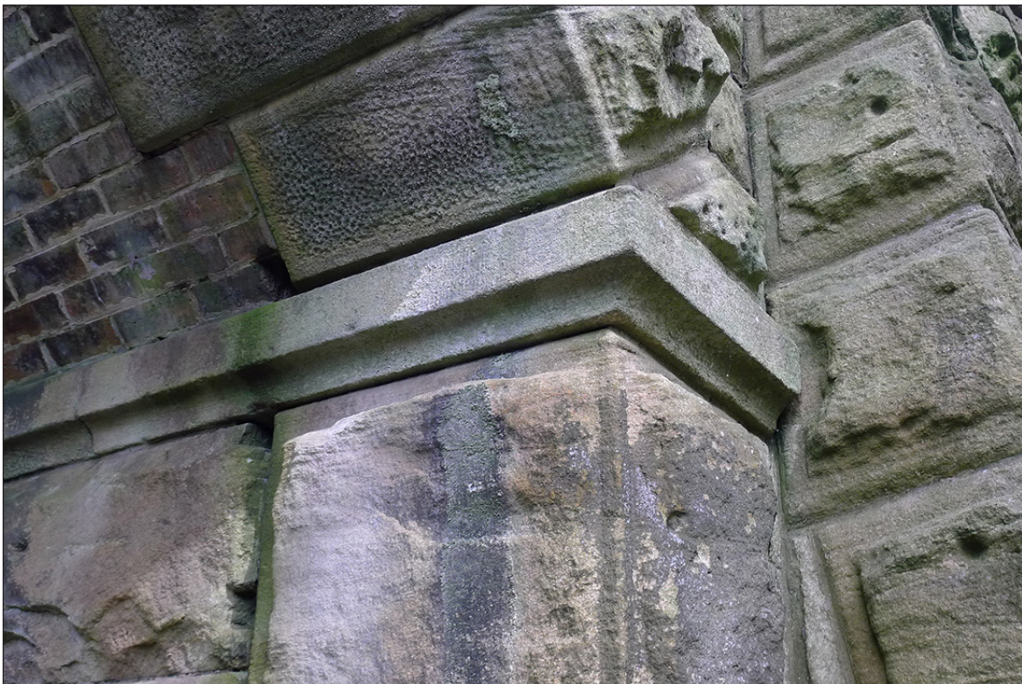
Fig 44. Detail of the springing of railway accommodation bridge BIF/11 ('Bishop's Bridge'), showing impost banding plus the varied finishes applied to the other stonework. (© Historic England/Marcus Jecock)
