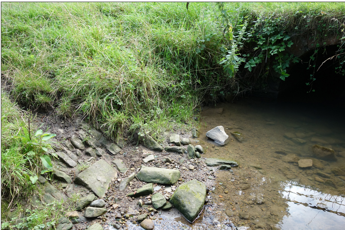
Fig 83. Detail of the paved stream bed or invert of an earlier bridge site immediately downstream of 'Bishop Trevor's' culvert for the Coundon Burn in Auckland Park. (© Historic England/Rebecca Pullen)
