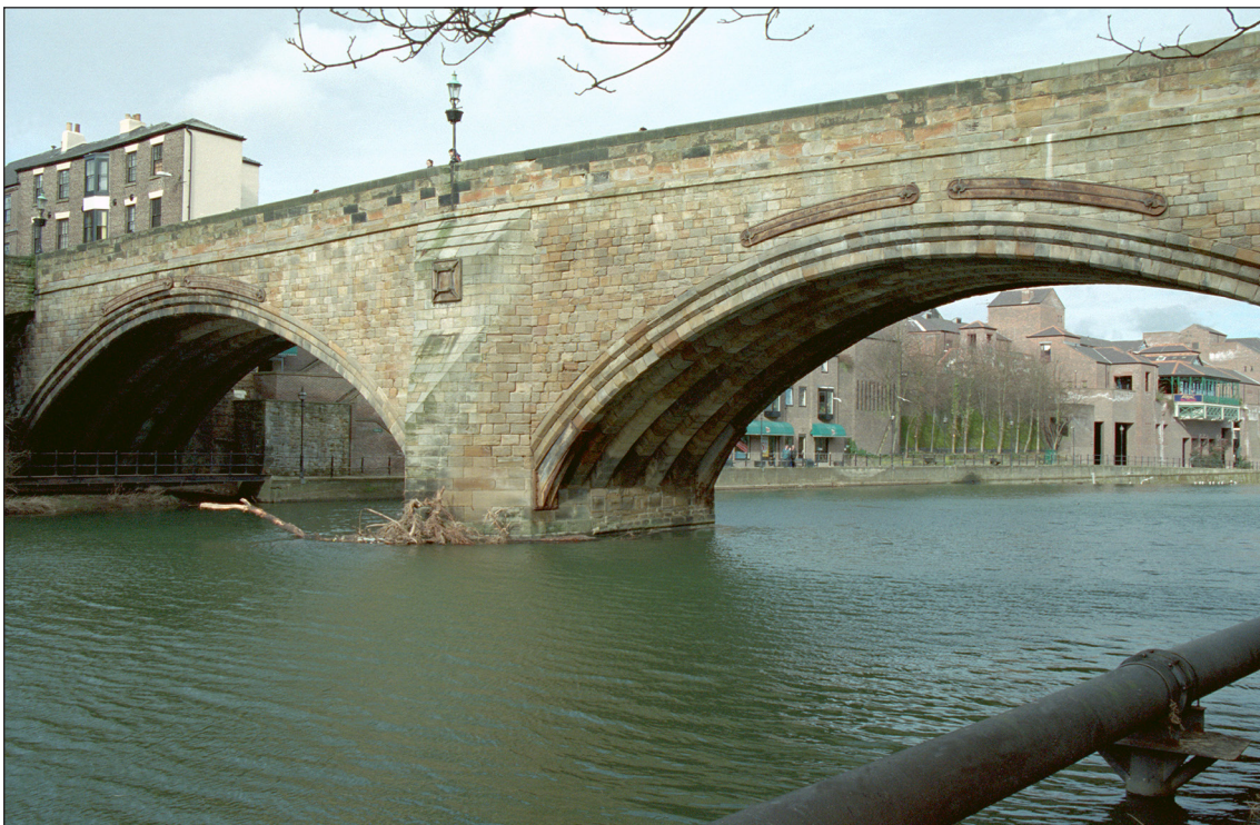
Fig 2. Framwellgate Bridge, Durham. Note the triple arch rings visible on the elevation, with the first ring made up of a series of discrete ribs (visible under the soffit of the arch). © Mr Bob Cottrell. Source: Historic England Archive IOE01_03605_35
