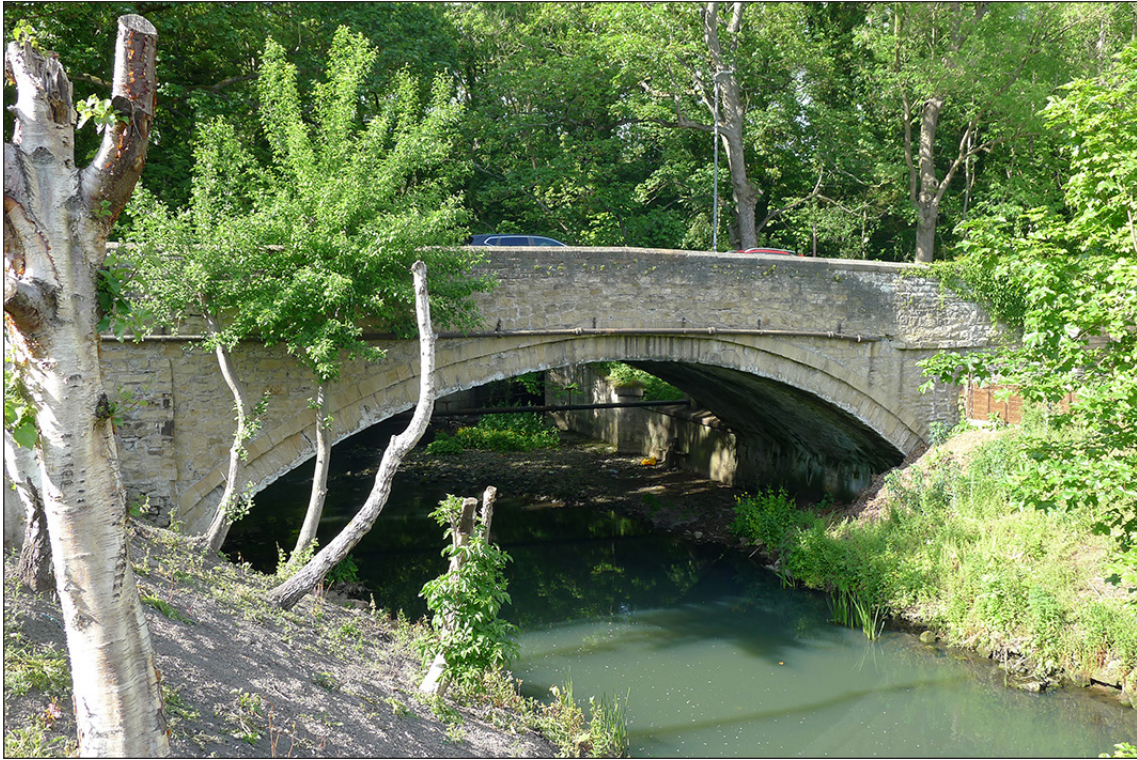
Fig 16. The southern (upstream) elevation of the phase-1 Gaunless Bridge. (© Historic England/Marcus Jecock)
