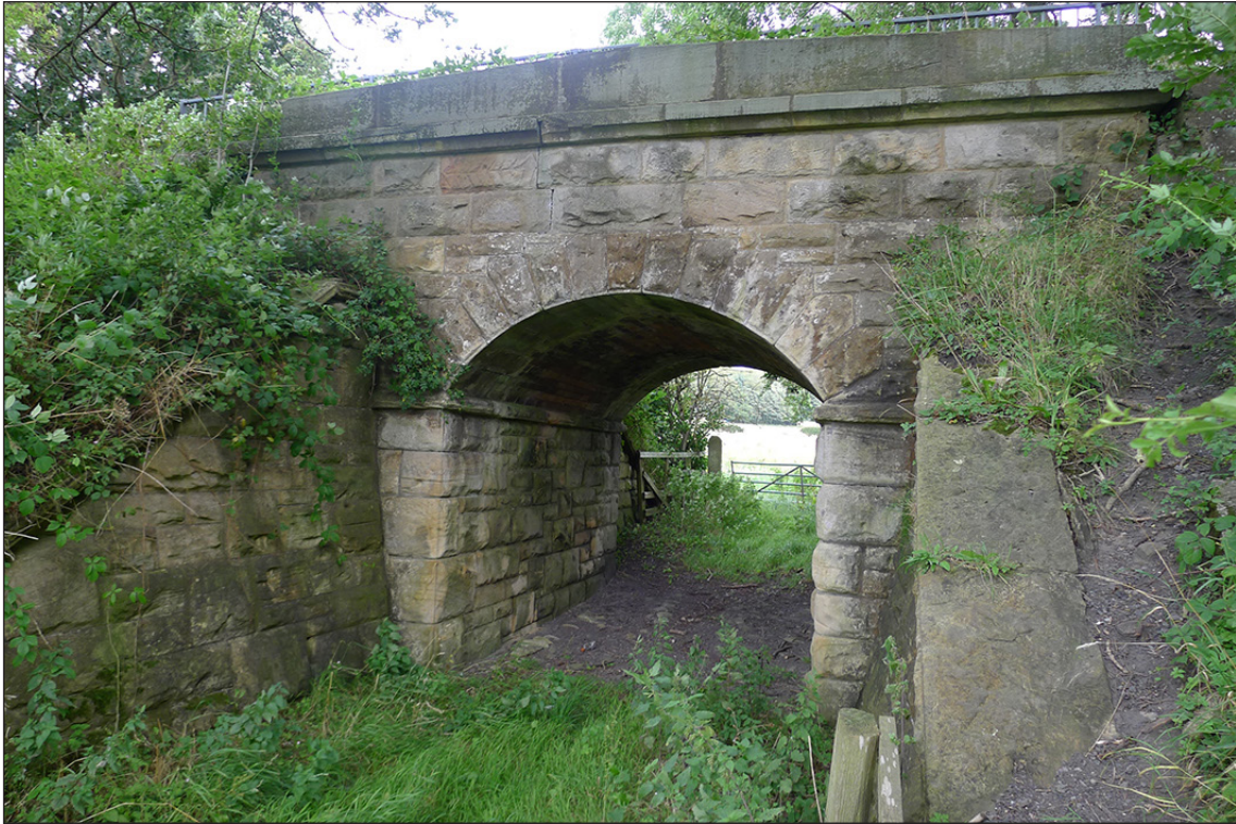
Fig 40. West elevation of railway accommodation bridge BIF/10. (© Historic England/Marcus Jecock)
