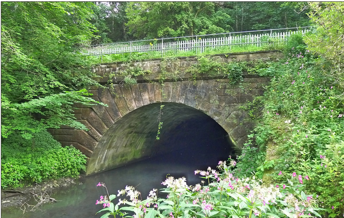
Fig 64. The northern portal of railway bridge DAE2/8 over the River Gaunless. Note the low parapet wall above the coping, probably added before 1896 to retain extra embankment material when the railway was widened. (© Historic England/Marcus Jecock)
