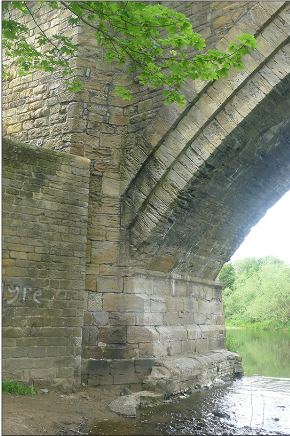
Fig 9. The face of the southern abutment of Newton Cap Bridge. (© Historic England/Marcus Jecock)
