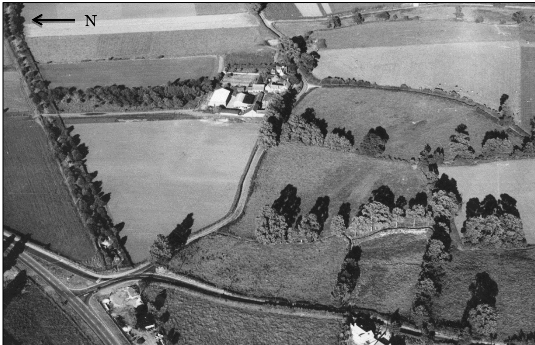
Figure 68 Linear earthworks (MDO41036) to the west of Lake Farm, Pamphill; the site of an early 1st century AD Roman fort (MDO5864).
