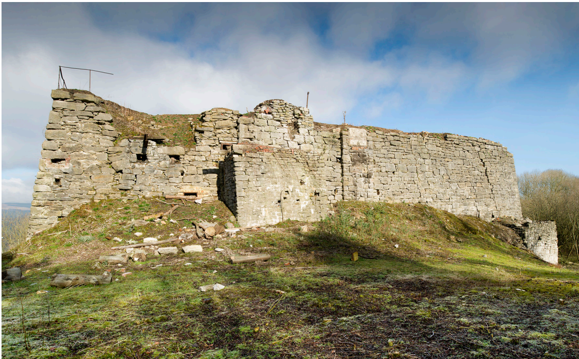
Fig 4. Bellmanpark kiln block from the south. Note the bridge abutment with its massive stone bearing block just right of centre of frame, and the various wall boxes and apertures towards the west end of the block (above and right of the off-centre stone projection). (Photograph: DP169492 © Historic England / Alun Bull, 24 February 2016).
