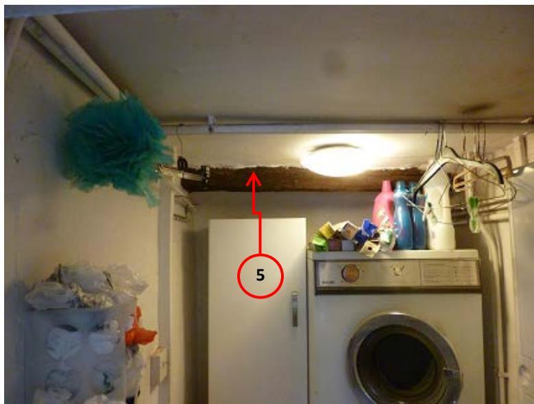
Figure 4c/d: Plan of unit B (top) (after building survey team) and annotated photograph of unit A looking south (bottom) (photograph Robert Howard) to help locate sampled timbers
