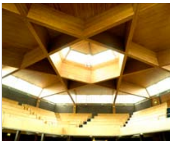
Fig. 59 Beth Hamedrash Hagadol, ceiling detail. © English Heritage NMR DP034091
