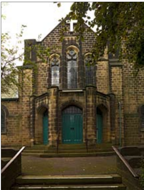
Fig. 36 Lidgett Park Methodist Church. © English Heritage NMR DP028537
