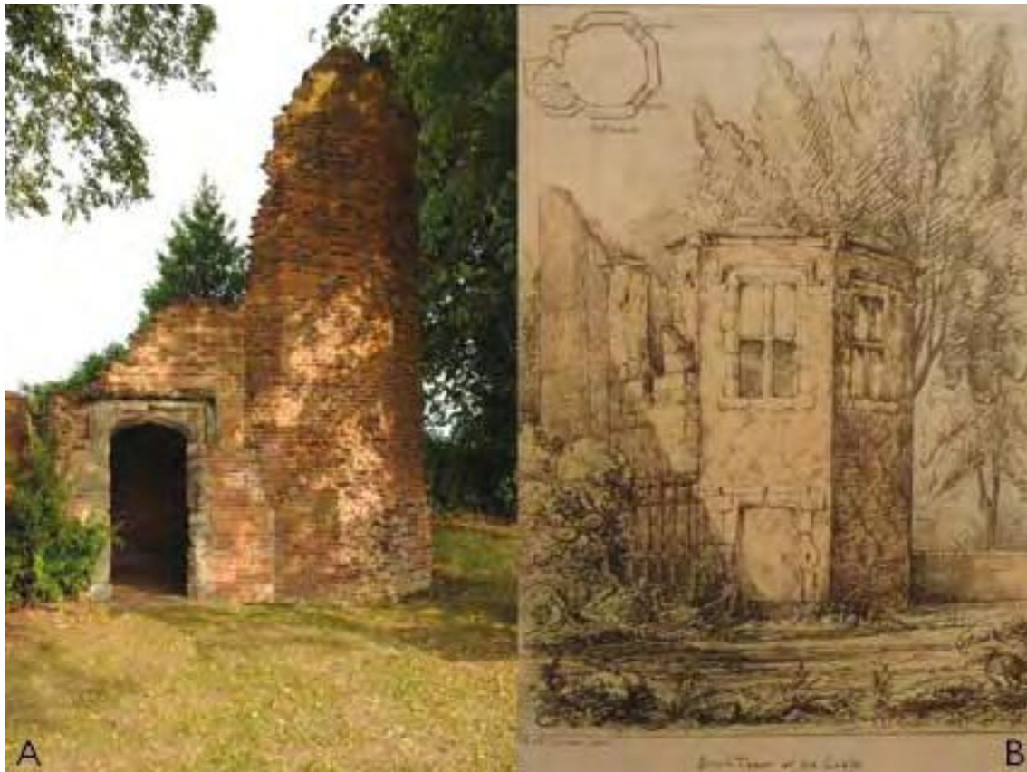
Figure 28: Eastern garden building. A – North-west elevation. B - 1855 sketch of eastern elevation by MAE Vavasour (Reproduced with the kind permission of Ashby Museum.)
