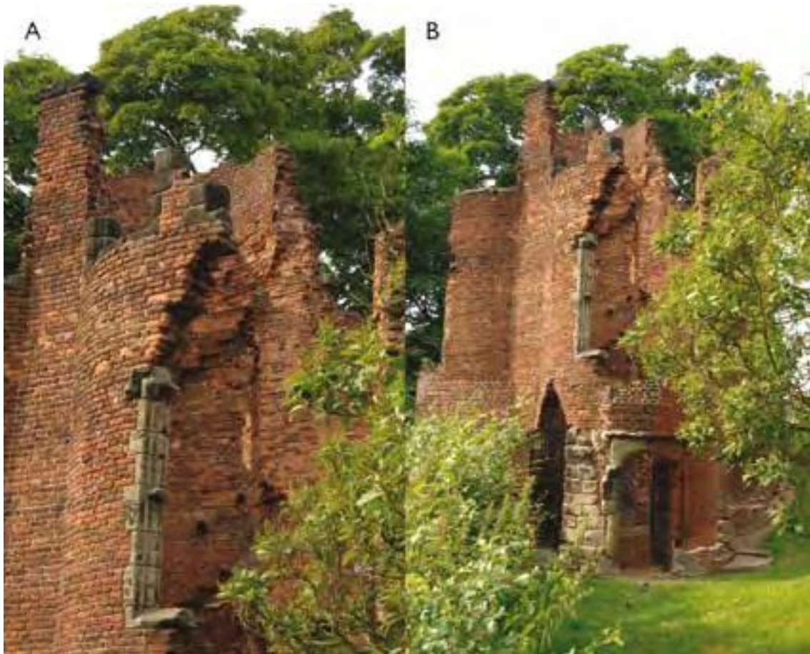
Figure 27: Western garden building. A - Window detail. B - Reconstructed south face.
