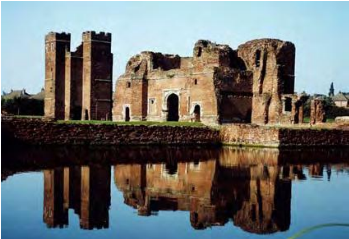
Figure 4: The unfinished remains of William, Lord Hastings' complete rebuild of the family seat at Kirby Muxloe.
