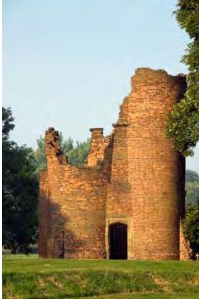
Figure 26: The western garden building.
