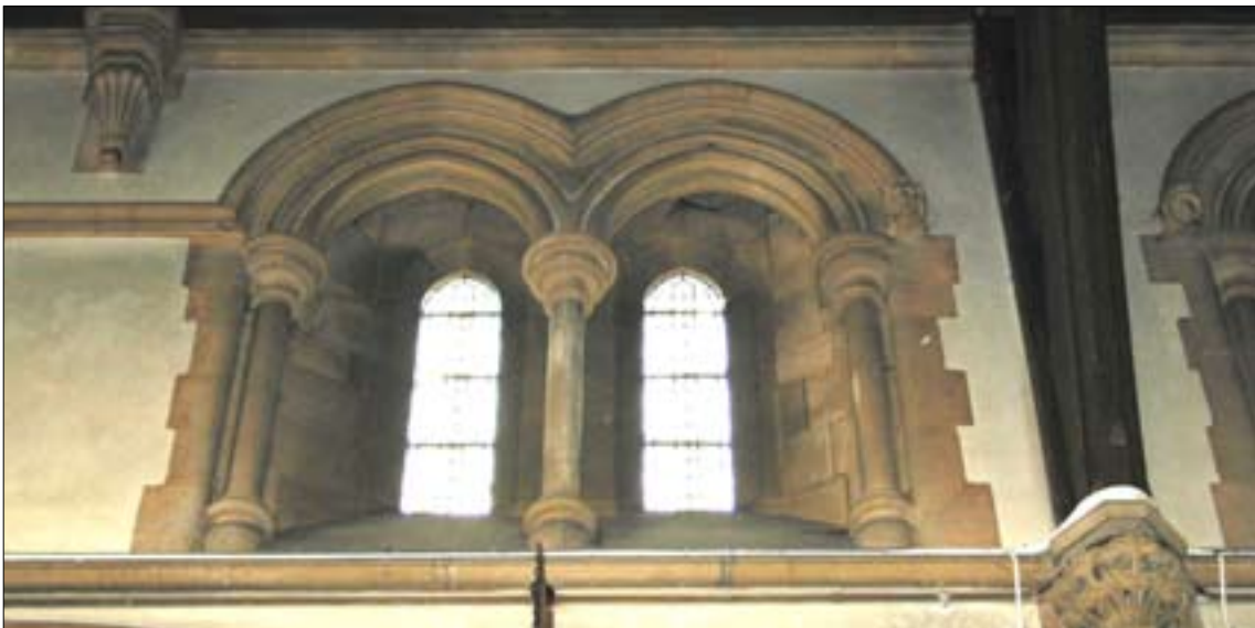
Fig. 10. Clerestory windows showing scoinson arch.
