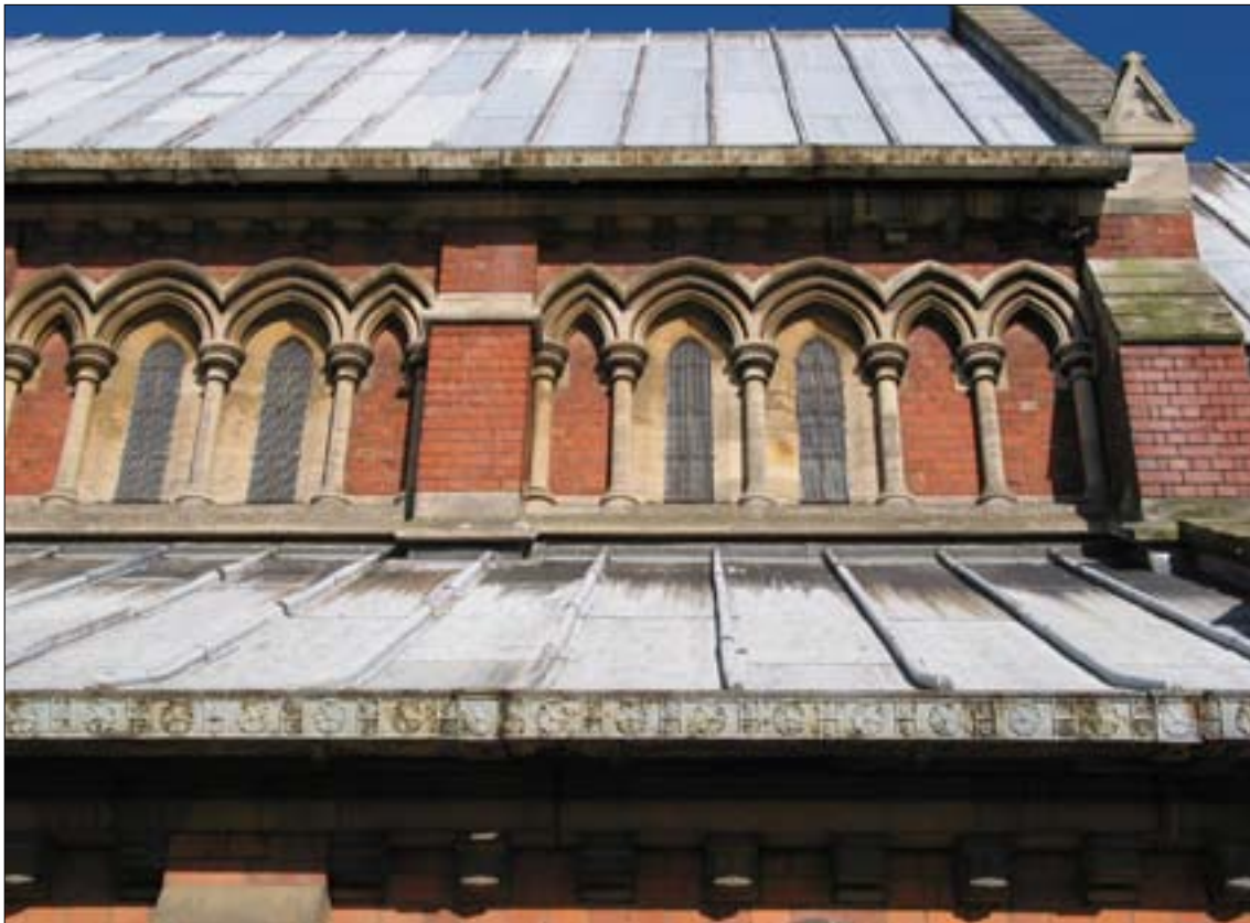
Fig. 4. Clerestory arcading and cast iron guttering.
