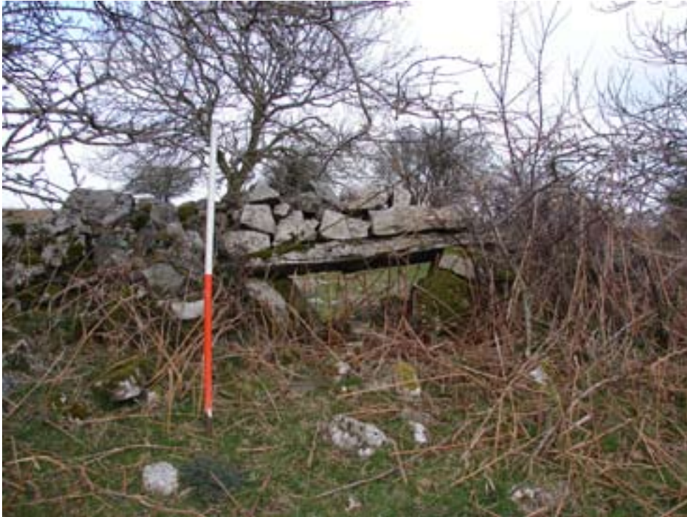
Figure 9 Sheep creep in the southern enclosure wall at Andrews Green.
