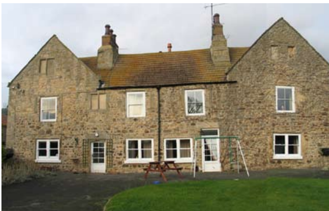
Figure 9: The south façade of Ulnaby Hall
