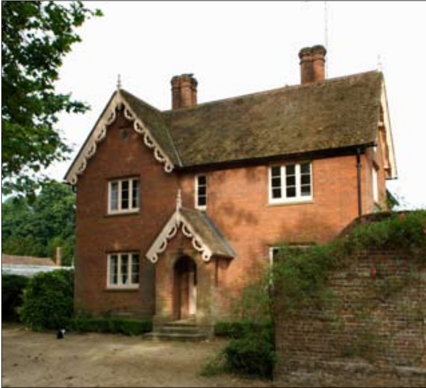
Fig. 40. The head gardener's house, probably designed by Richard Hussey in 1875.
