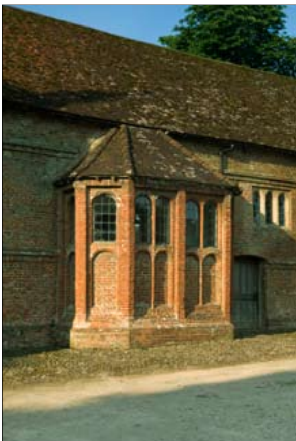
Fig. 7. The east bay window on the north front of the stable building, probably added c.1620. © English Heritage DP029955
