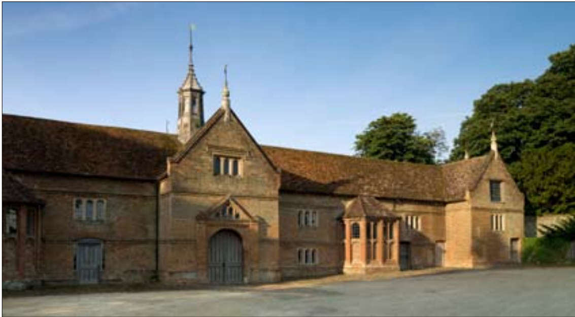
Fig. 2. The north front of the stable building.
