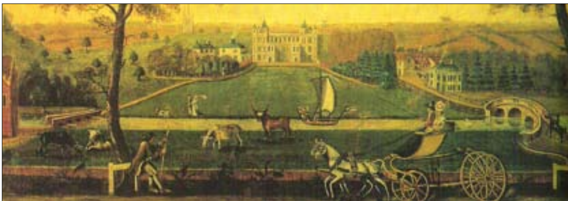
Fig. 32. Anon. Audley End from the west c.1780. This painting shows the stable building (far left) with the crenellated gables added by John Hobcroft, and Lord and Lady Braybrooke in a 'crane-necked' pheaton (right). Stanley Falconer
