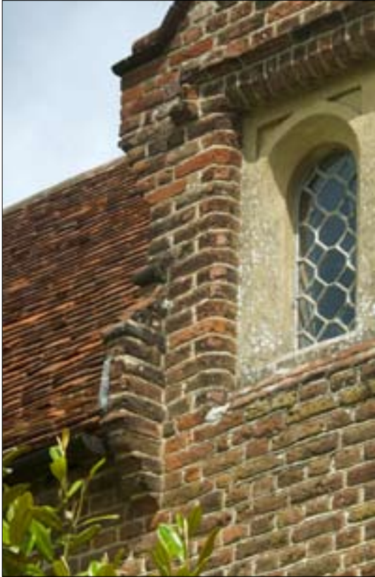
Fig. 5. One of the unusual moulded brick kneelers flanking the dormer windows on the south front.
