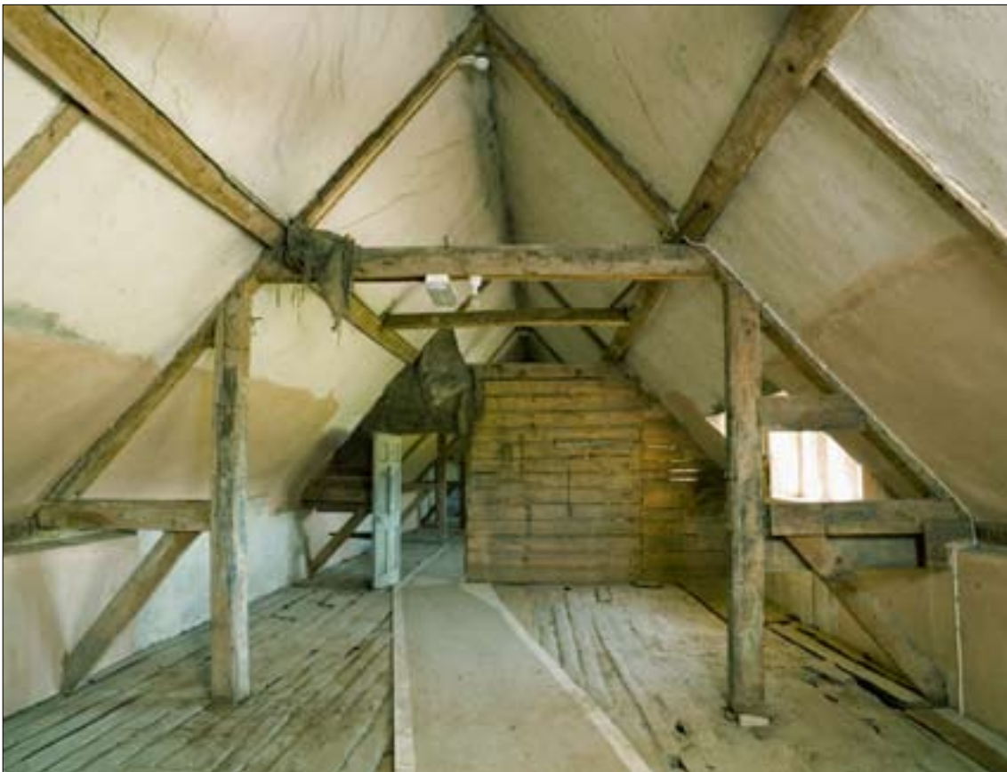
Fig. 19. The roof structure of the stable building.
