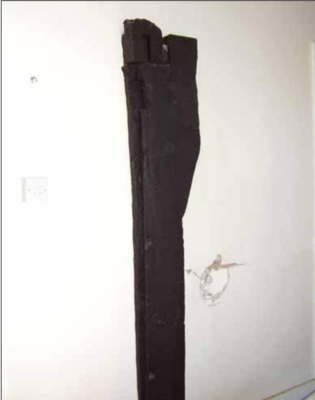
Figure 2: The east post exposed at first-floor level.
