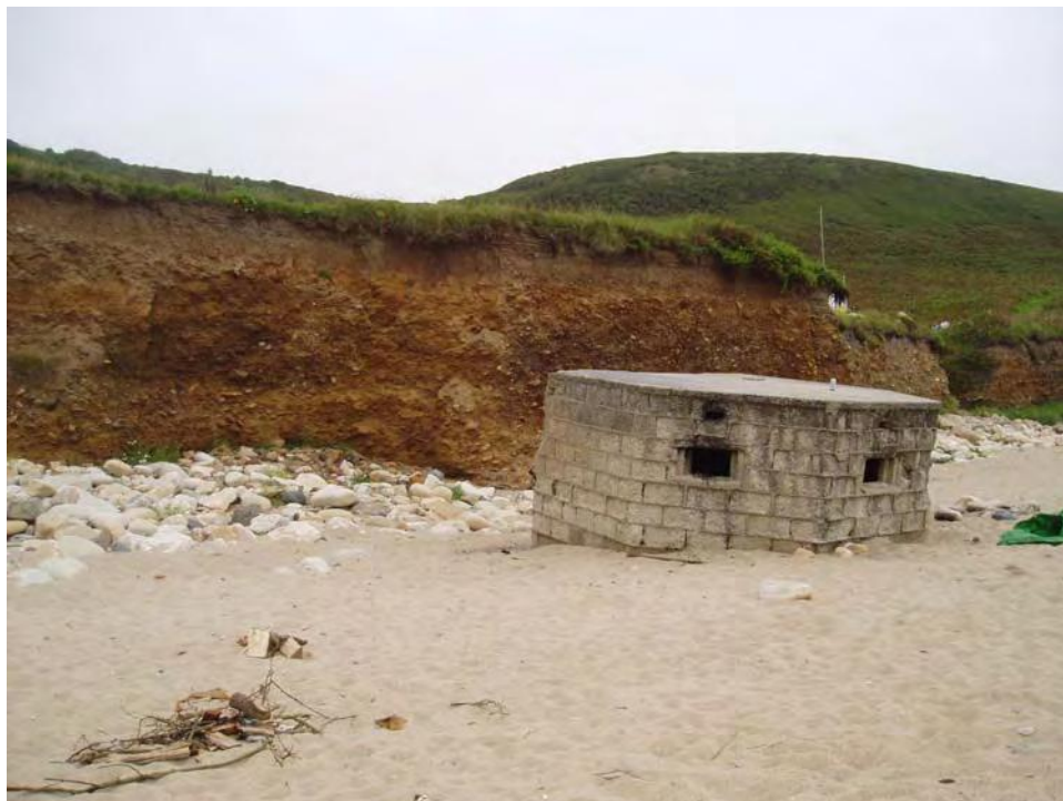
Figure 37: Prah Sands pillbox originally erected in dunes, now on the beach as the result of coastal erosion
