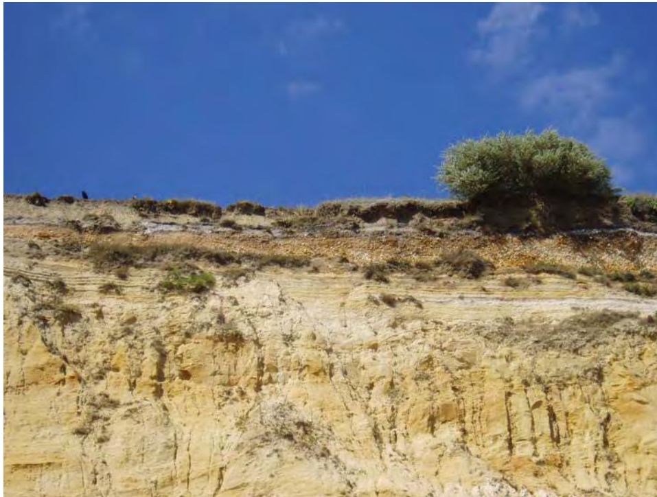
Figure 40: Branksome Chine, Bournemouth, Tertiary Beds overlain by what from the beach appear to be Pleistocene flint gravel, a podsol and the possible blown sand
