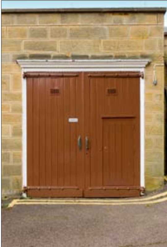
Figure 9 The doors to garage 2, showing the ventilators installed.
