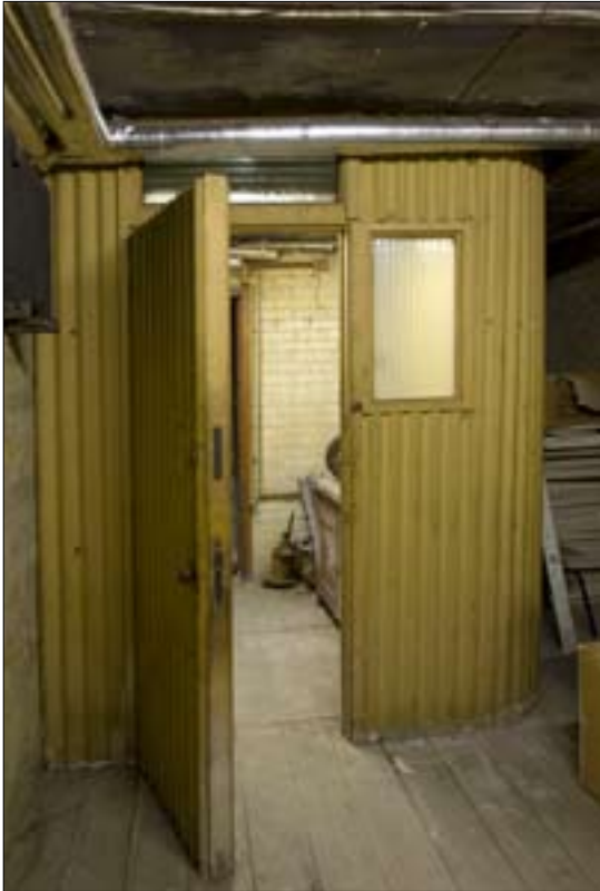
Figure 13 Basement and mechanic's dressing room.
