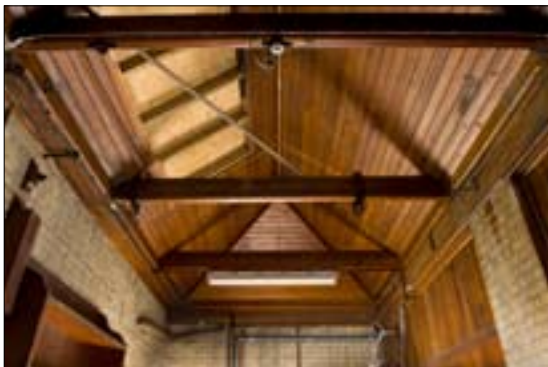
Figure 4 The roof of garage 2, showing the surviving lifting apparatus.
