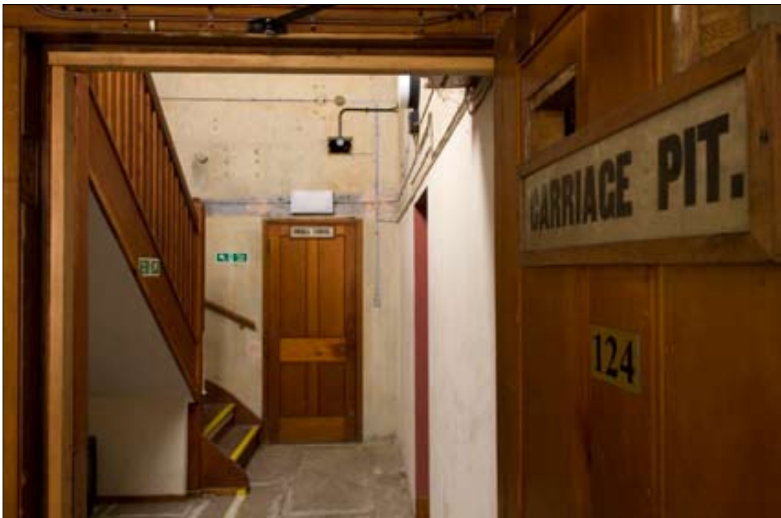
Figure 8 The basement from the inspection pit to the small forge.
