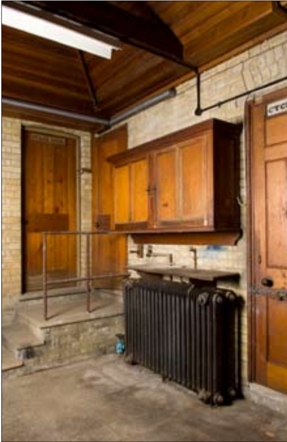
Figure 20 Cupboards for spares and central heating radiators in garage 3. Doorway to cloak cupboard to the right.
