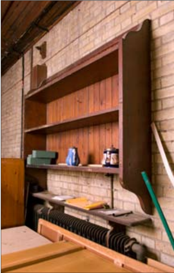
Figure 19 Shelves for spares in garage 2. © English Heritage NMR DP070055
