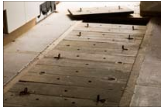
Figure 5 The removable timber boarding of the motor pits.
