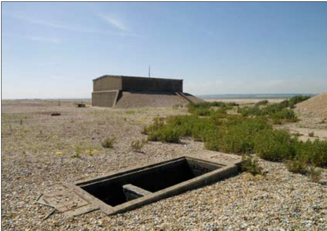
Figure 39: Centrifuge E1 to the right is one of the shingle revetted sides facing the occupied section of the site, also in view is an emergency escape way through the traverse. (C) English Heritage DP068500
