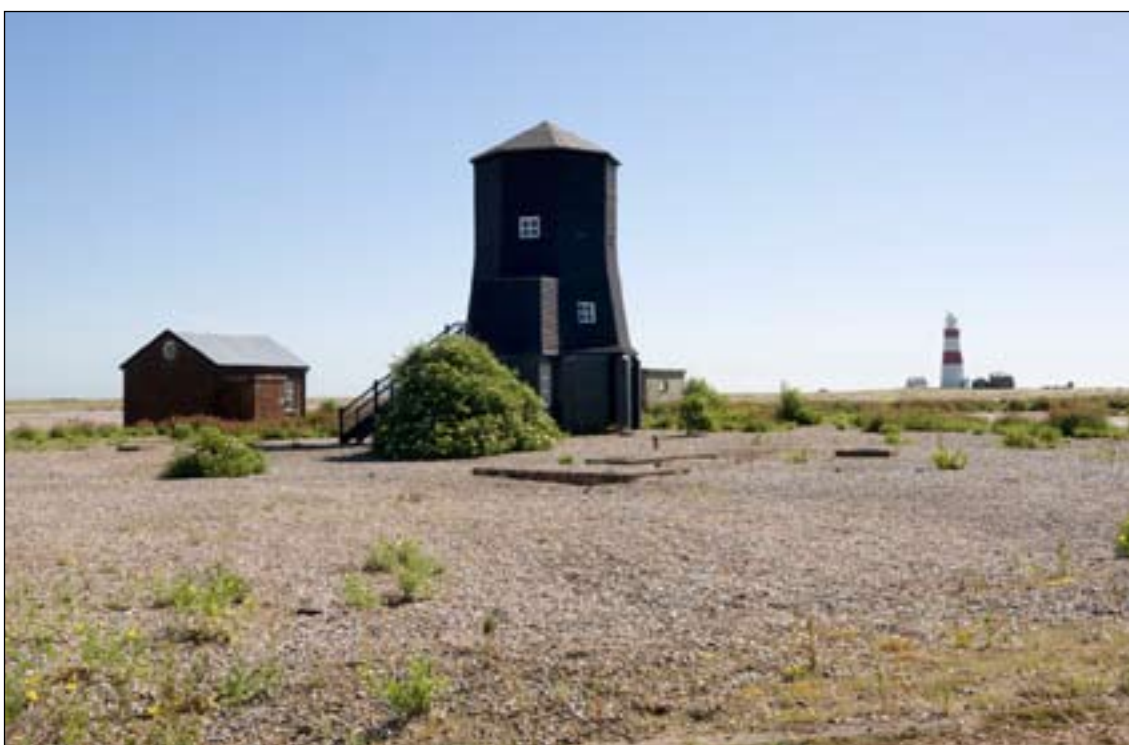
Figure 22: The Black Beacon G1/40 and to the left the Generator House G2/46. (c) English Heritage DP068424
