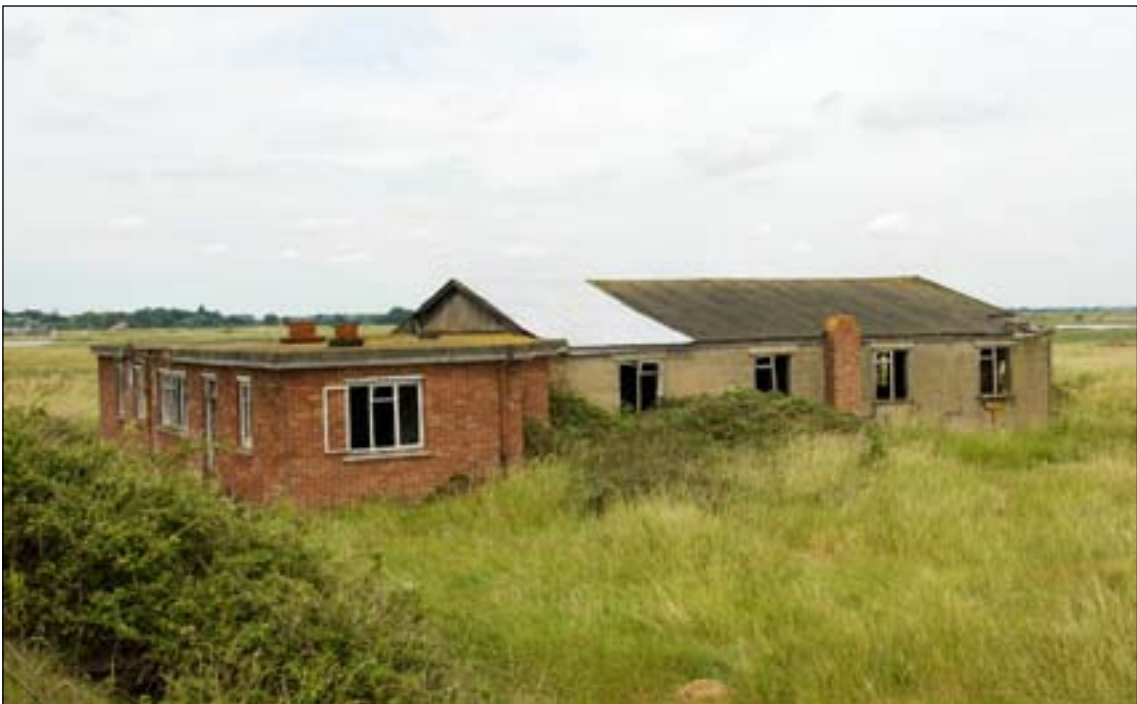
Figure 17: Building C13/3 First World War Officers' mess to right and 1950s AWRE Canteen extension to left. (c) English Heritage DP070030
