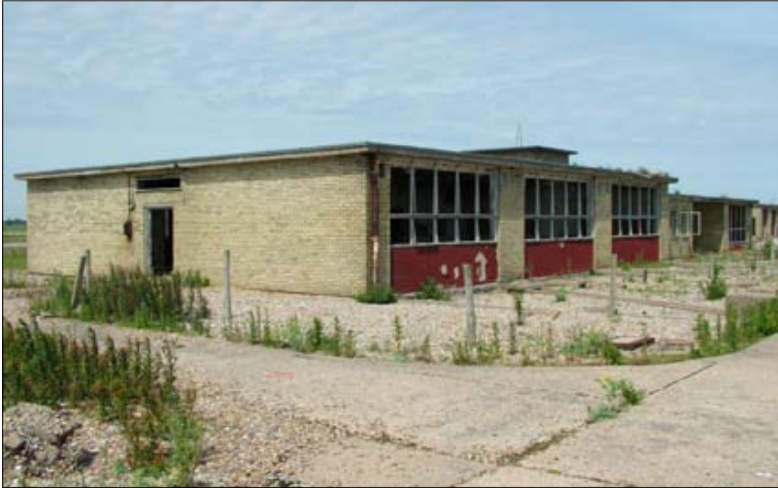
Figure 31: The Control Room E4/I39. (c) English Heritage
