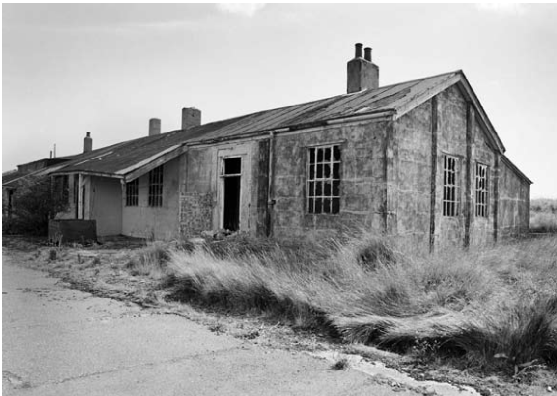
Figure 3: First World War Royal Flying Corps Headquarters building, note the use of cement block construction. This view was taken in the 1990s, it has since been demolished. (c) English Heritage AA99/08438
