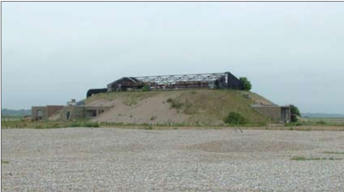
Figure 29: Laboratory 1, F3/123, to the left is the rear plant room and to the right the main entrance passage. (c) English Heritage
