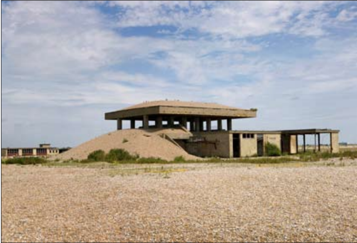
Figure 34: Vibration Laboratory E2, to the right are plant rooms. To the rear is the Control Room E4. (c) English Heritage DP0685509
