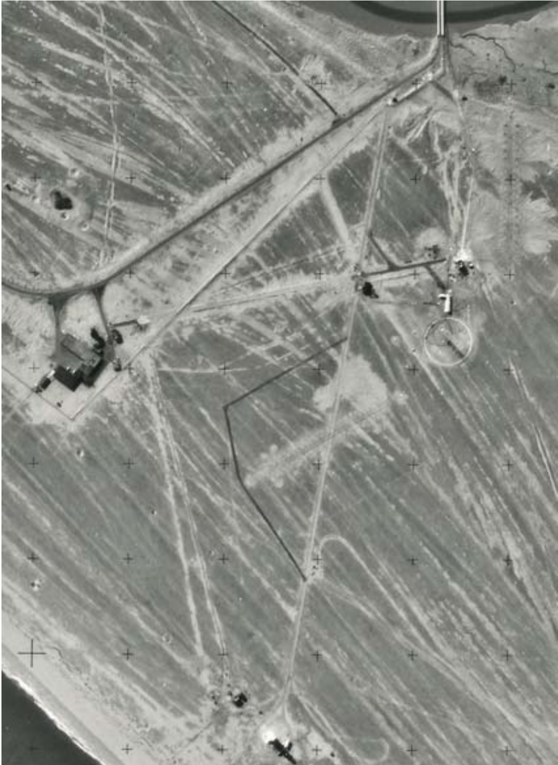
Figure 24: View of the area to the east of the AWRE boundary fence, showing to the top the circular Antenna base H50 and linear arrays to its north and south. The dark section of track marks where it has been diverted around one of the arrays. OS/65054 V029 30 April 1965 (c) Crown Copyright. Ordnance Survey
