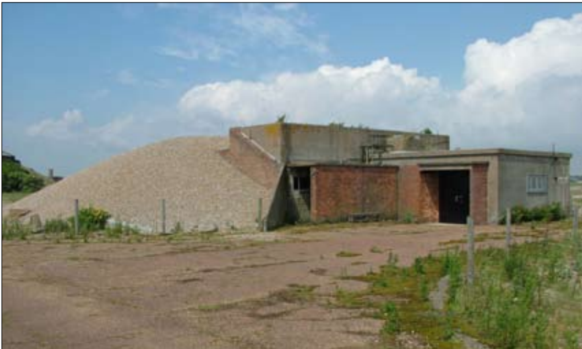
Figure 26: Control Room F4 127/67, showing the later brick porch and blast wall. (c) English Heritage
