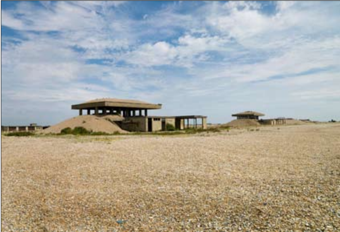
Figure 11: Vibration Test Buildings E2 and E3, or Pagodas, they were built about 1960 (c) English Heritage DP068510
