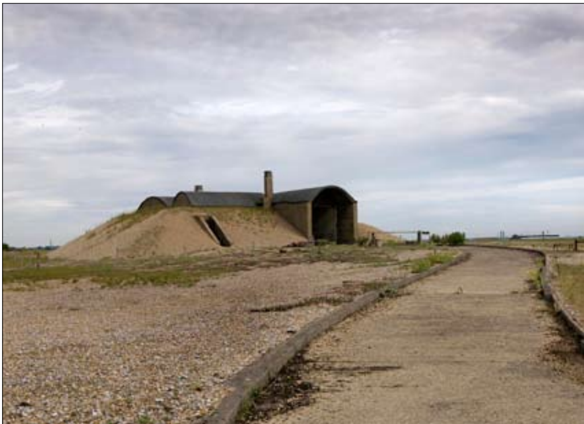
Figure 36: The Magazine E5, to the left is the door to the plant room. (c) English Heritage DP068522
