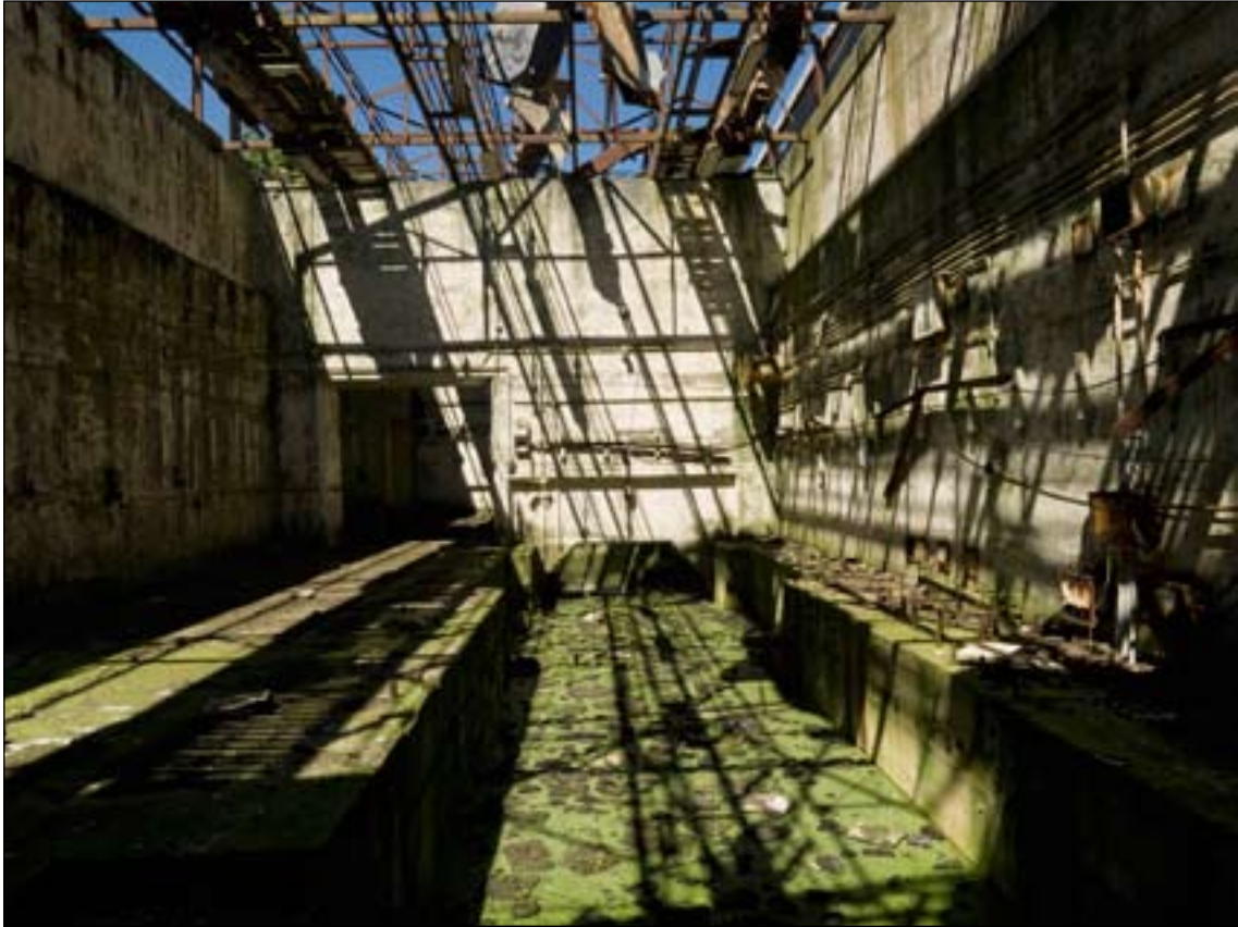
Figure 25: Laboratory I F3/I23 showing the large vibration laboratory to the southeast of the main dividing wall. (c) English Heritage DP068442
