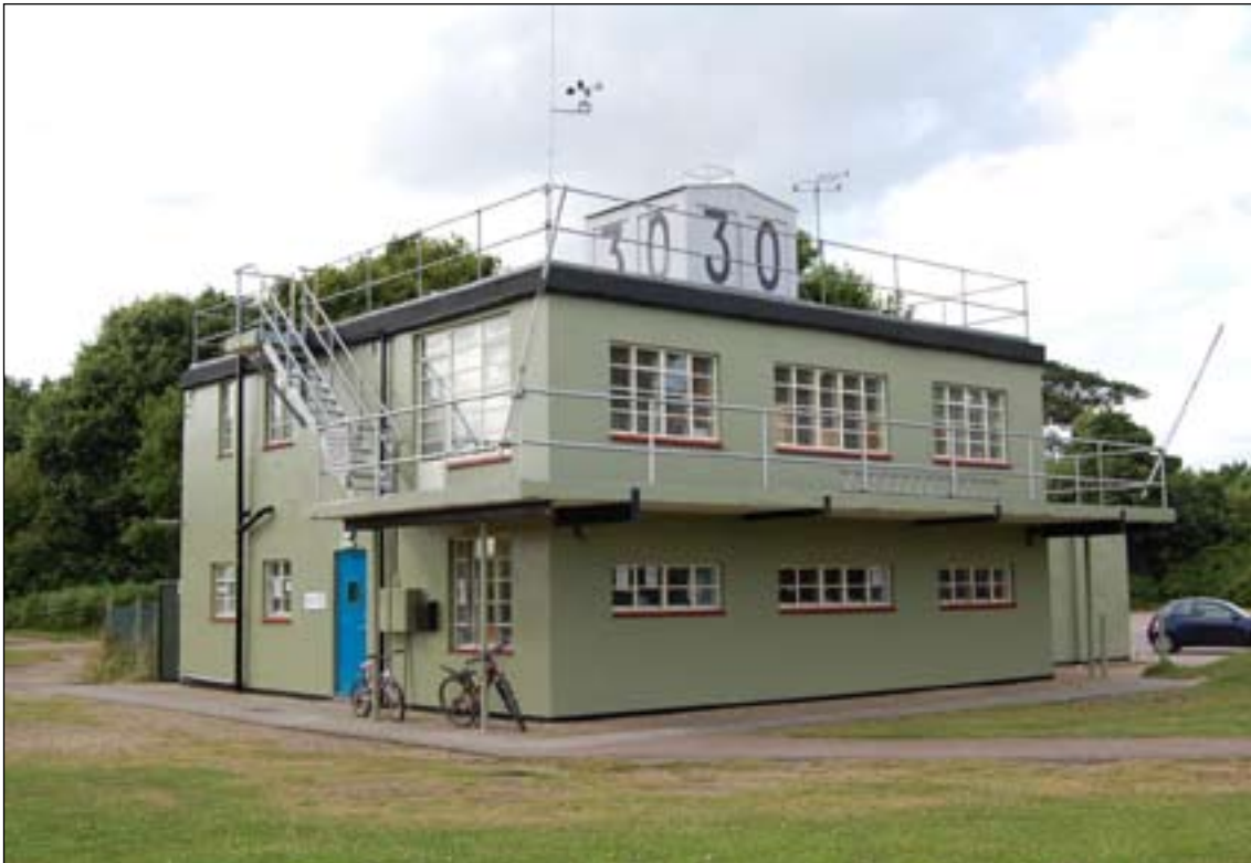
Figure 5: Former RAF Martlesham Heath, preserved Air Traffic Control tower (c) English Heritage
