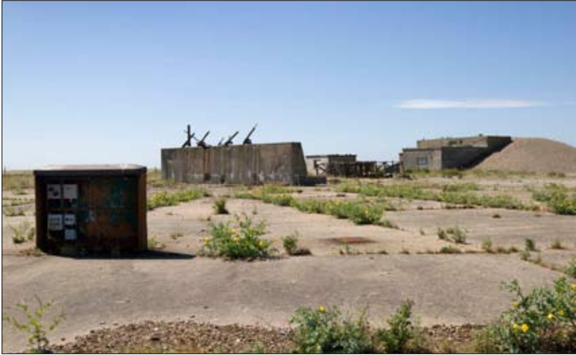
Figure 38: The Impact Facility F5, visible on the wall are the impact spots from firing bomb casings against its surface. To the right is the Control Room F4. (c) English Heritage DP068431
