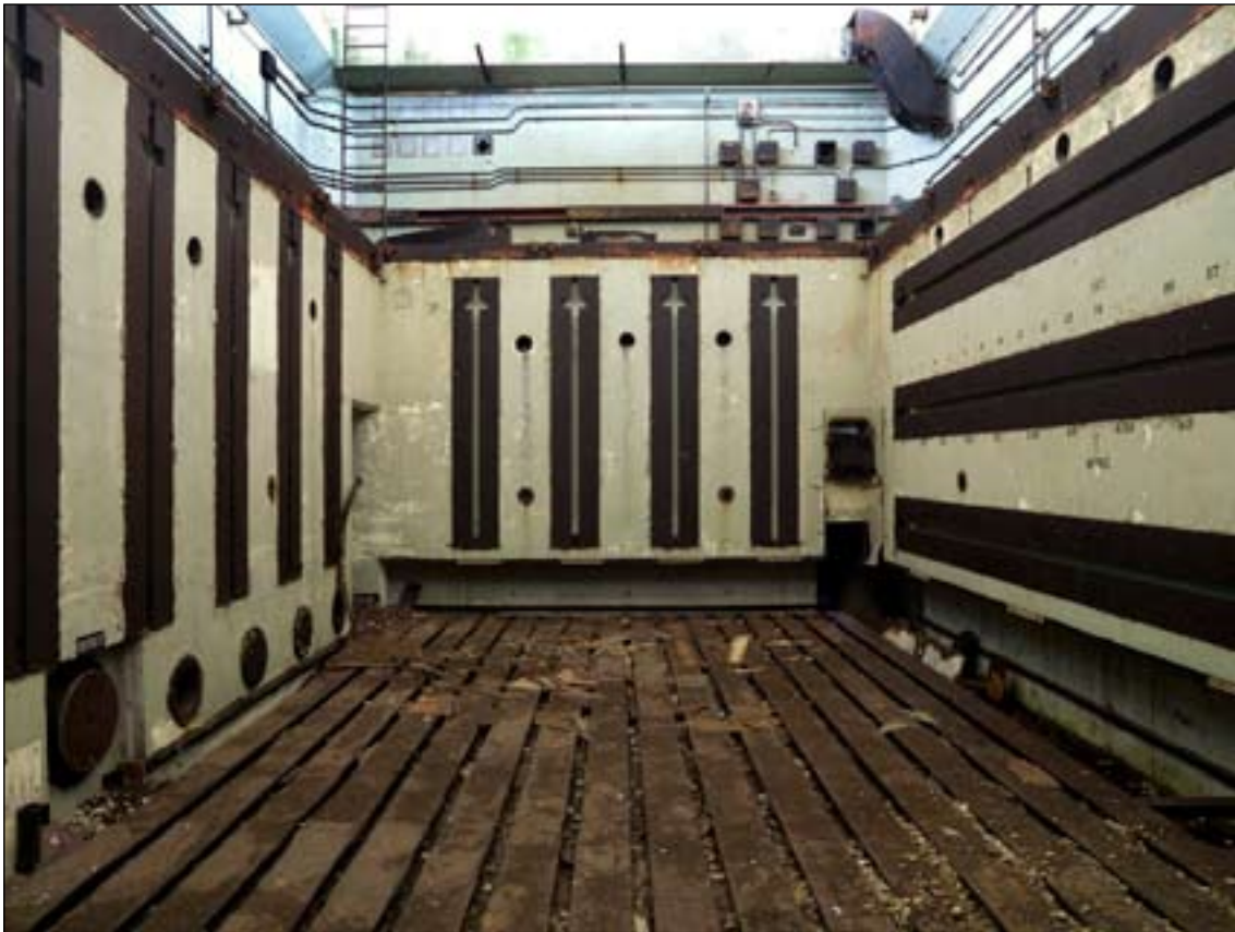
Figure 35: Vibration Laboratory E2 showing the main test chamber with slots for mounting test equipment. (c) English Heritage DP068518
