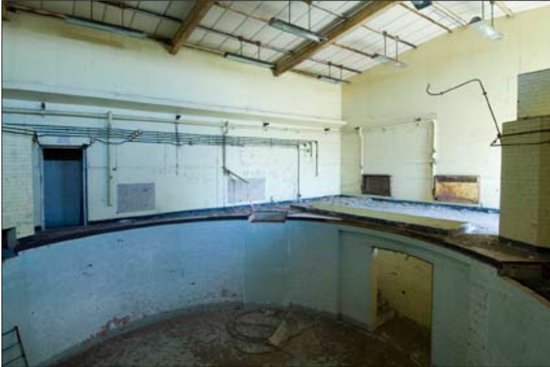
Figure 40: Centrifuge E1, interior showing the main entrance to the right and steps down into the pit. Also visible in this view are three of the four concrete piers that supported the centrifuge's frame. The rear door led to the emergency escape way. (c) English Heritage DP068497
