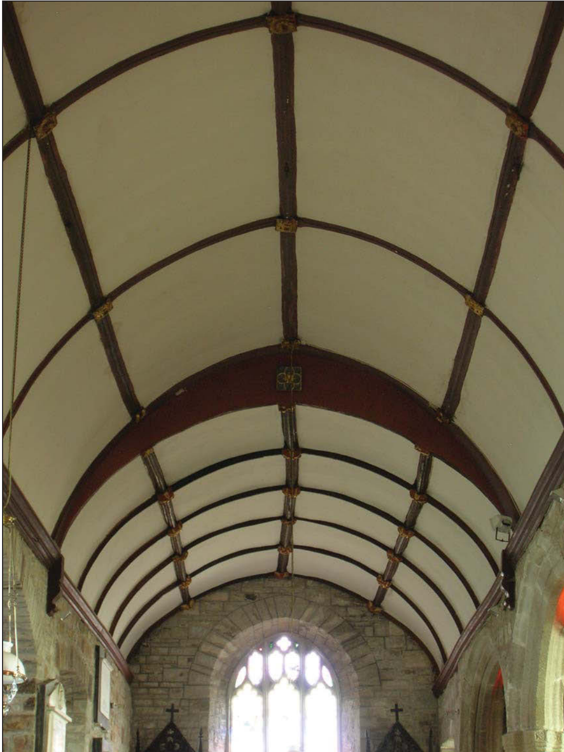
Figure 4: Nave and chancel ceiling (photograph taken facing east)
