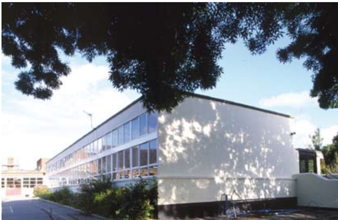
Fig. 23: Sidlesham, West Sussex (C.G. Stillman, 1936), one of the first schools to utilise 'light and dry' construction (© Elain Harwood).
