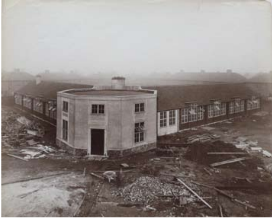
Fig. 22: Infants' Department of Athelney Road School, LB Lewisham (LCCAD, 1920-23) nearing completion. The octagonal hall is of rendered brick, and the flanking classroom wings are timber-framed (LMA:SC/PHL/02/0233-11; City of London, London Metropolitan Archives).
