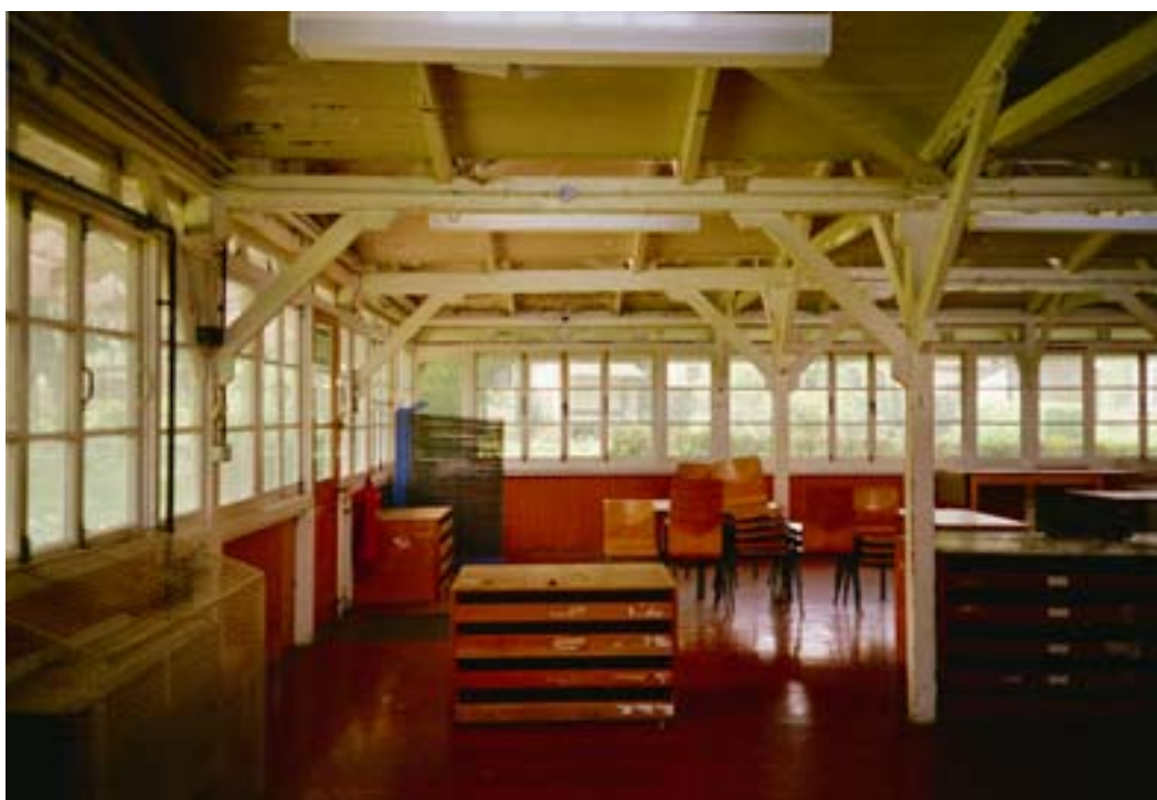
Fig 70: Interior of pavilion classroom at Aspen House (DP070356).
