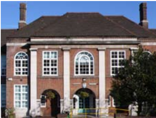
Fig 27: Entrance portico to the Woolwich County Secondary School, LB Greenwich (1927, LCCAD). DP070346.
