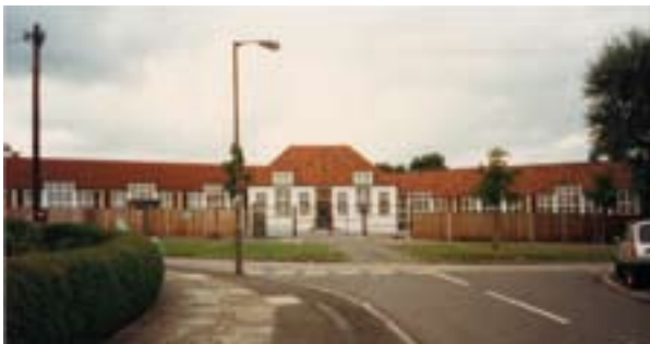
Fig. 42: The Juniors' and Infants' Department of Huntingfield Road, LB Wandsworth (LCCAD, 1920-25; dem.). A single-storey, pavilion-plan school, for the LCC Roehampton estate and designed by J.M. Scott (DP070359).
