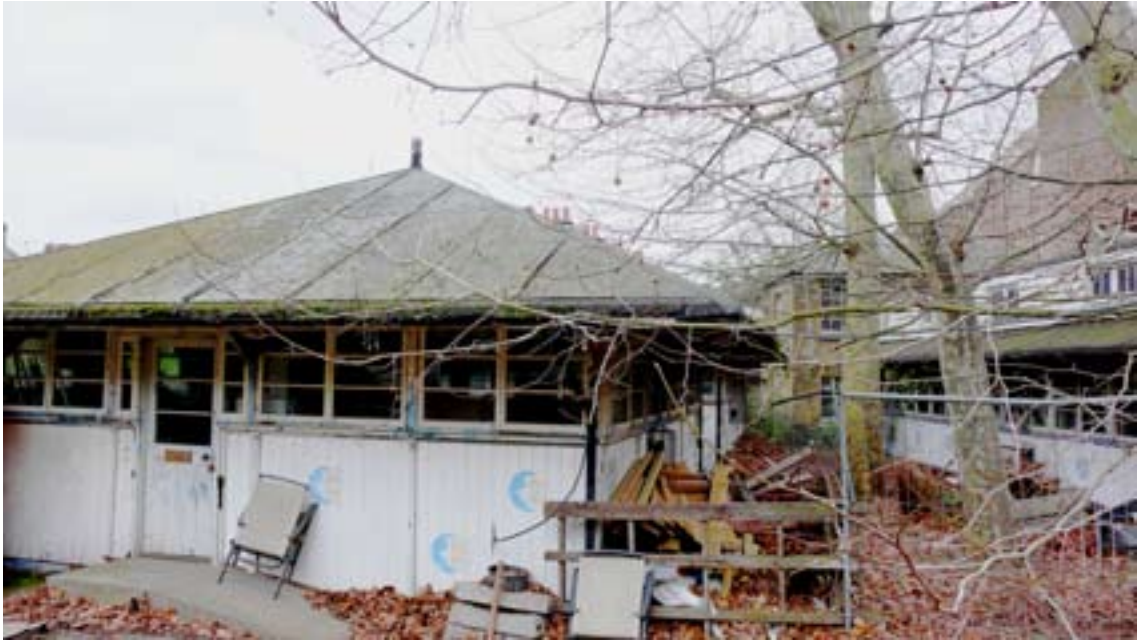
Fig 71: The buildings of the Geere House Open-Air school in 2009. The classroom pavilions are to the left and part of the dining/rest shelter can be made out at the right (DP070357).
