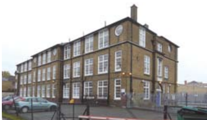
Fig 51: Webb Street School , LB Southwark . ( LCCAD , 1922). (DP070351).
