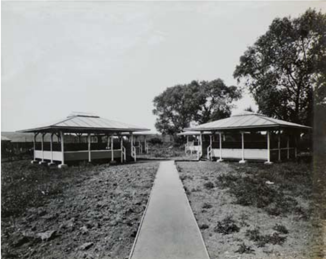
Fig. 14: The classroom pavilions at Wood Lane Open-air School, LB Hammersmith and Fulham. (LMA: SC/PHL/02/0432-5; City of London, London Metropolitan Archives).
