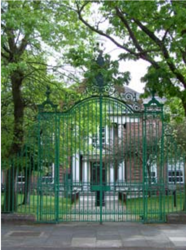
Fig 26: Entrance gates to the Roan School, LB Greenwich (Fletcher & Dannatt, 1926-28). DP070345.
