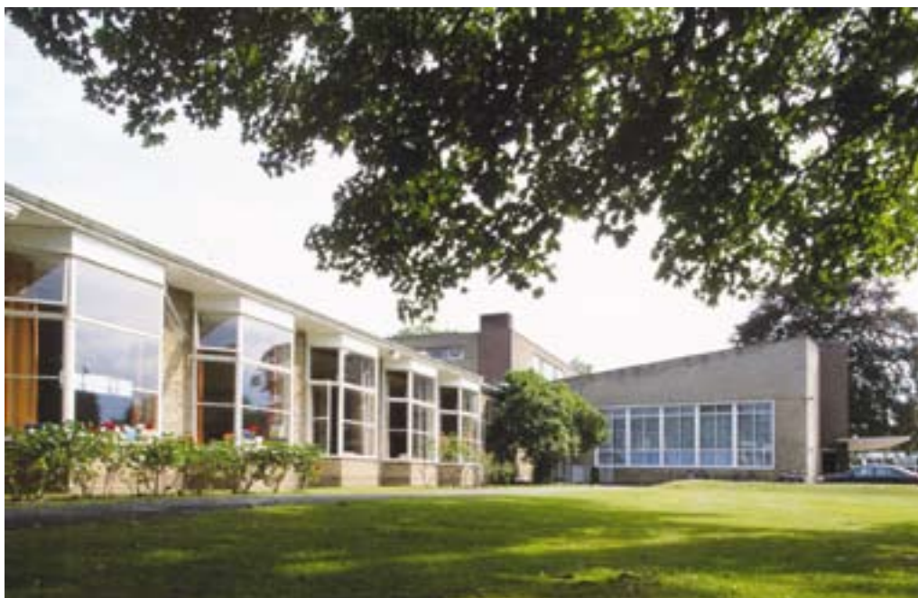
Fig. 7: Impington Village College, Cambridgeshire; Gropius and Fry, 1938-40. A view showing the adult education wing with assembly hall in the background (© Elaine Harwood).
