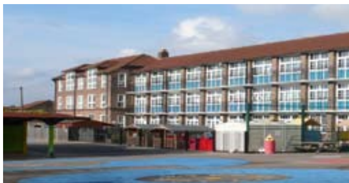
Fig. 1: Ealdham Square School, LB Greenwich (LCCAD, 1929). The school as built (top) and in 2008 with upVC replacement windows and other alterations. Top: LMA: SC/PHL/02/0240-39; City of London, London Metropolitan Archives. Bottom: DP070342.
