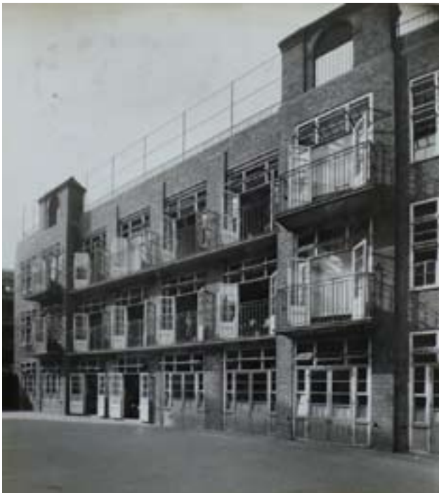
Fig. 17: Wilmot Street School, LB Tower Hamlets (LCCAD; 1931). (LMA: uncatalogued album entitled 'LCC schools section photographs'; City of London, London Metropolitan Archives).
