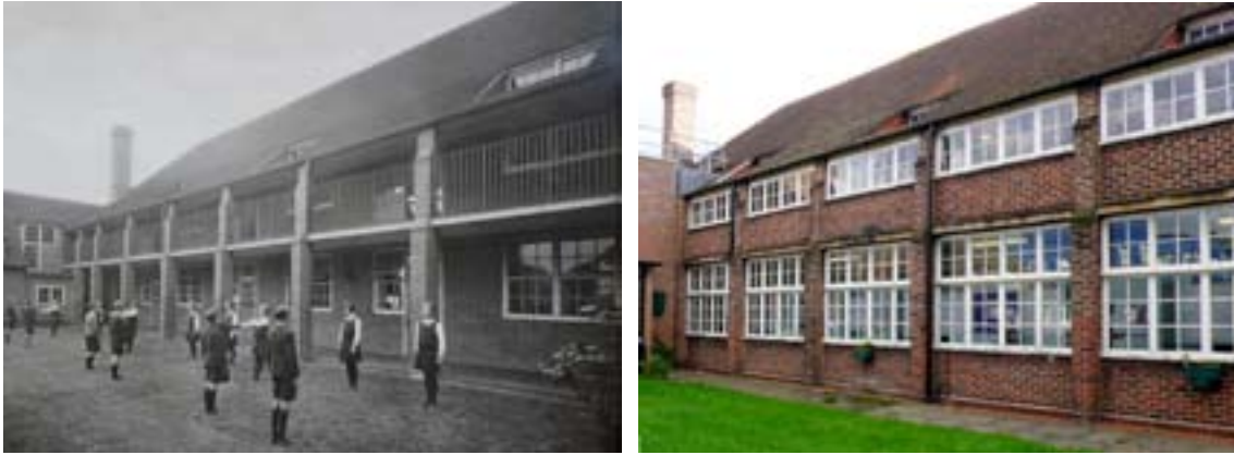
Fig. 55: North Hammersmith Central School, , LB Hammersmith and Fulham (LCCAD; 1931). The 'veranda' corridors, shown in this 1932 photograph (left), had been infilled by 1937 (right). (Left: LMA: SC/PHL/02/0267-21; City of London, London Metropolitan Archives. Right: DP070353).
