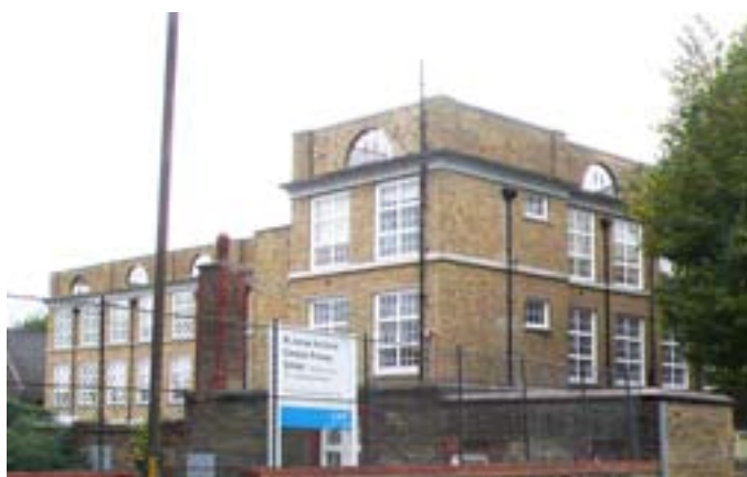
Fig 50: Sumner Road School , LB Southwark . ( LCCAD , 1921-22). (DP070350).
