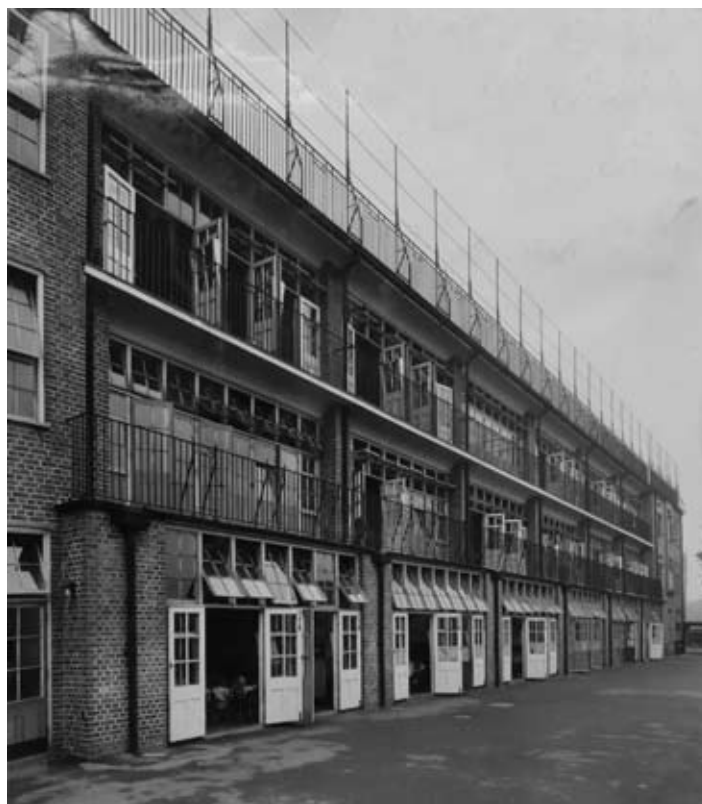
Fig 54: South elevation of Hanover Street School, LB Islington, (LCCAD, 1931-32), overlooking the Regent's Canal. (LMA:SCI/PHL10210243-6; City of London, London Metropolitan Archives).
