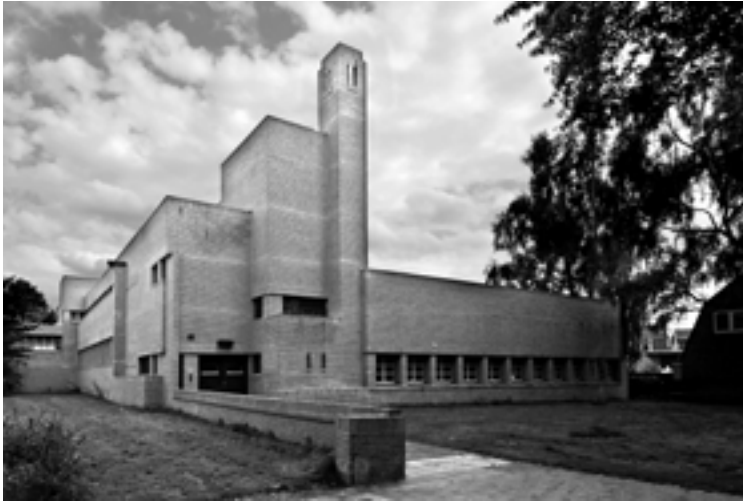
Fig 28: Bavinck School, Hilversum (W.M. Dudok, 1921-22). (Reproduced courtesy of Roosje Hoogenhout; Copyright acknowledged).
