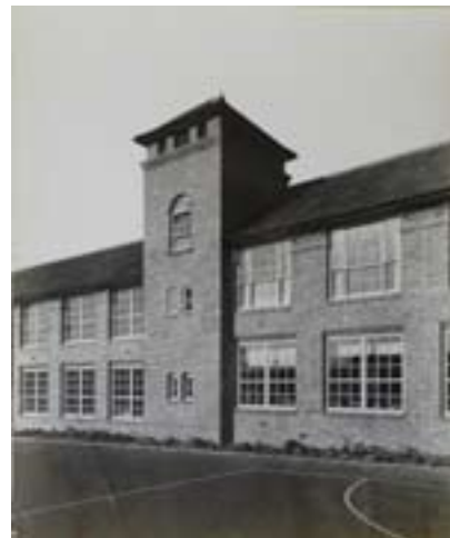
Fig. 45: Detail of south elevation of the King's Park School, LB Greenwich (LCCAD, 1934). The tower separates girl' and boys' classrooms wings (LMA: SC1PHL10210245-25; City of London, London Metropolitan Archives).
