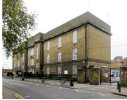
Fig. 41: North elevation of London Fields School, LB Hackney (LCCAD, 1921-23). A similar view was published in the LCC's The London Education Service , captioned 'A return to a simple style'. The stark corridor elevation, with its widely-spaced windows, was chosen over the more generous fenestration of the classroom elevations. (DP070347).
