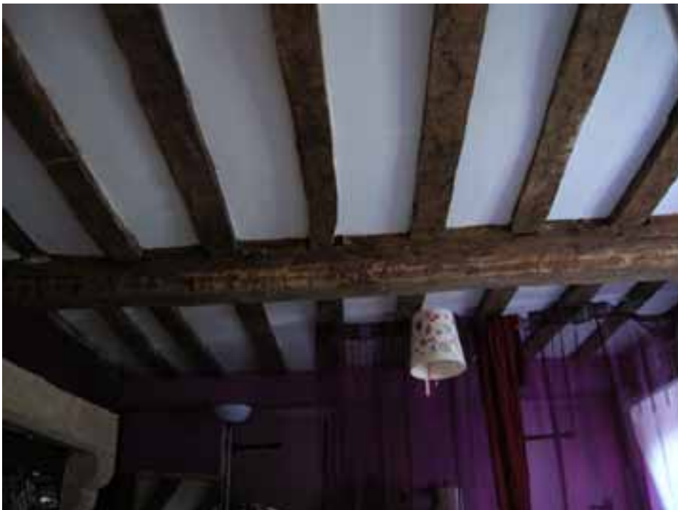
Figure 4 (top): Ceiling to bedroom 2 (now the office) of No 1 The Square
