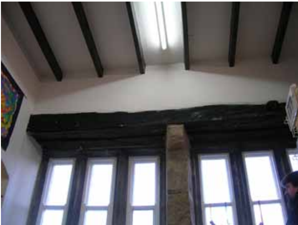
Figure 6 (top): Ground-floor ceiling (living room) room of No 1 The Square
