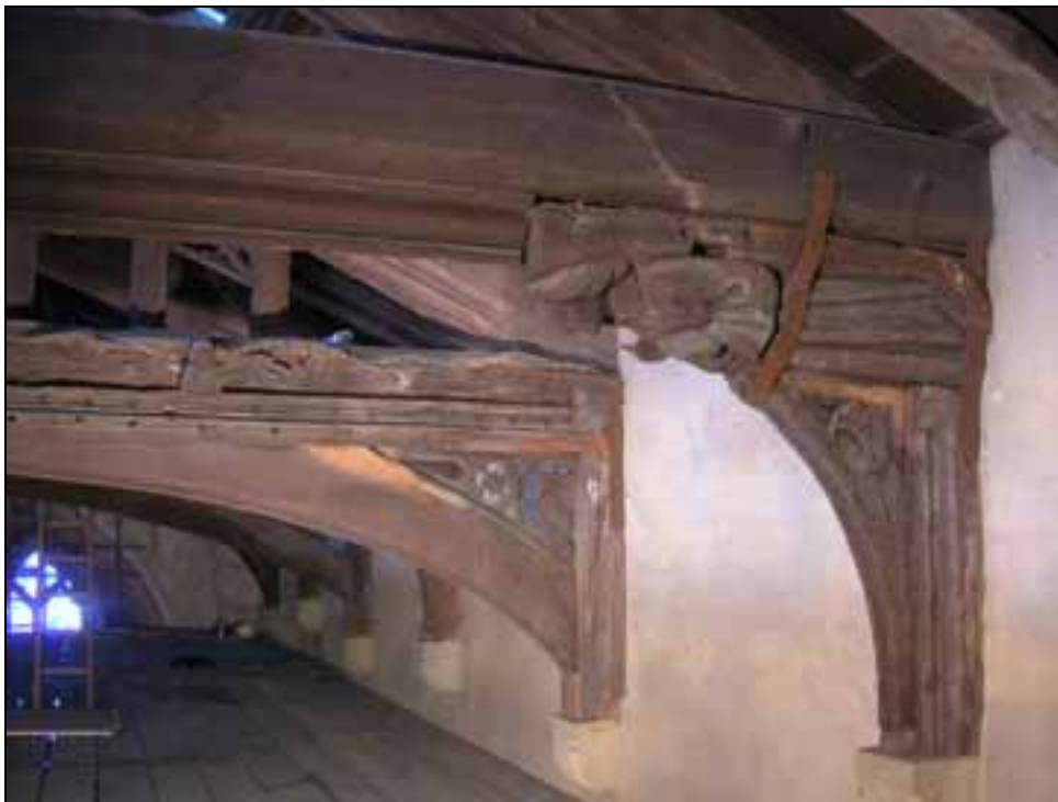
Figure 5: Nave roof; intermediary truss 6
