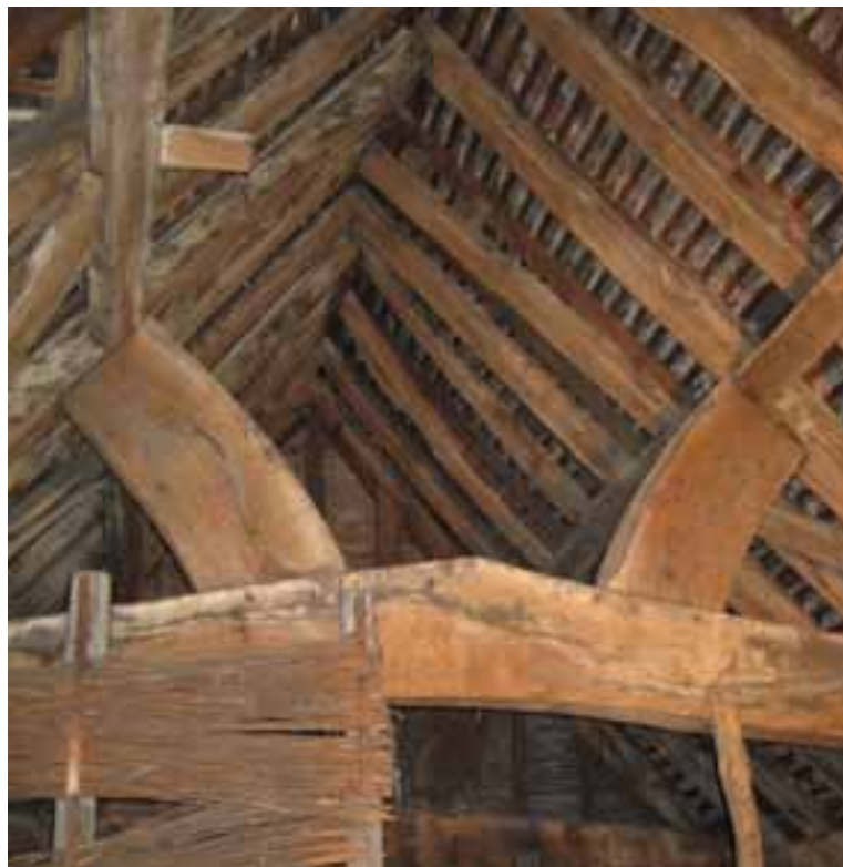
Figure 8: South cross-wing truss 2 looking south-east
