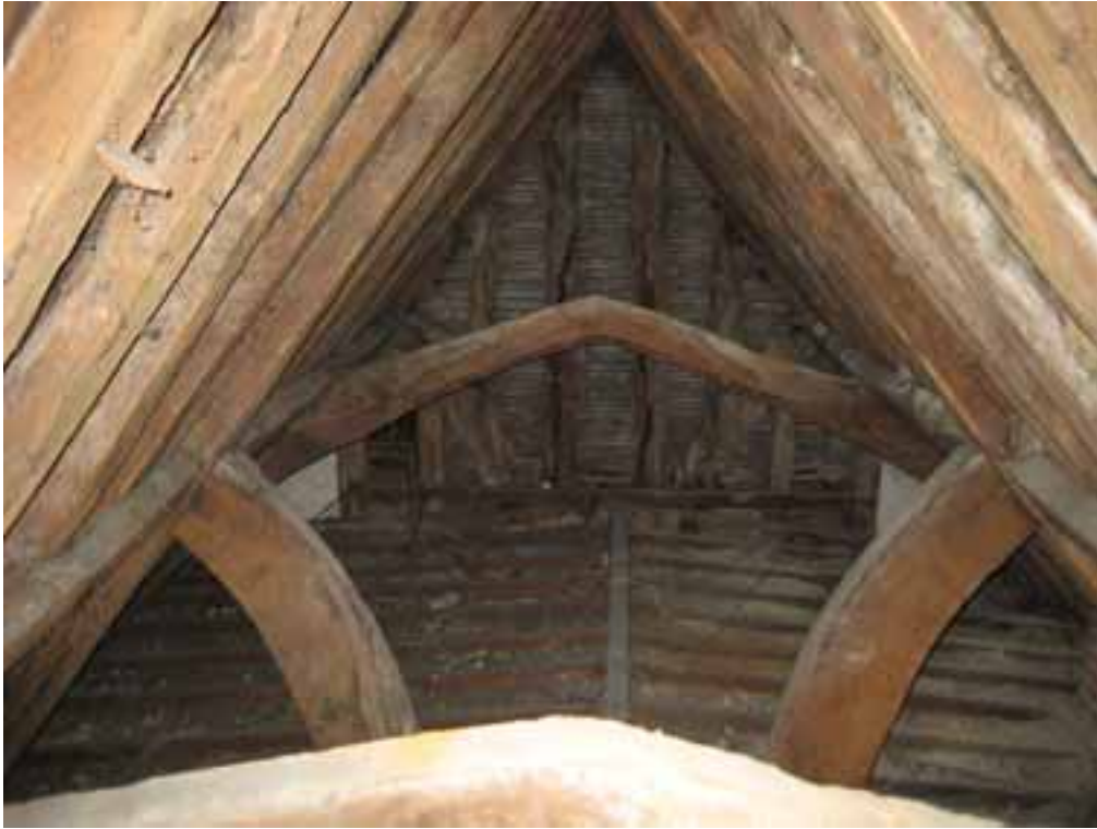
Figure 7: North cross-wing truss 7 viewed looking west
