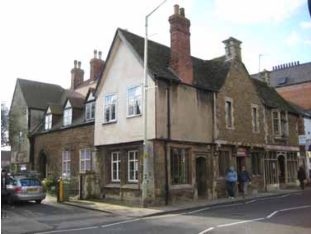
Figure 3: Flore's House looking south west
