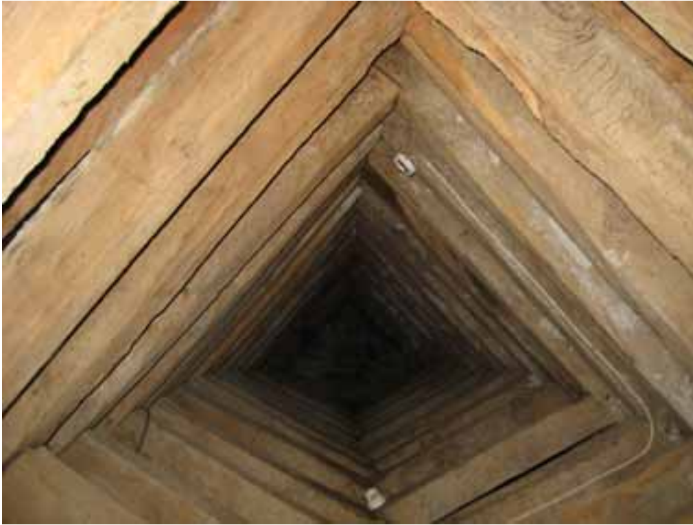
Figure 7: Roof timbers over the Great Chamber viewed looking south-east
