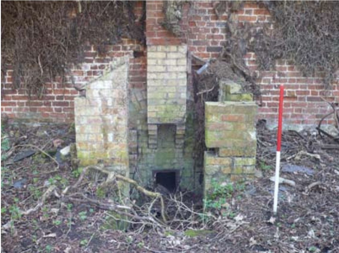
Plate 9: Brick-built furnace attached to the external face of the garden wall close to its midpoint. This probably provided heat for a series of hot- and greenhouses placed along the interior face of the walled garden © David McOmish
