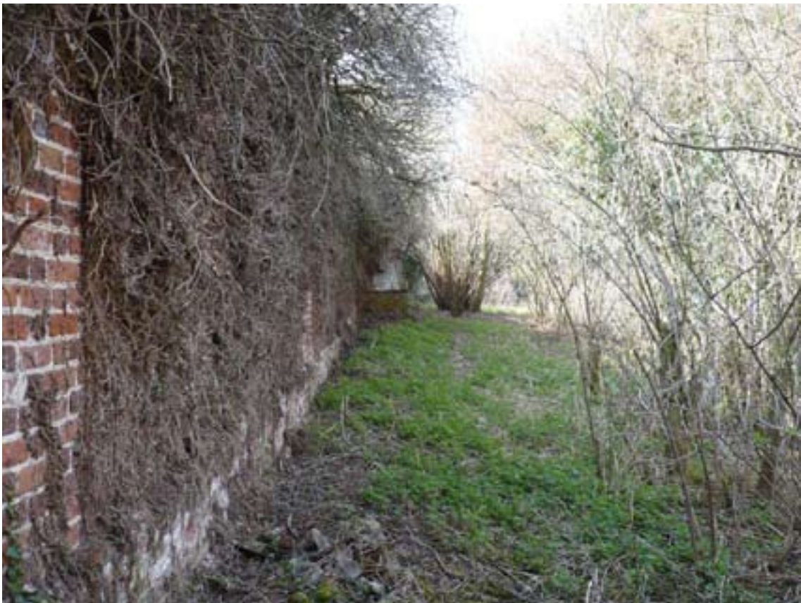
Plate 8: View of the garden wall and brick rubble (foreground) looking west from the south east corner of the moated enclosure. The wall rests of a wider plinth and there are suggestions of later modifications and episodes of re-building © David McOmish
