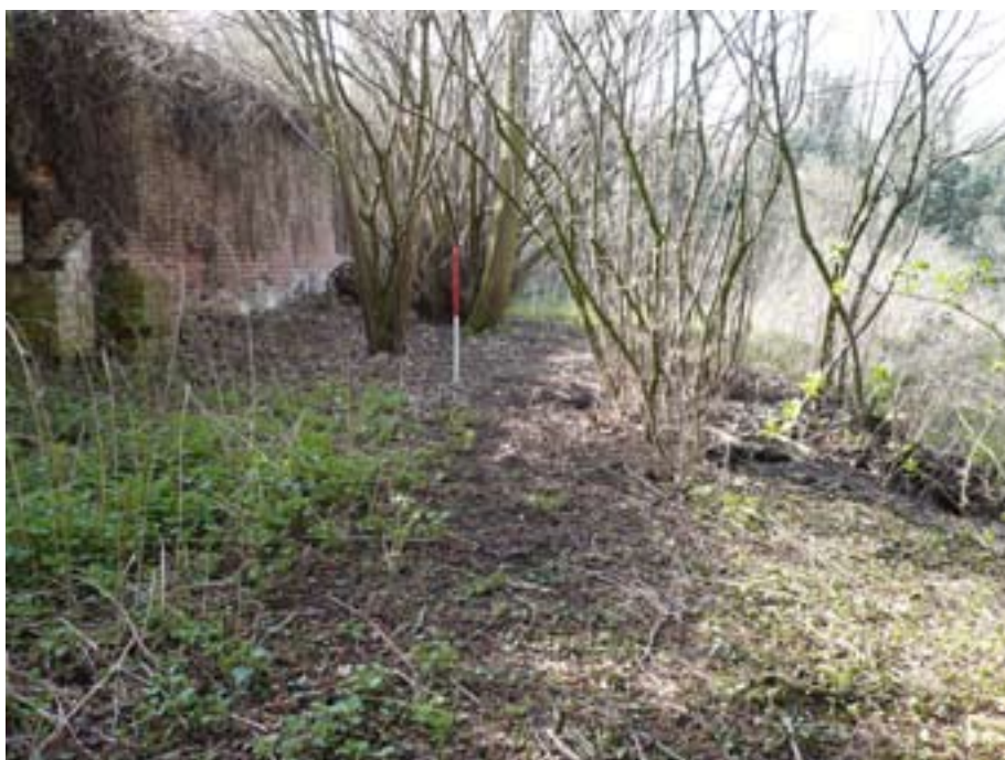
Plate 10: A talus-like deposit of coal, ash, and slate spread from the furnace towards the edge of the moat ditch, obscuring the counterscarp bank and walkway here © David McOmish
