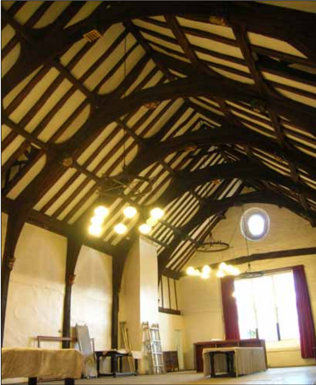
Figure 5: View of the first-floor hall (looking west to east)
