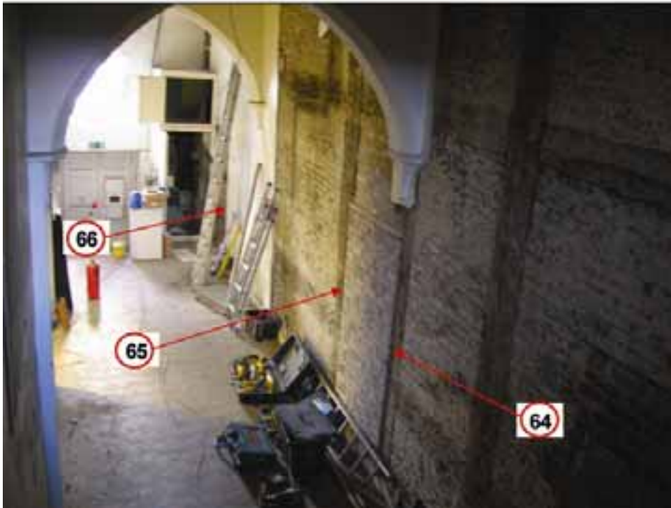
Figure 6j/k: East wall of the chapel to show sampled timbers
