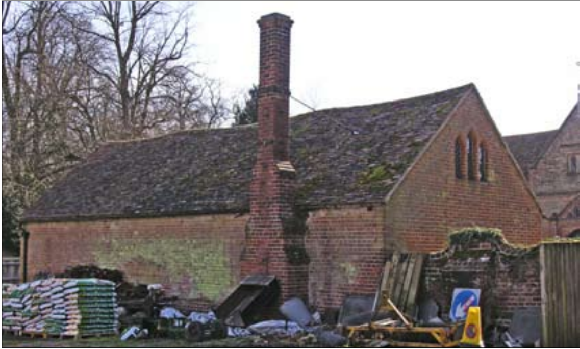
Fig. 3. The north and west fronts of the New Coach House showing the external brick chimney stack to the former forge.
