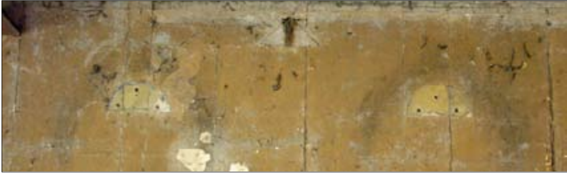
Fig. 9. The scars for fittings to support saddles in the Tack Room.
