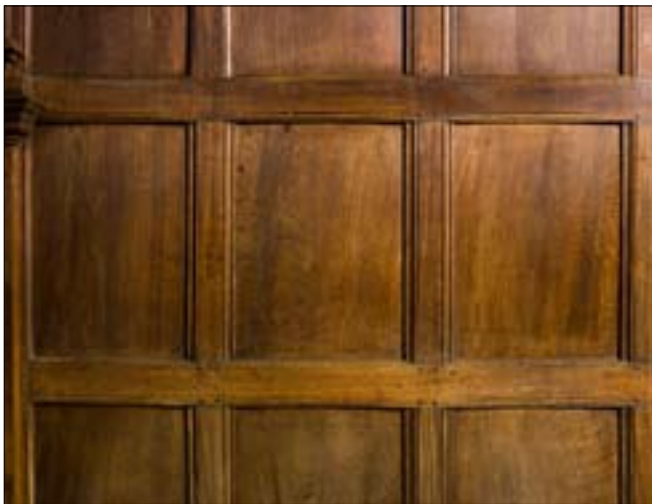
Figure 12. Typical section of panelling, with double-pegged joints and the two types of moulding. © English Heritage DP029562
