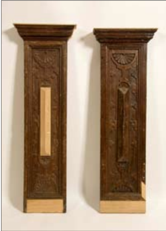
Figure 17. Front view of the two types of pedestal. The first type, to the left, is framed, while the second type to the right is of solid construction. © English Heritage DPO29372
