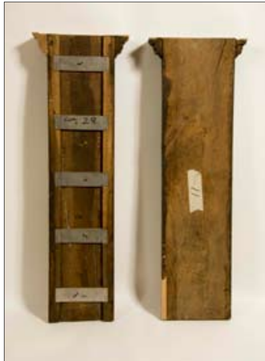
Figure 20. Rear view of the two pedestal types, showing framed and solid construction. © English Heritage DPO29373
