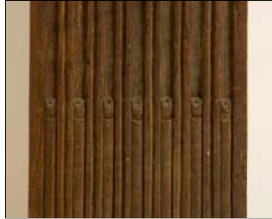
Figure 23. Type 2 pilaster with 'C' shape at the top of the cabling. © English Heritage DPO29369
