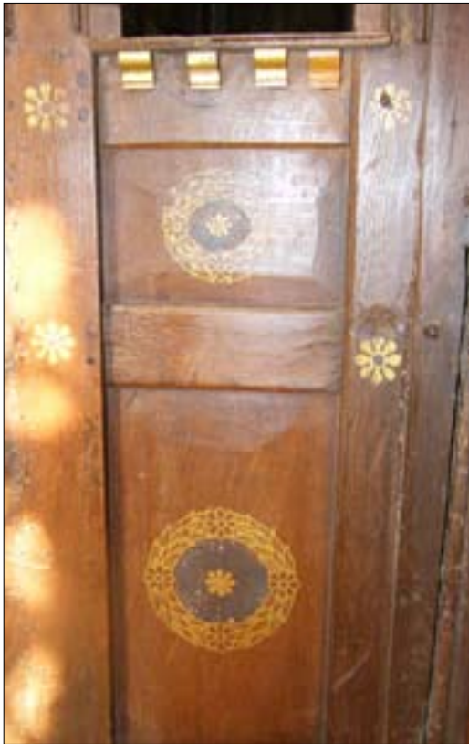
Figure 53. Rycote Chapel, c.1620, with original stencilled paint designs to frame and panel bed, but the remainder of the oak left exposed. © Nick Hill 2008
