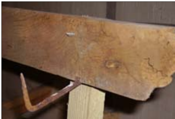
Figure 35. Original iron cramp used to fix panelling around WE2.07. © Nick Hill 2006
