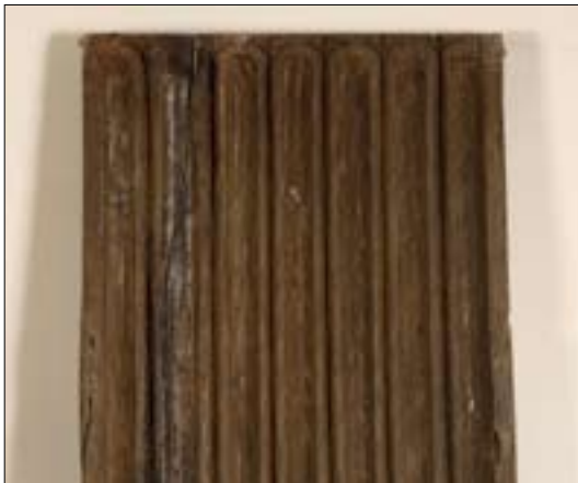
Figure 24. Top of Type 1 pilaster, with plain top to fluting. © English Heritage DPO29367
