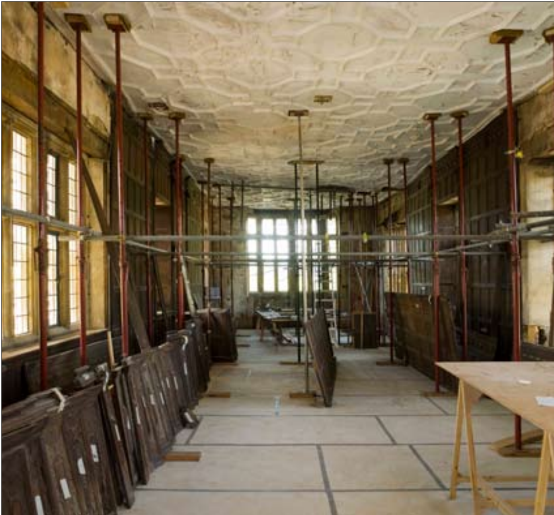
Figure 1. The Long Gallery during repair works in 2006.
