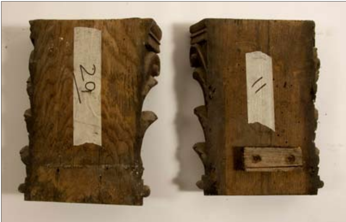
Figure 29. Rear face of capitals. The right hand one is made of two pieces, with a vertical glued joint, later reinforced with a screwed-on batten.
