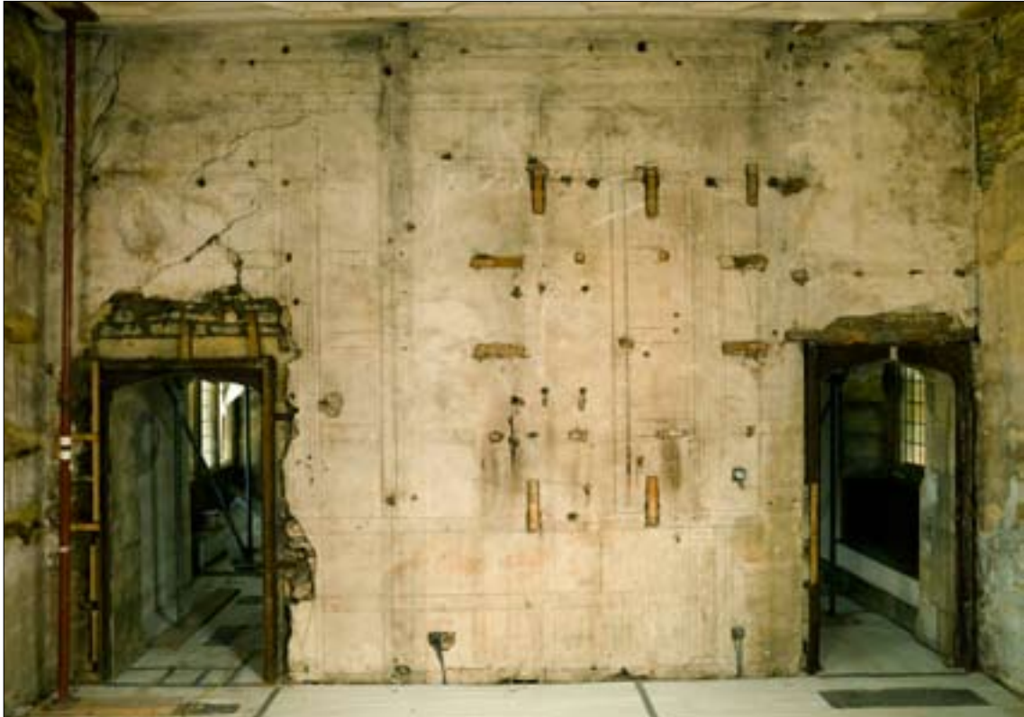
Figure 45. The design on the south wall after removal of panelling.
