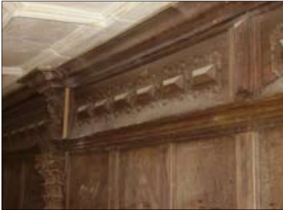
Figure 14. The frieze and cornice in 2006 before dismantling. © Nick Hill 2006
