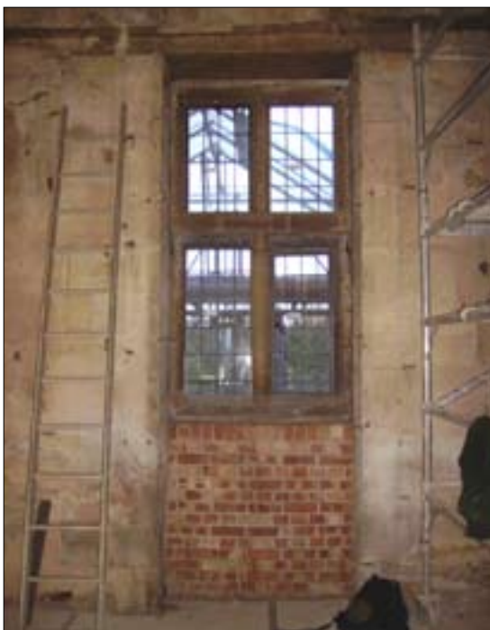
Figure 32. The original doorway onto the east balcony, converted to a window in the early 20 th century. © Nick Hill 2006
