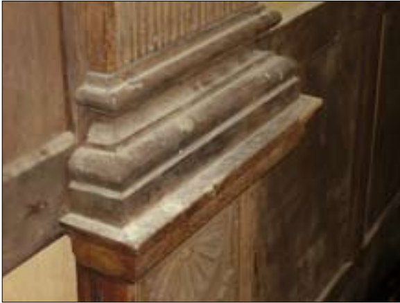
Figure 26. Moulded base to pilaster. © Nick Hill 2006
