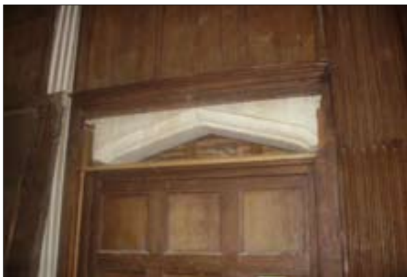
Figure 33. North-west doorway, with original stone doorway covered by the panelling – clearly added later. © Nick Hill 2007
