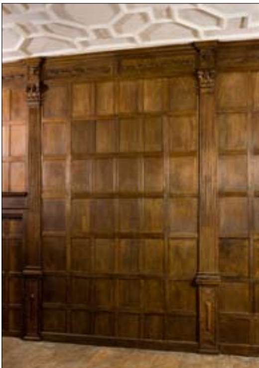
Figure 3. Typical section beside the north-west doorway in 2008.
