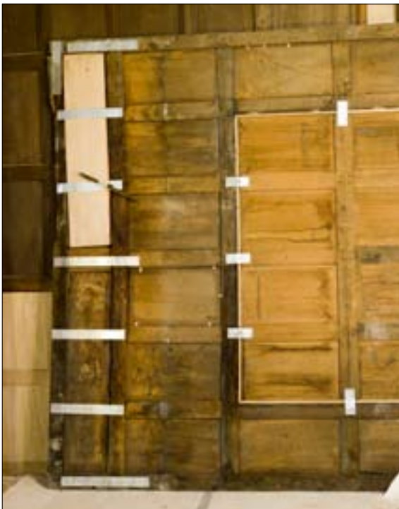
Figure 7. Detail of rear of panelling. © English Heritage DPO29338
