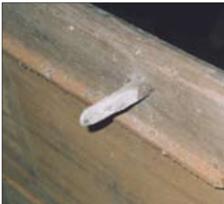
Figure 34. Original oak peg used to fix the panelling. © Nick Hill 2006
