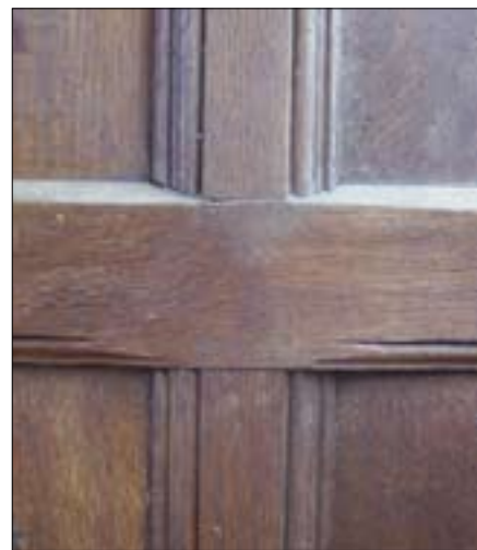
Figure 13. Detail of the two moulding profiles, with run-out stops not mitred joints. © Nick Hill 2007
