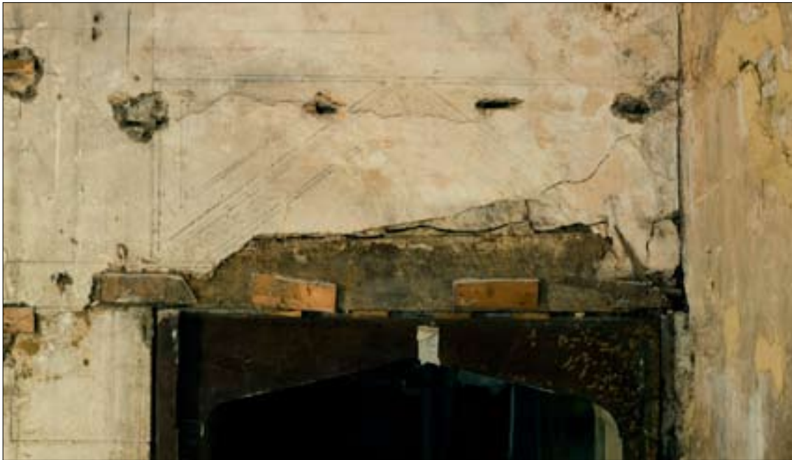
Figure 48. Pediment over doorway with guilloche detail.
