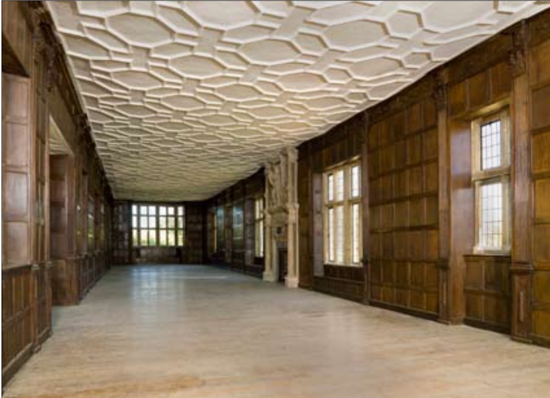
Figure 2. The Long Gallery at the completion of repairs works in 2008.
