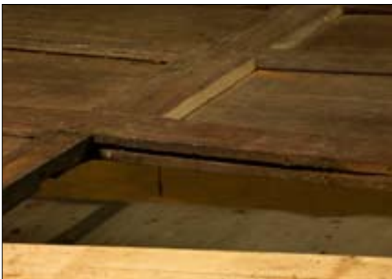
Figure 16. Panelling from bay window WE2.16. The run-out formation of the groove shows that a plough plane was used.
