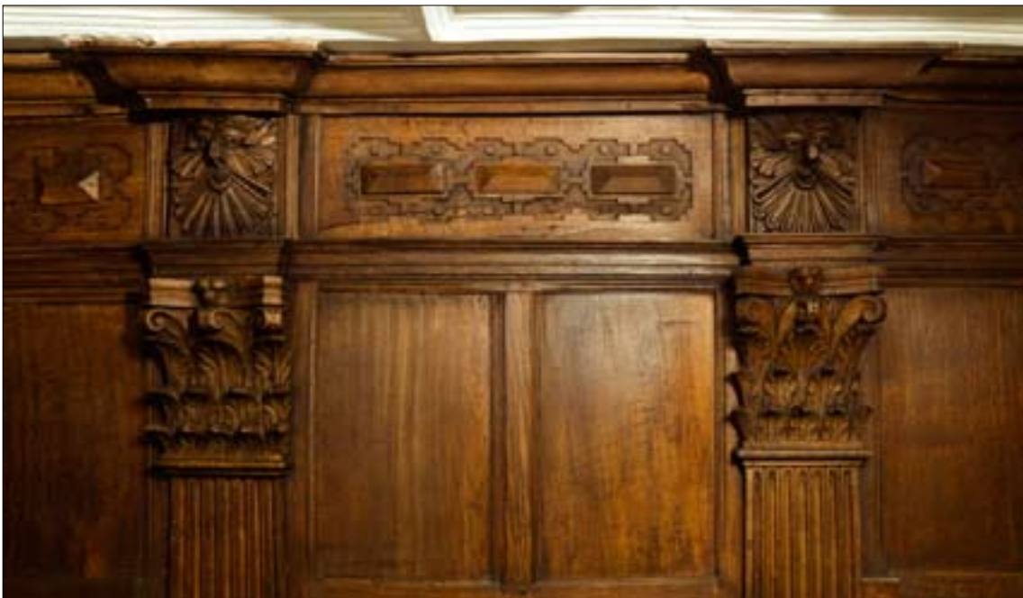
Figure 15. Upper part of the panelling in 2008, after repairs. © English Heritage DPO29546
