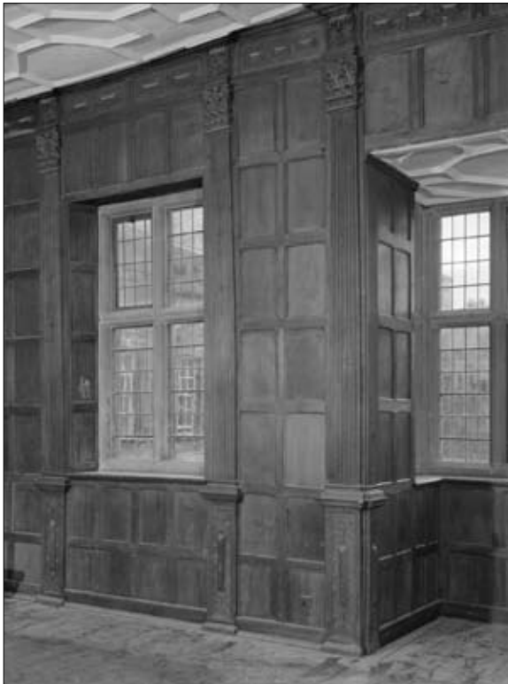
Figure 5. Section of panelling beside western bay window in 1978. © NMR BB78 8598
