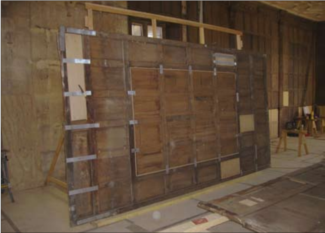
Figure 6. De-mounted section of panelling showing the blocking to portrait opening.
