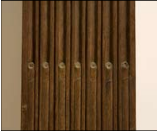
Figure 22. Type 1 pilaster with 'S' shape at the top of the cabling to the fluting. © English Heritage DPO29370
