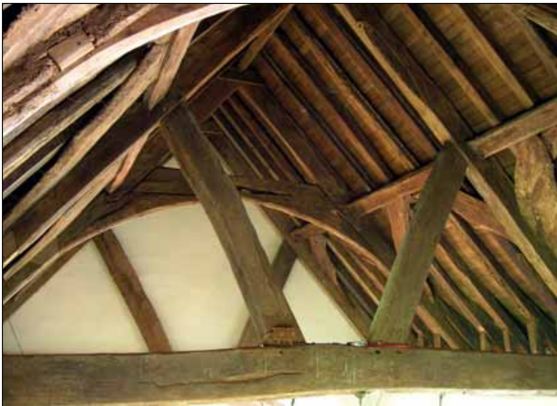
Figure 4: Nave roof, truss 3 in foreground (photograph taken from Truss 4)
