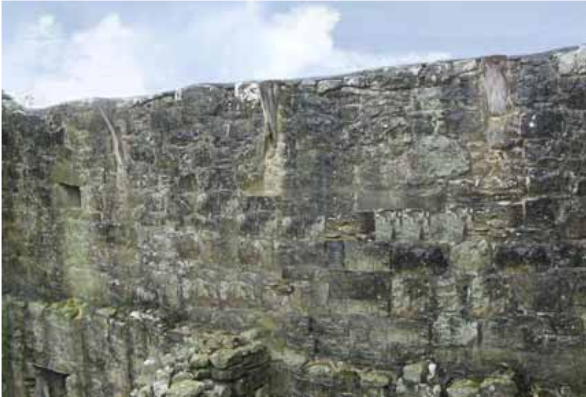
Figure 5: North wall, interior, to show stub remains of the three raised cruck blades
