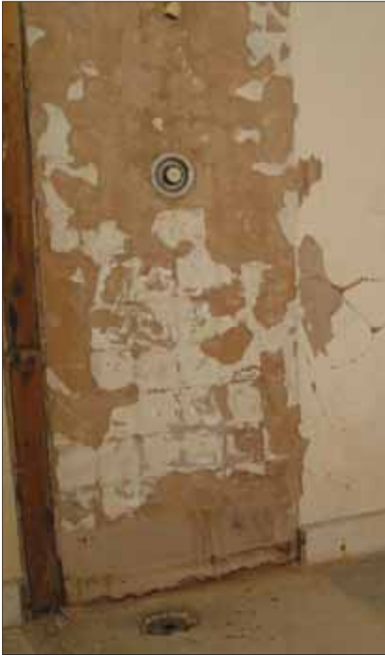
Fig. 10 Ablution Rooms (SI.03) showing the remains of shower cubicles.
