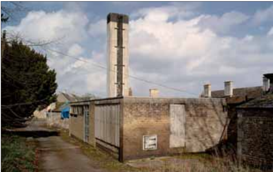
Fig. 5 The boiler house, from the south west.
