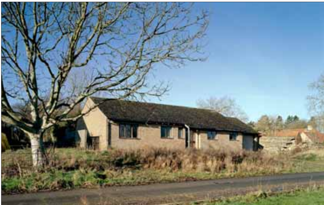
Fig. 19 Priest's Bungalow at north end of Hunting Way.
