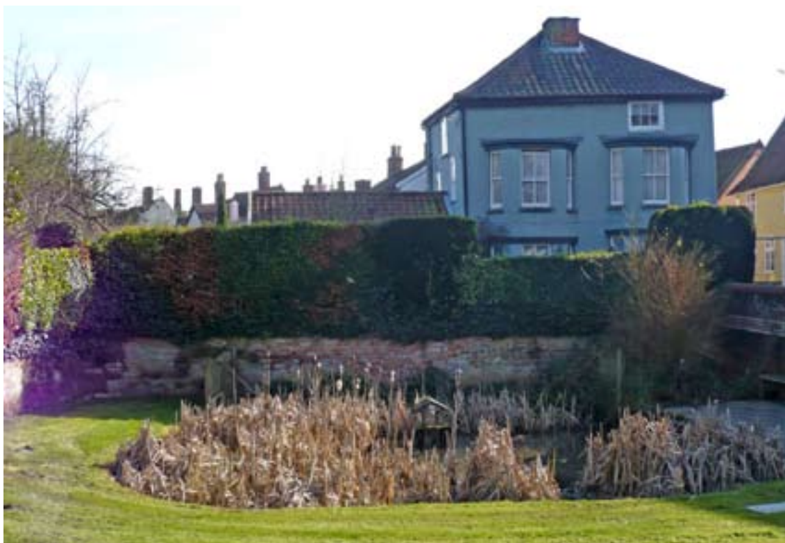
Figure 9 - Properties to the north of Castle Street. The pond in the foreground lies within the outer bailey ditch. The properties can clearly be seen to have encroached on this and the building in the foreground has settled into the softer make-up deposits in the ditch. From TM 2862 6357 looking east.
