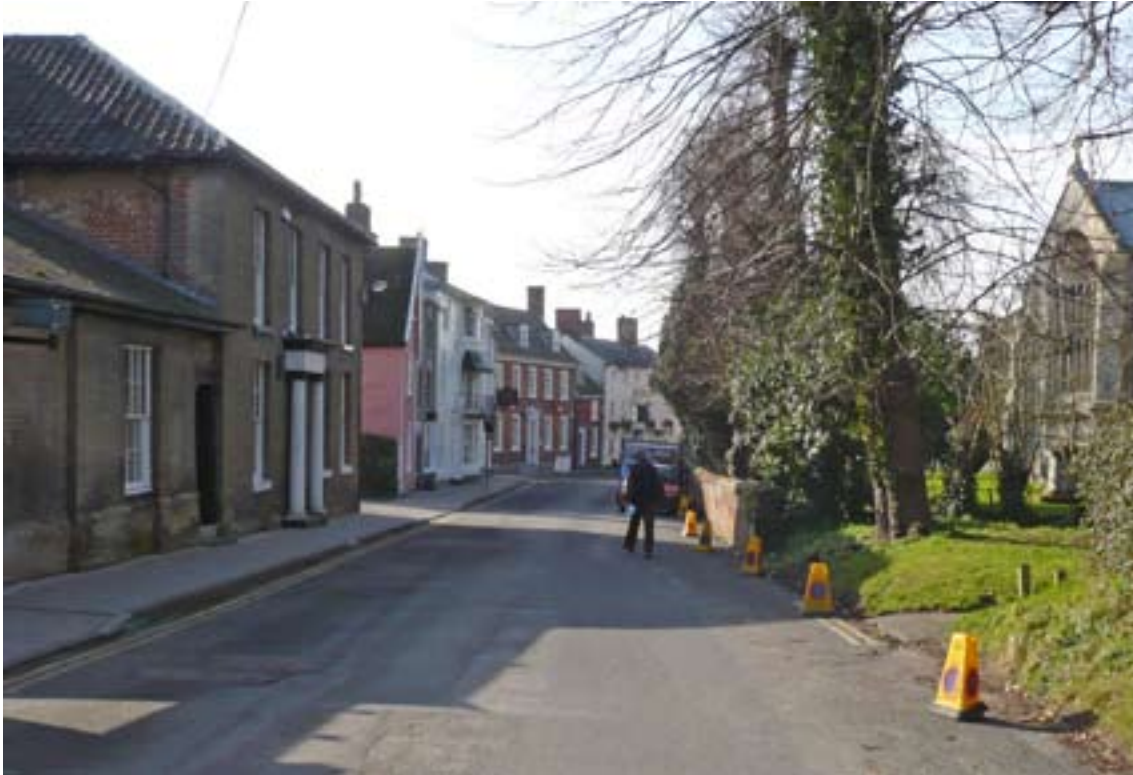
Figure 8 - Church Street. The change in orientation where Double Street meets Church Street is clearly visible. St Michael's Church is on the right. From TM 2861 6355 looking SW.
