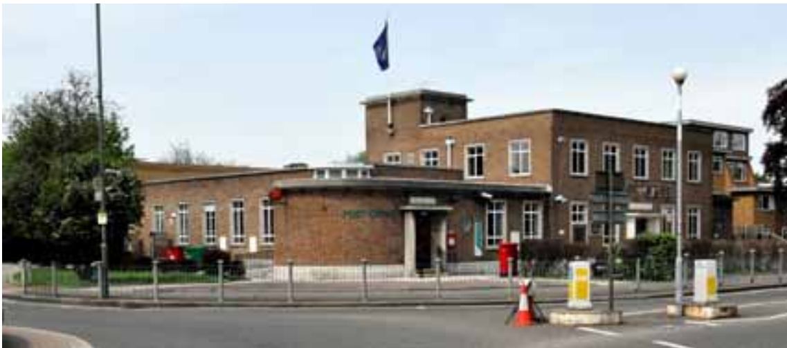
Figure 13 Beckenham Post Office and Sorting Office (1939) by F.A. Llewellyn (DP040073).
