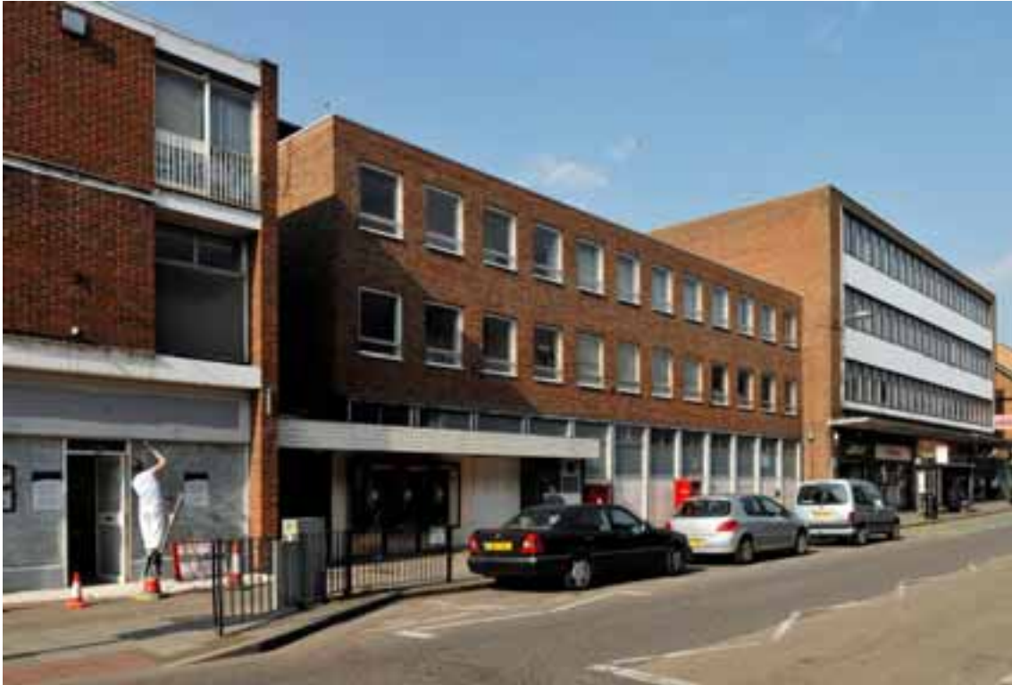
Figure 14 Hitchin Head Post Office – the first Post Office to emanate from the cross-departmental R&D group established in 1957 which was tasked with providing more economical, efficient buildings (DP040074).
