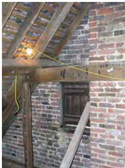
Fig. 45: Detail of south truss of hall range. Fair face outwards, indicating a terminal truss. The purlin extends beyond the principal rafter and there are no signs that the truss was ever closed. The stack is visible to the right (DP040099).
