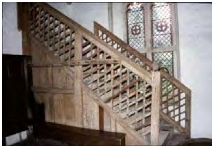
Fig. 59: Lattice balustrades to stair at the Hospital of St Cross, Winchester (© Linda Hall).
