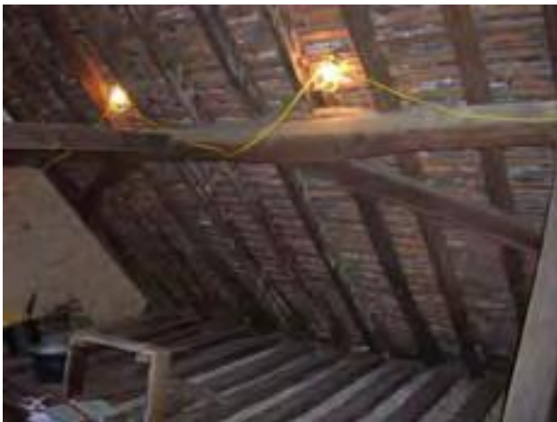
Fig. 36: Detail of principal truss, showing clasped purlin construction and windbrace (DP040095).
