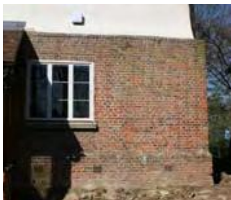
Fig. 8: The west wall of the parlour, showing diaperwork (DP040083).
