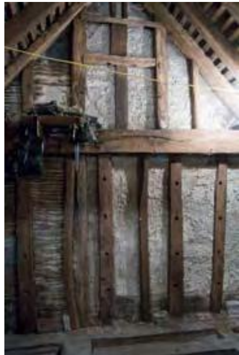
Fig. 37 (above): Western truss of cross wing. Note pegholes for fitting below collar, and former three-light window above. Photograph by Derek Kendall (DP042424).
