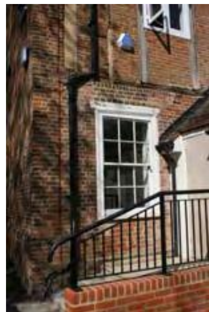
Fig. 11: Detail of east elevation, showing inserted sash window (DP040080).
