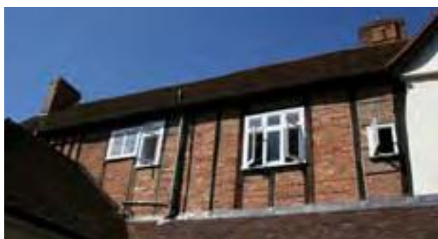
Fig. 12: First floor of east elevation (DP040081).
