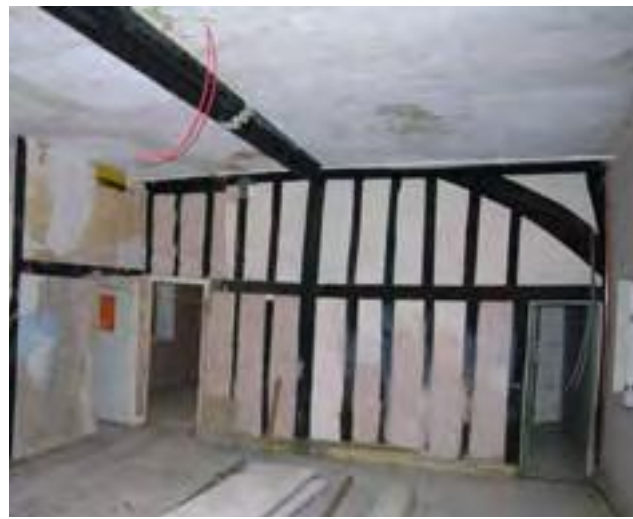
Fig. 29: Parlour chamber (room 28), looking southwest. Photograph by Derek Kendall (DP042356).
