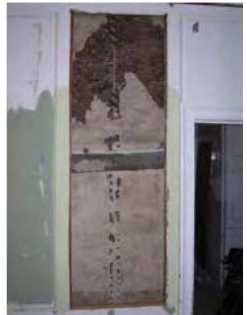
Fig. 47: South wall of entrance hall (room 9). Fragments of wallpaper of c.1700 survives under later panelling (DP040100).
