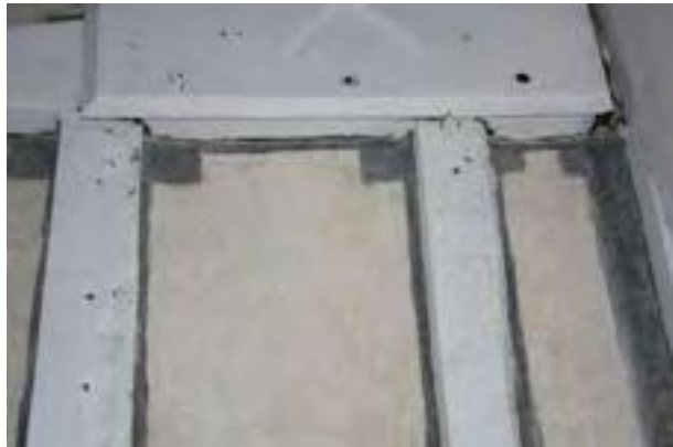
Fig. 60: Painted decorative scheme in the infill panels of the framing of the principal stair (DP070340).
