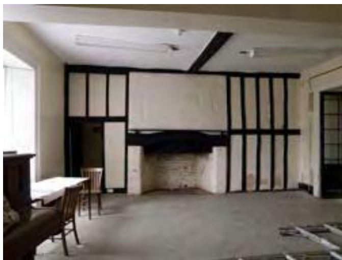
Fig. 16: North elevation of hall. Photograph by Derek Kendall (DP042331).
