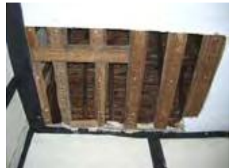
Fig. 43: Framed opening adjacent to north wall of room 25 (DP040098).
