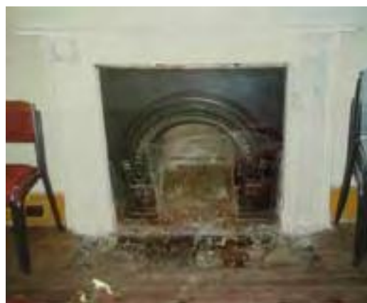
Fig. 22 Detail of Room 10 fireplace in the late 20 th century. (Local history room at Manor Farm Library, Ruislip).
