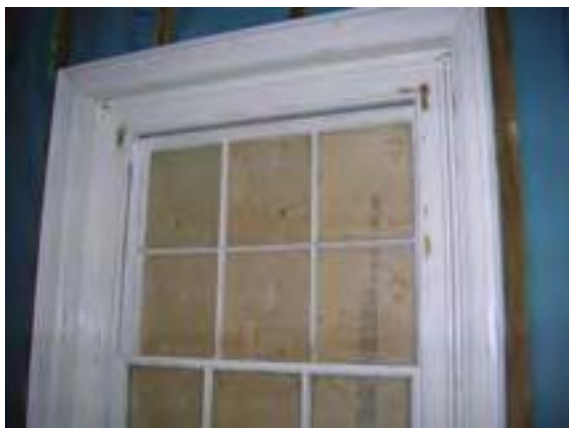
Fig. 53: West window of room 23, showing early 19 th century glazing bars within an 18 th century architrave (DP070336).
