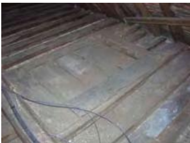
Fig. 34: Framed opening in attic floor (DP040094).
