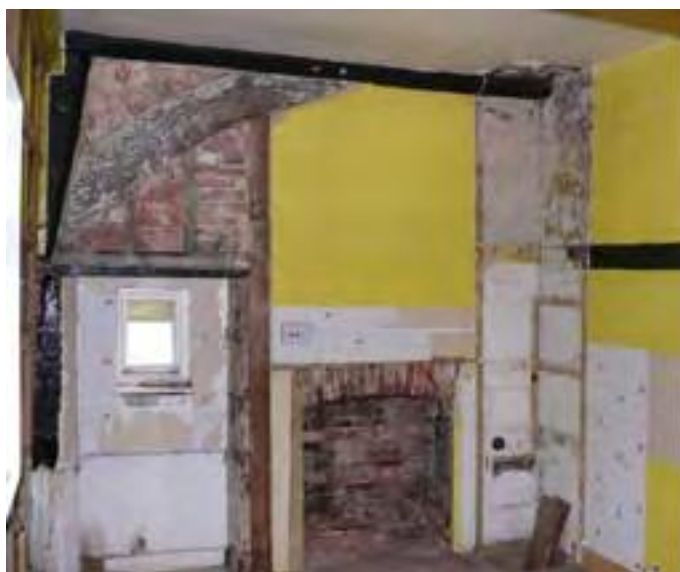
Fig. 27: Room 20, looking south (DP040088).
