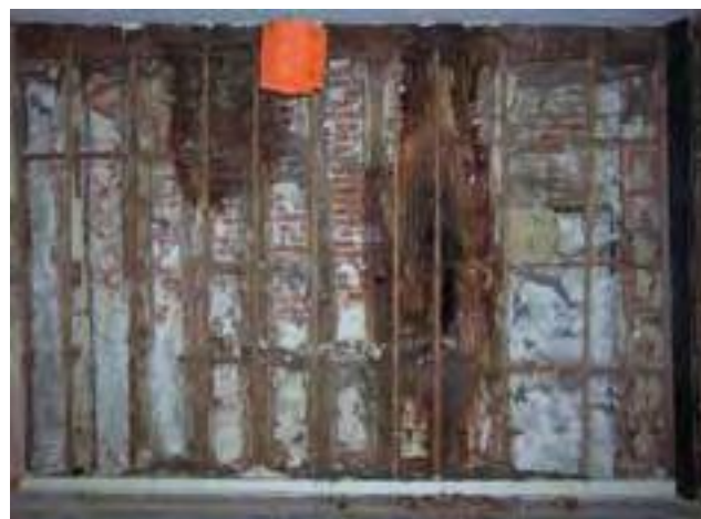
Fig. 31: North wall of Parlour chamber (Room 28), exposed during works in 2007-08. Note blocked garderobe door to right. (DP040090).
