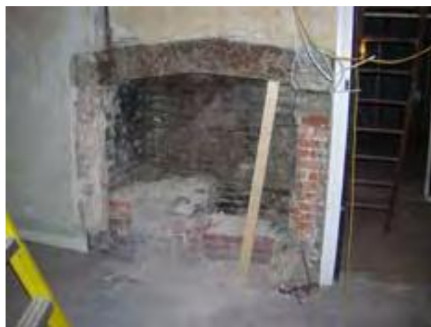
Fig. 26: Hall chamber fireplace, exposed during works in 2007-08 (DP040087).
