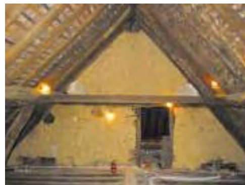
Fig. 39: Closed truss III of hall range (DP040096).
