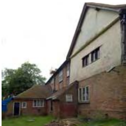
Fig. 14: East elevation of cross wing (DP040082).
