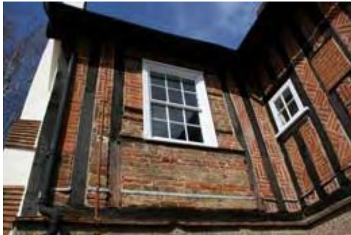
Fig. 15: South elevation of cross wing at first-floor level, showing replacement infill and window in position of the original window (DP040084).
