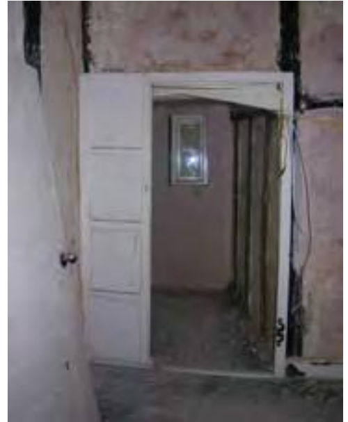
Fig. 33: Original, four-centred doorway to closet (room 26), reduced in size with reused 17th century door (temporarily removed) and panelling (DP040093).
