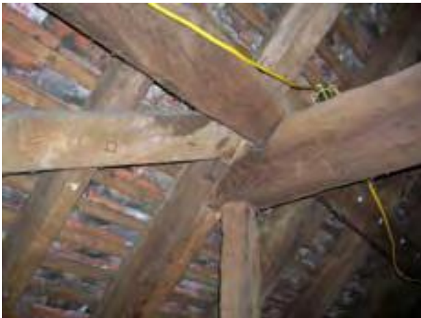
Fig. 36: Detail of principal truss, showing clasped purlin construction and windbrace (DP040095).
