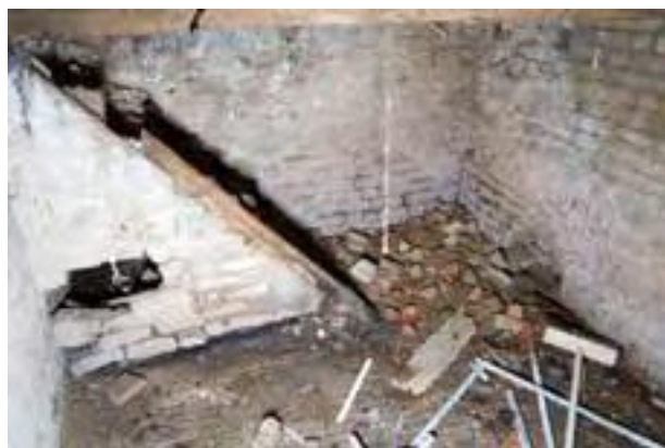
Fig. 25: Cellar underneath Room 14. Photograph by Derek Kendall (DP042412).
