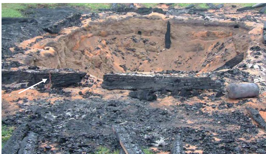
Figure 2. The Grubenhäus on 30 March 2005 looking east (Photo: Brian Kerr). Note the chain lying over the cill beam (arrowed) and the fire extinguisher (centre right).
