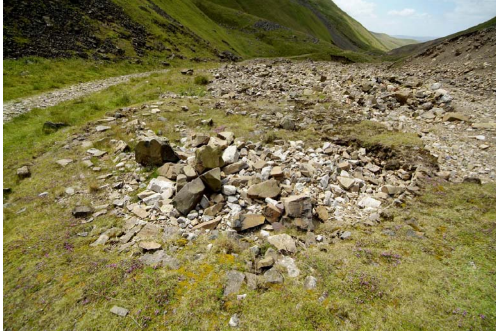
Figure 6 Remains of a buddle (75), the western edge of which is being eroded by Scordale Beck (right-hand side of the photograph). (Taken in July 2006)
