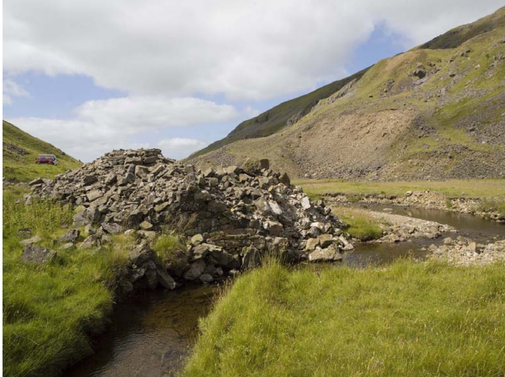
Figure 7 The remains of a dressing-mill (81) with a braid of Scordale Beck running up to and around it. (Taken in July 2006)
